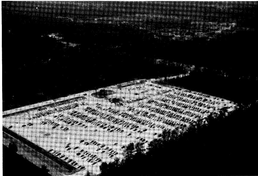
Figure 17. Aerial View of Spring Park-and-Ride Looking to the Northwest
