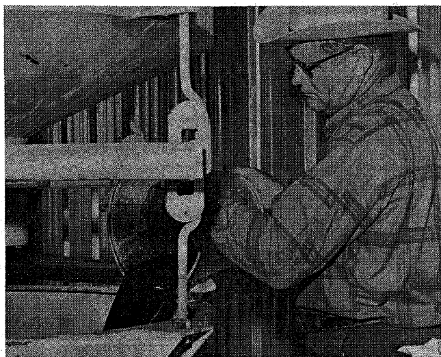
Figure 3. Adding admixtures to batch water.
