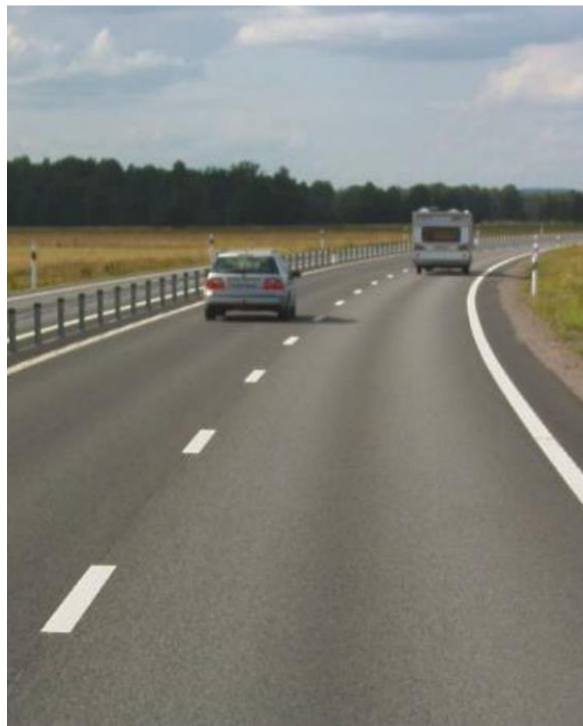
Figure 8. Passing Lane with a Median Barrier in Sweden (36)
