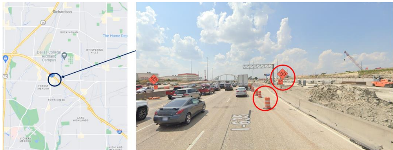
Figure 87. Setting 2: Intersection at Loop 12/Buckner Blvd and I-30 Frontage Rd.
