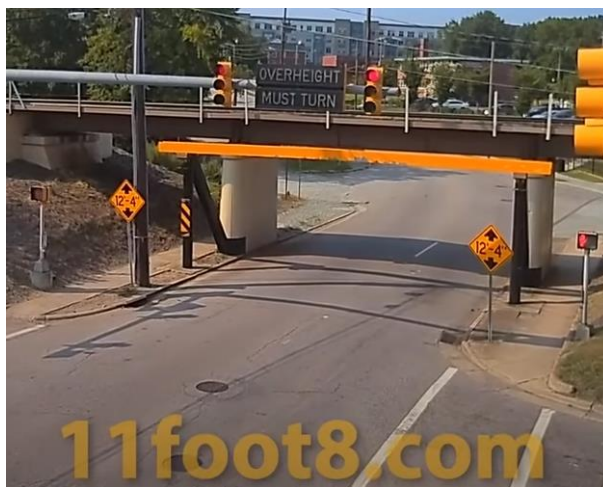
Figure 4. Overheight Detection and Warning Measures in Durham, North Carolina.
