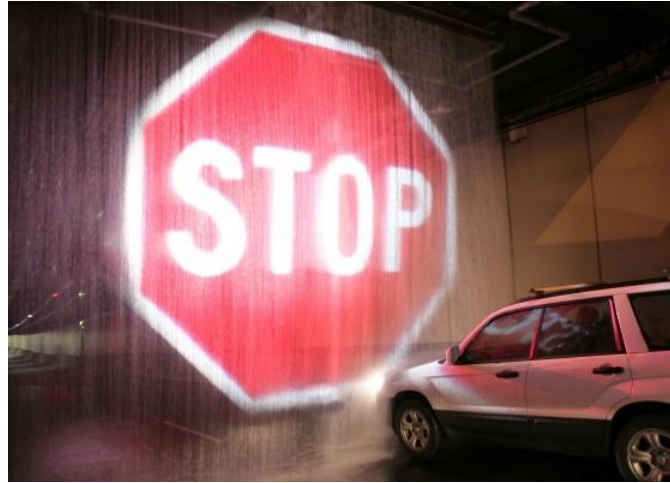
Figure 5. Stop Sign on Water Curtain, Sydney Harbour Tunnel.
