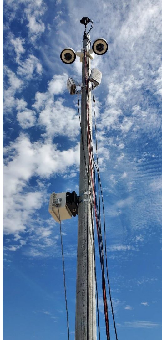
Figure 50. TAPCO® Equipment for Testing.
