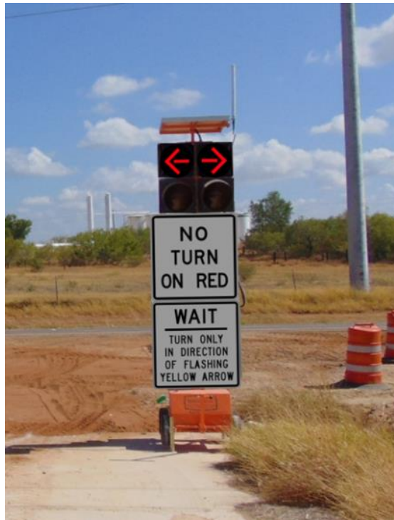
Figure 26. Stop Four-Section Stacked DAD.
