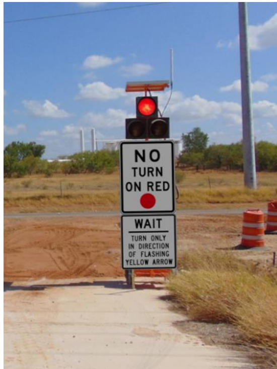
Figure 23. Stop Three-Section Doghouse DAD.
