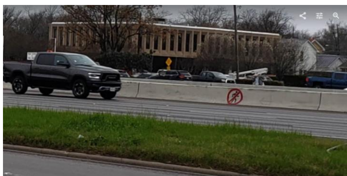
Figure 32. No Pedestrian Crossing Stencil and Signs on IH 35 in Austin.
