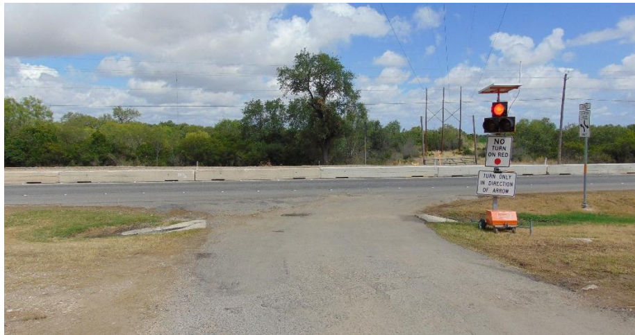
Figure 49. Project 1 DAD at Residential Driveway NB-12.
