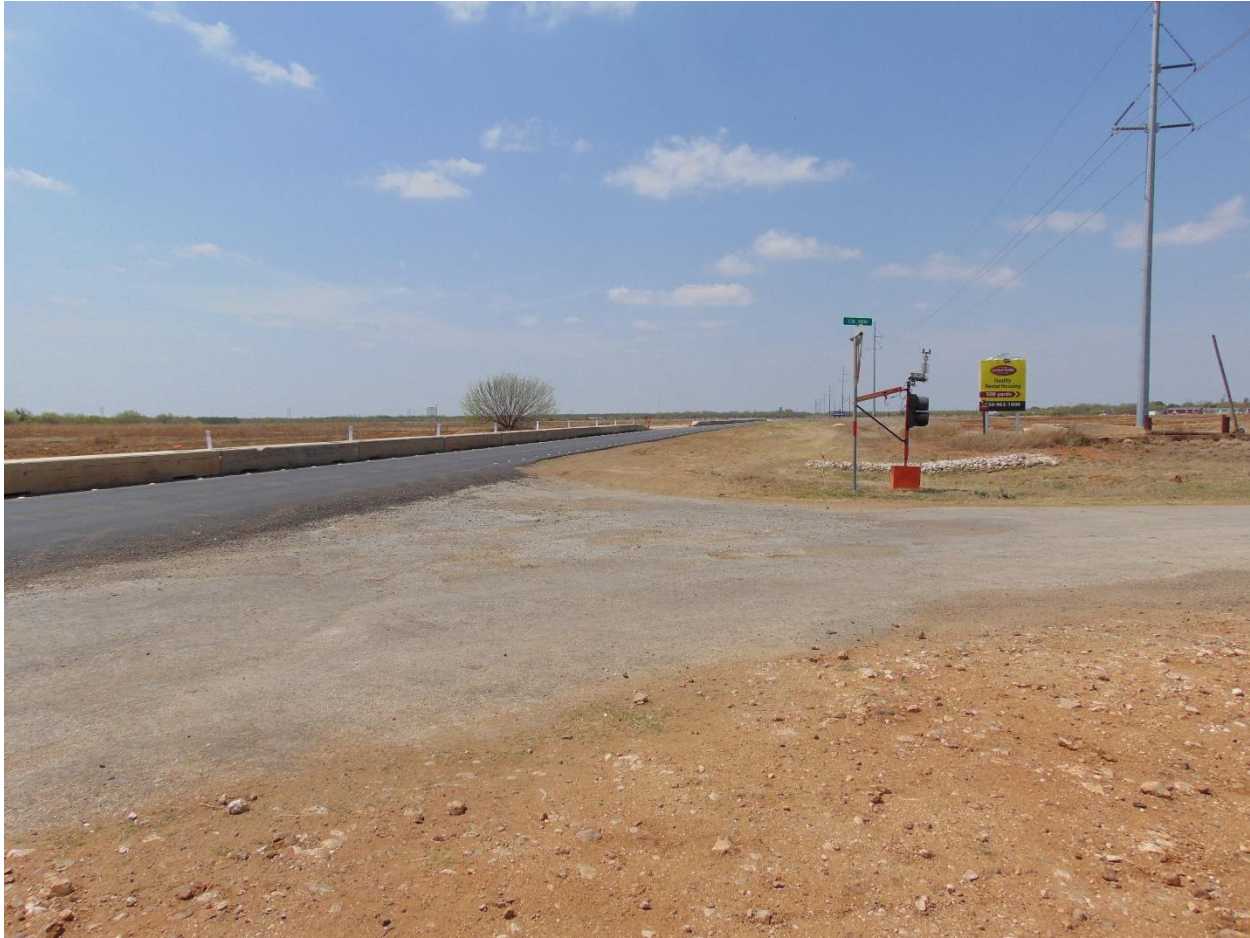
Figure 56. Project 2 DAD at Intersection of SH 85 and CR 3800—Looking West.
