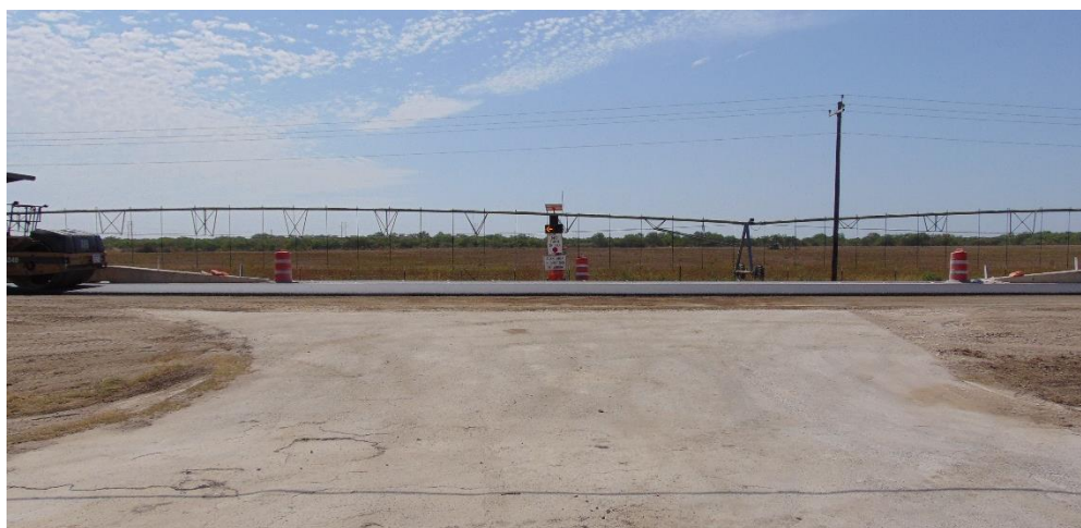
Figure 47. Project 1 DAD at Business Driveway SB-33.
