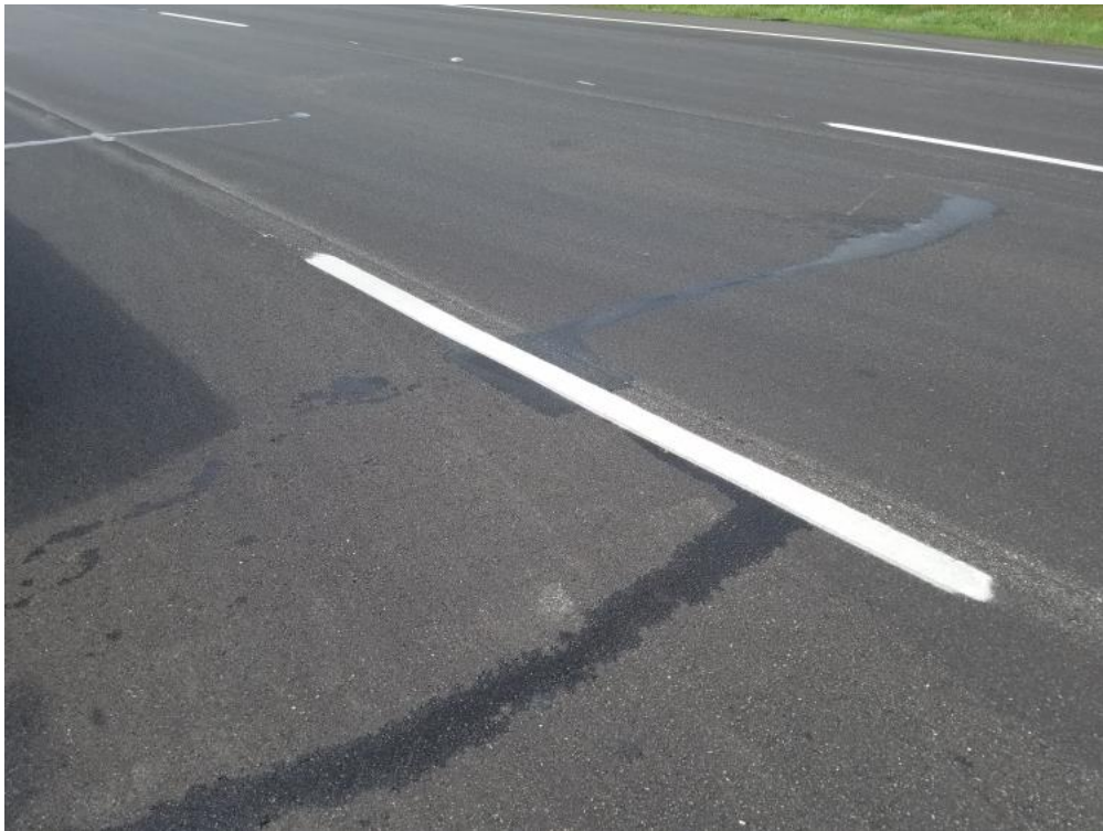
Figure 2. White Marking after Wet Retroreflectivity Evaluation.
