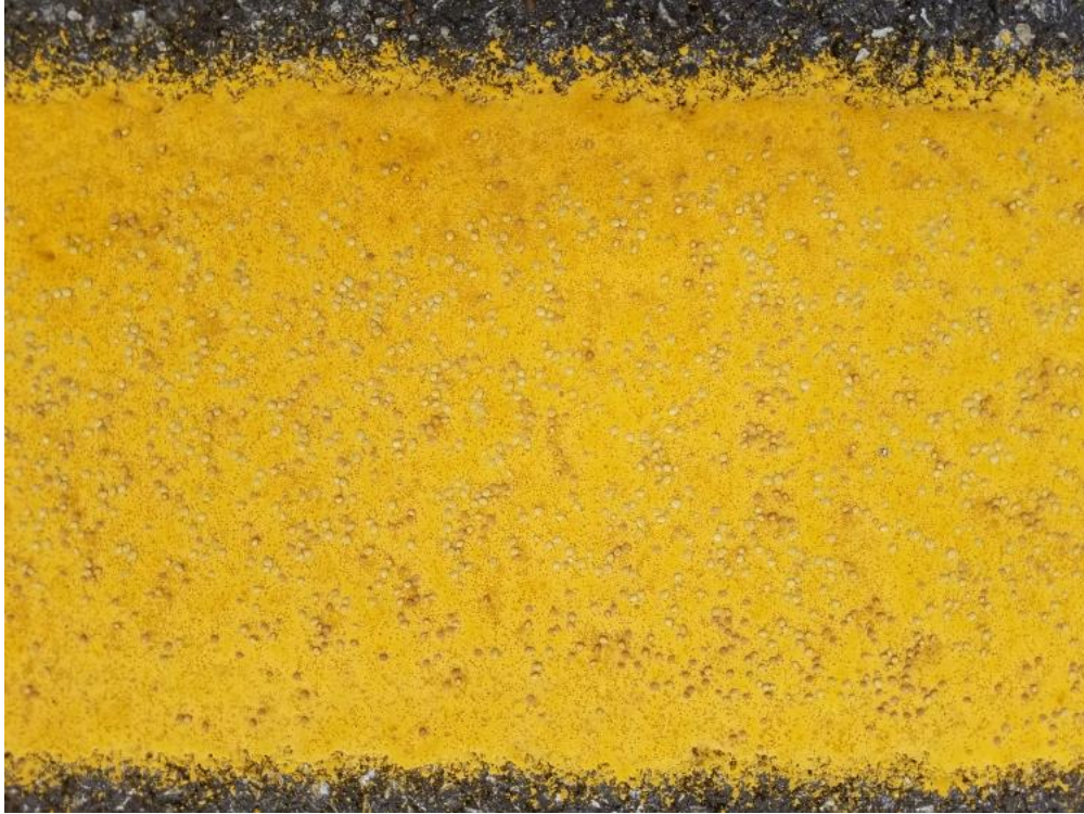
Figure 6. Yellow All-Weather Marking with Discolored Wet-Weather Optics.
