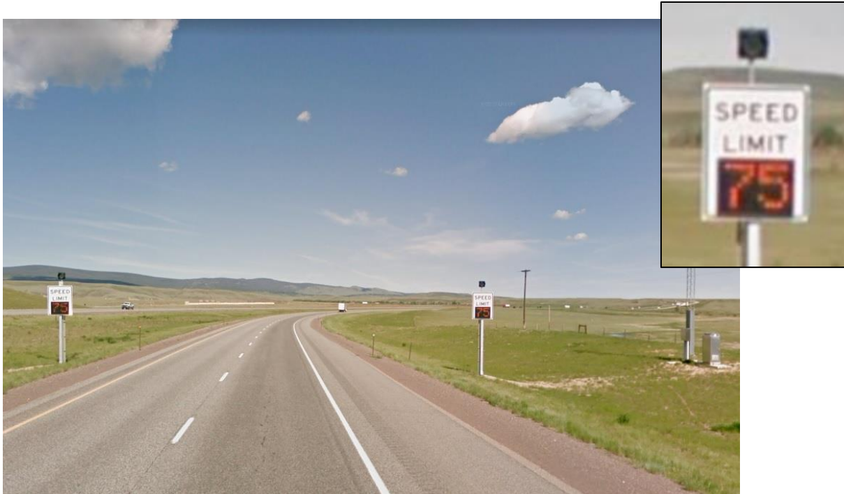
Figure 17. WYDOT IH 80 Variable Speed Limit Installation.
