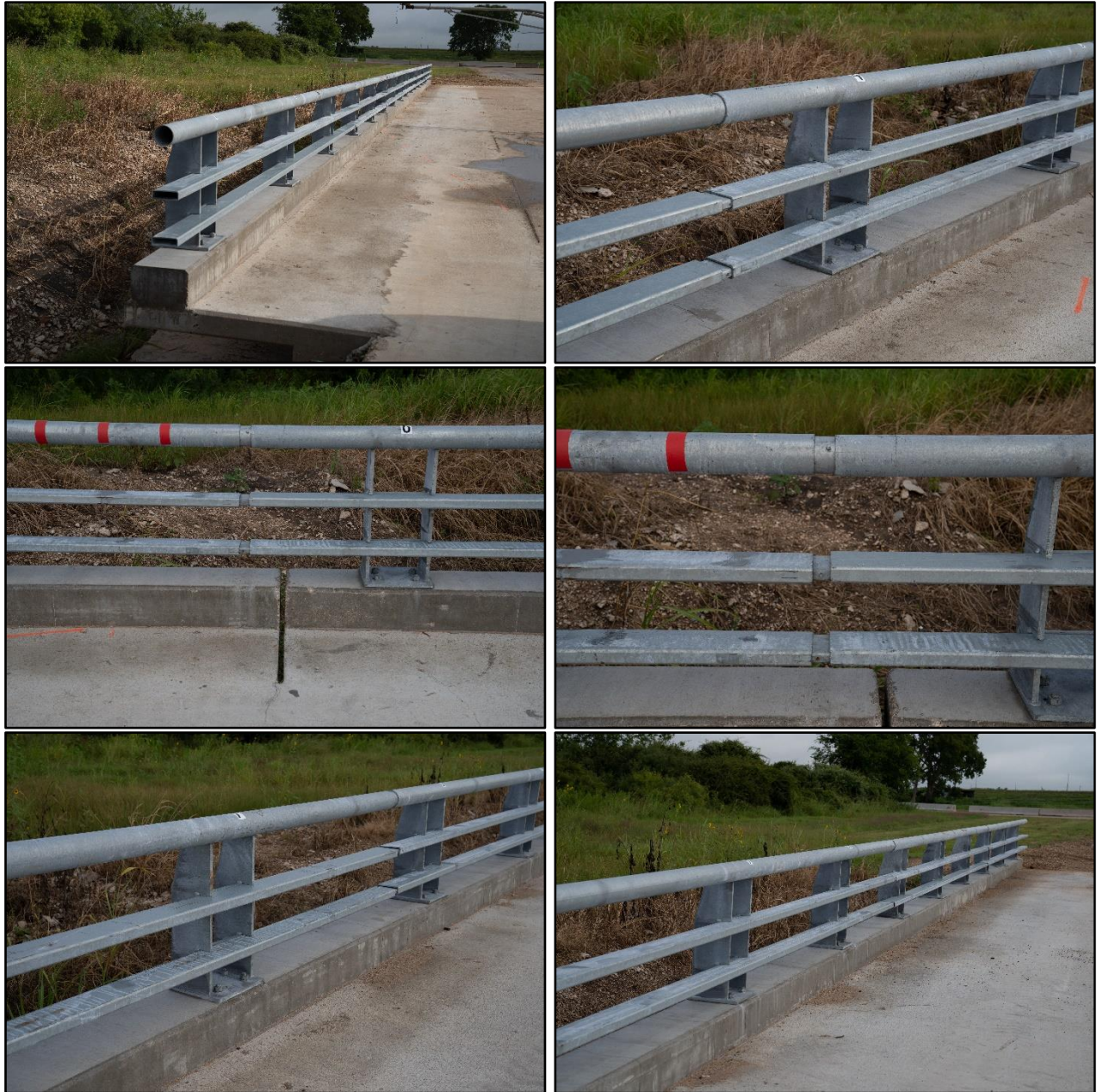
Figure 2.2. TxDOT T2P Retrofit Bridge Rail prior to Testing.
