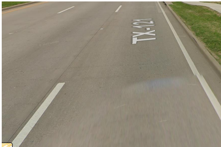
Figure A15. Presence of Curb.
