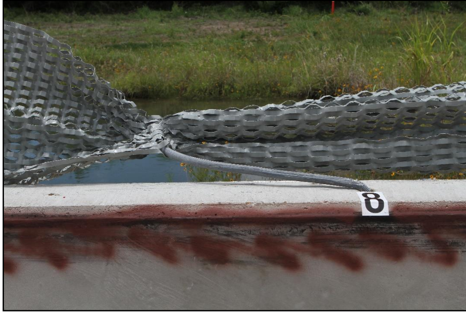
Figure 6.7. Screen-Safe® Glare Screen on Single-Slope Barrier after Test at Post 8, Test 440822-01-2.
