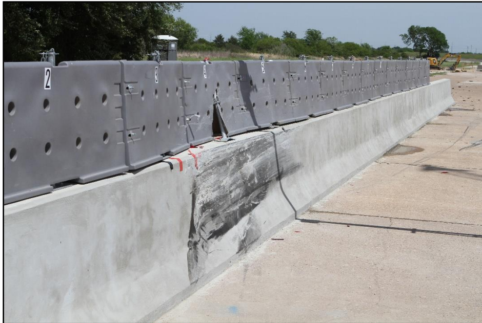
Figure 7.6. Armorcast® Gawk Screen on F-Shape Barrier after Test at Impact Location, Test 440822-01-3.
