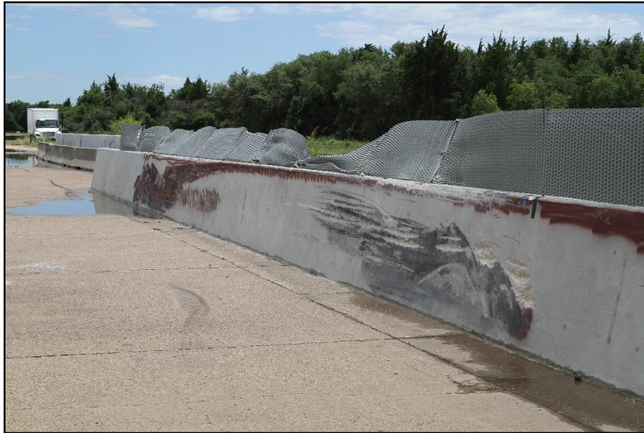
Figure 6.6. Screen-Safe® Glare Screen on Single-Slope Barrier after Test at Impact Location, Test 440822-01-2.
