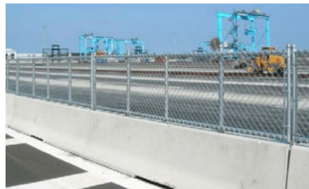
Figure 2.1. Chain-Link System for Concrete Barriers (4).
