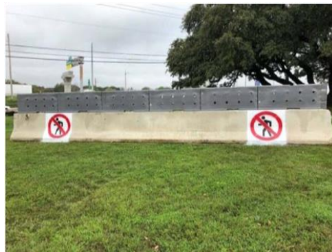
Figure 2.5. Barrier with Sign and Attachment (7).
