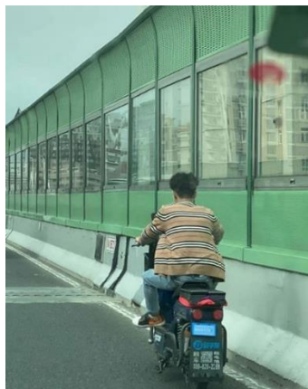
Figure 2.13. Bridge Rail Wall Installation for Noise Reduction in China (11).
