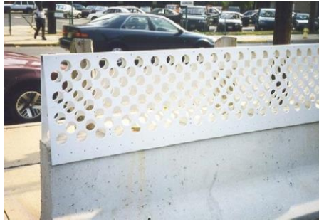
Figure 2.9. Prototype of Side-Mount CGSPF Using Recycled Plastics (8).
