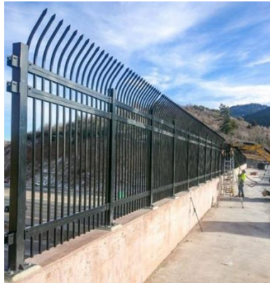
Figure 2.12. Ornamental Pedestrian Bridge Railing (10).
