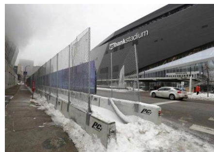
Figure 2.2. Chain-Link System for Concrete Barriers in Minneapolis (5).
