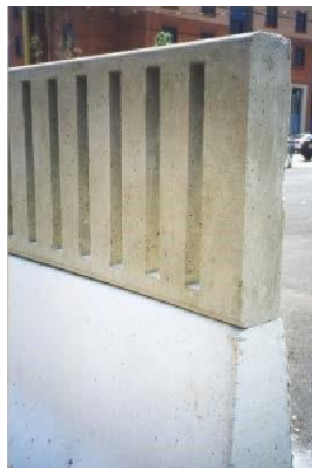
Figure 2.8. Modified Concrete Glare Screen (8).
