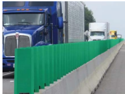
Figure 2.4. Modular Glare Screen (6).
