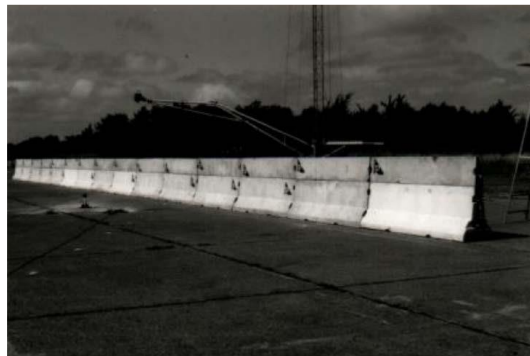
Figure 2.7. Concrete Median Barrier Retrofitted with Concrete Glare Screen.
