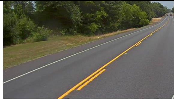
Example Current Condition Photo 2
