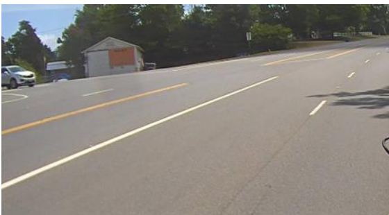
Example Current Condition Photo 1
