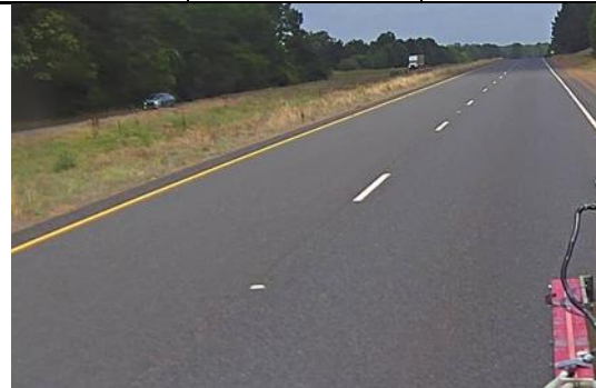
Example Current Condition Photo 2
