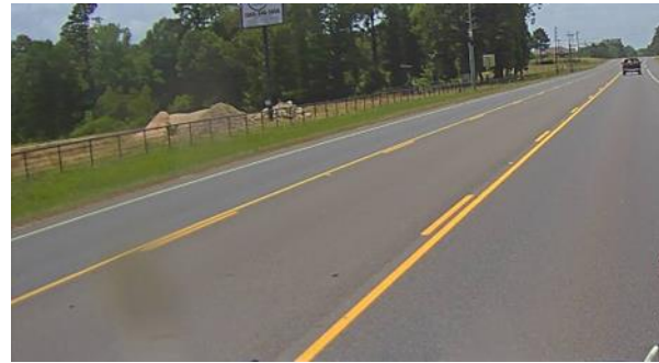
Example Current Condition Photo 2
