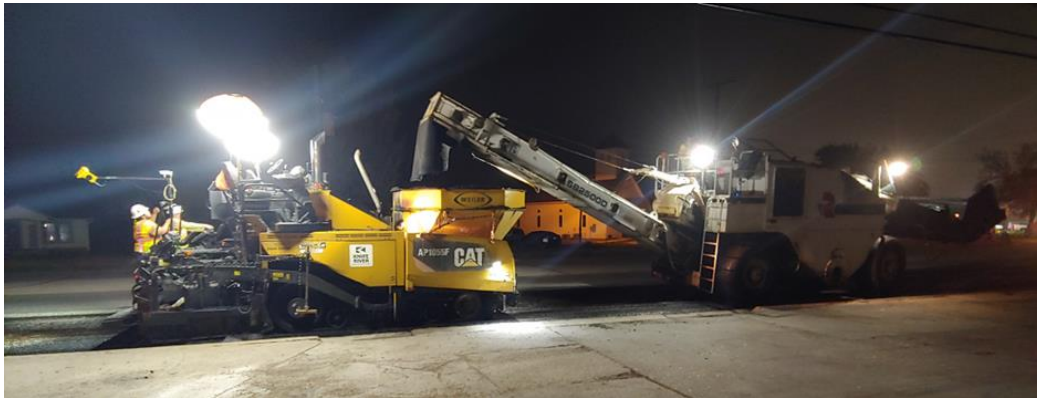
Figure 69. Paving Operation on SH 105.
