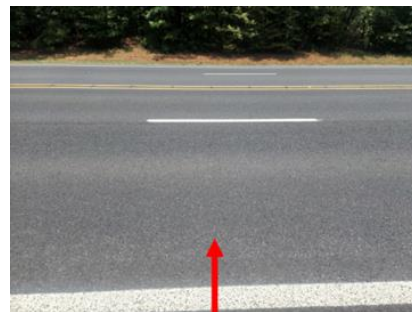
Example Current Condition Photo 2
