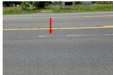
Example Current Condition Photo 2
