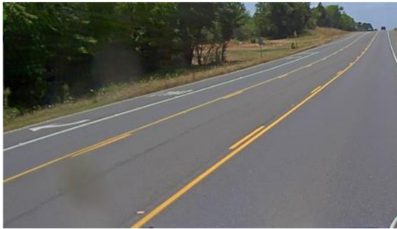
Example Current Condition Photo 1
