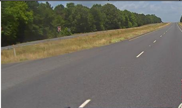
Example Current Condition Photo 1
