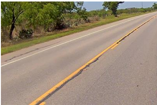
Example Current Condition Photo 1
