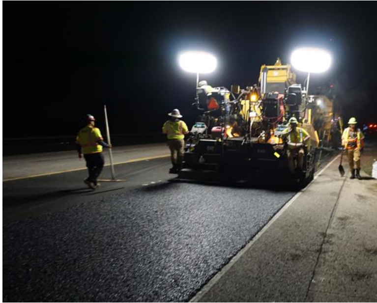
Figure 61. Paving Operation on SH 6.
