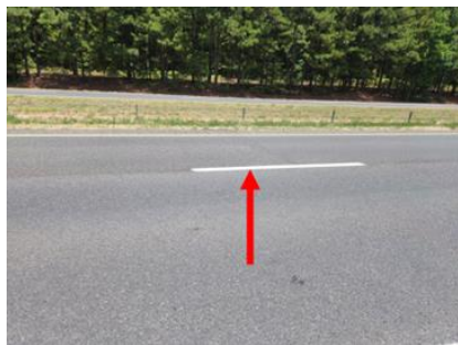
Example Current Condition Photo 1
