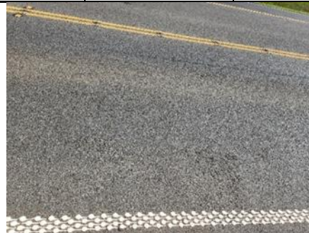
Example Current Condition Photo 2
