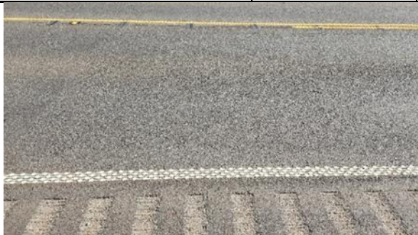
Example Current Condition Photo 1
