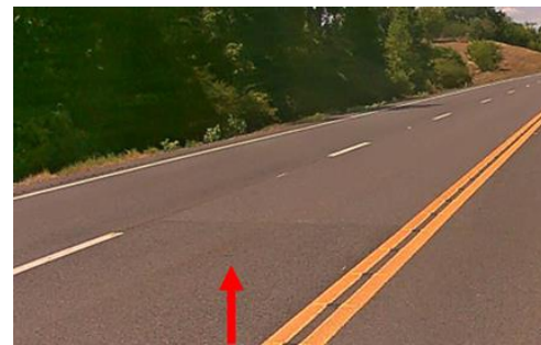
Example Current Condition Photo 2
