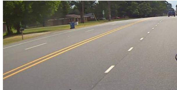
Example Current Condition Photo 2
