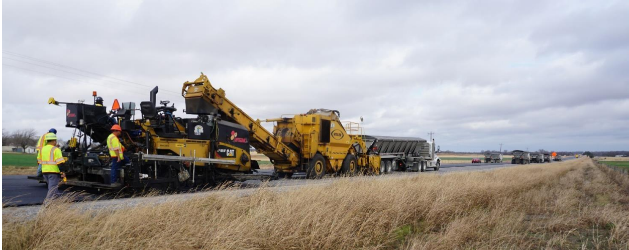
Figure 48. Paving Operation on US 183.
