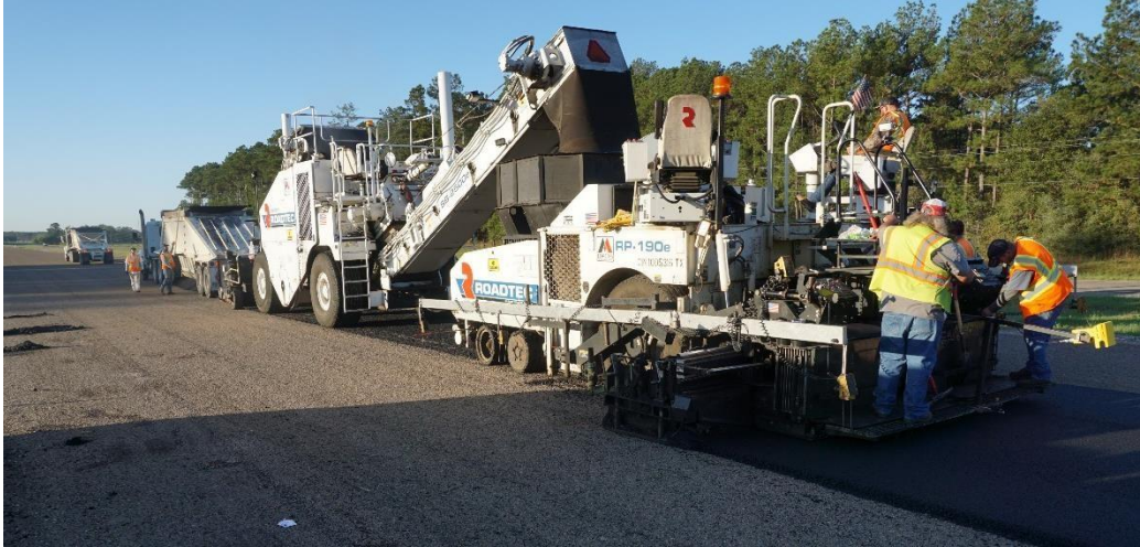
Figure 23. Paving Operation on US 69.
