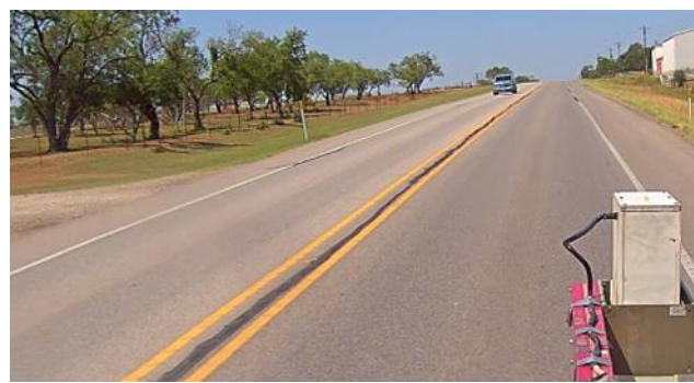
Example Current Condition Photo 2
