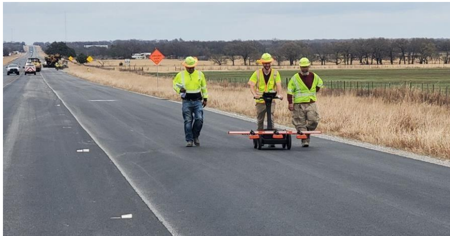
Figure 29. GPR Survey on the In-Place Mat with Multichannel GPR.
