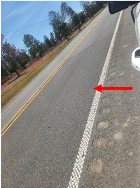
Example Current Condition Photo 1
