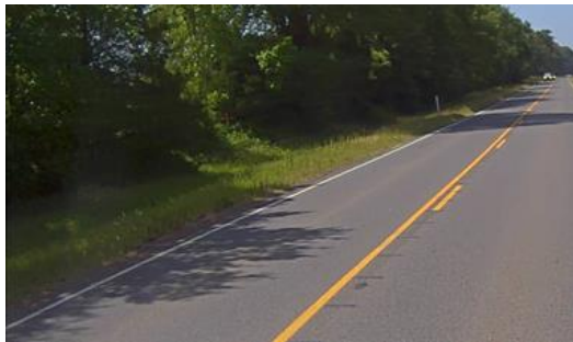
Example Current Condition Photo 1
