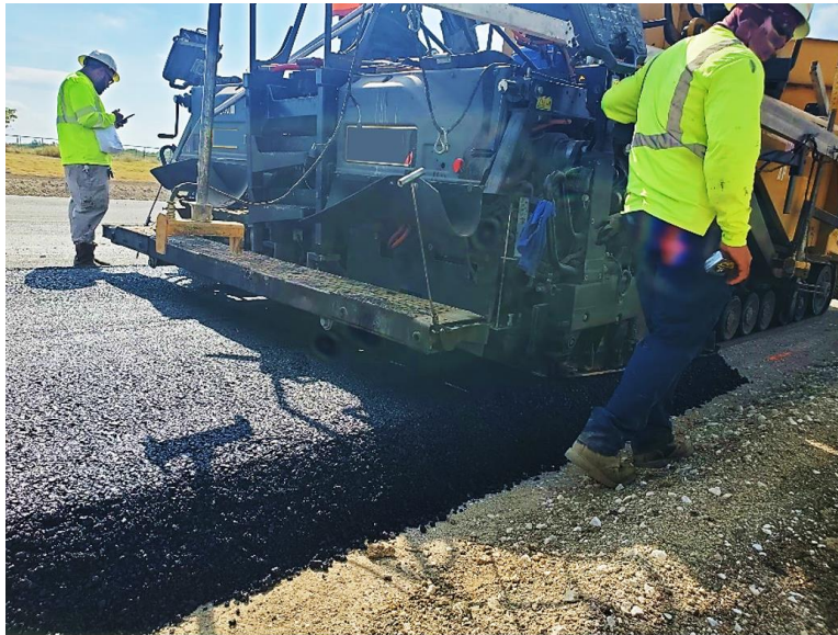
Figure 1. Thick-Lift Paving.
