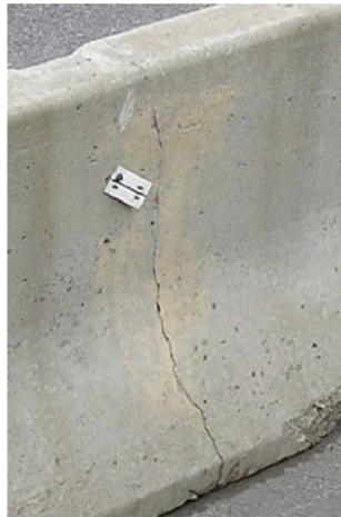
a. Acceptable barrier
