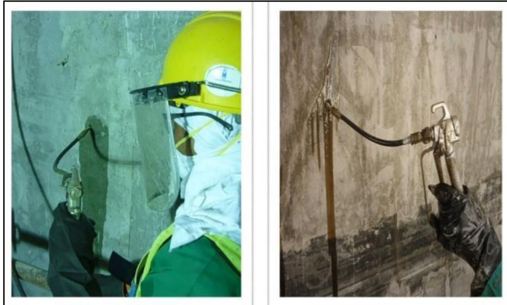
Figure 9.9. Injection of Epoxy Resin into the Holes (54).
