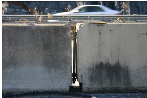
a. Acceptable barrier
