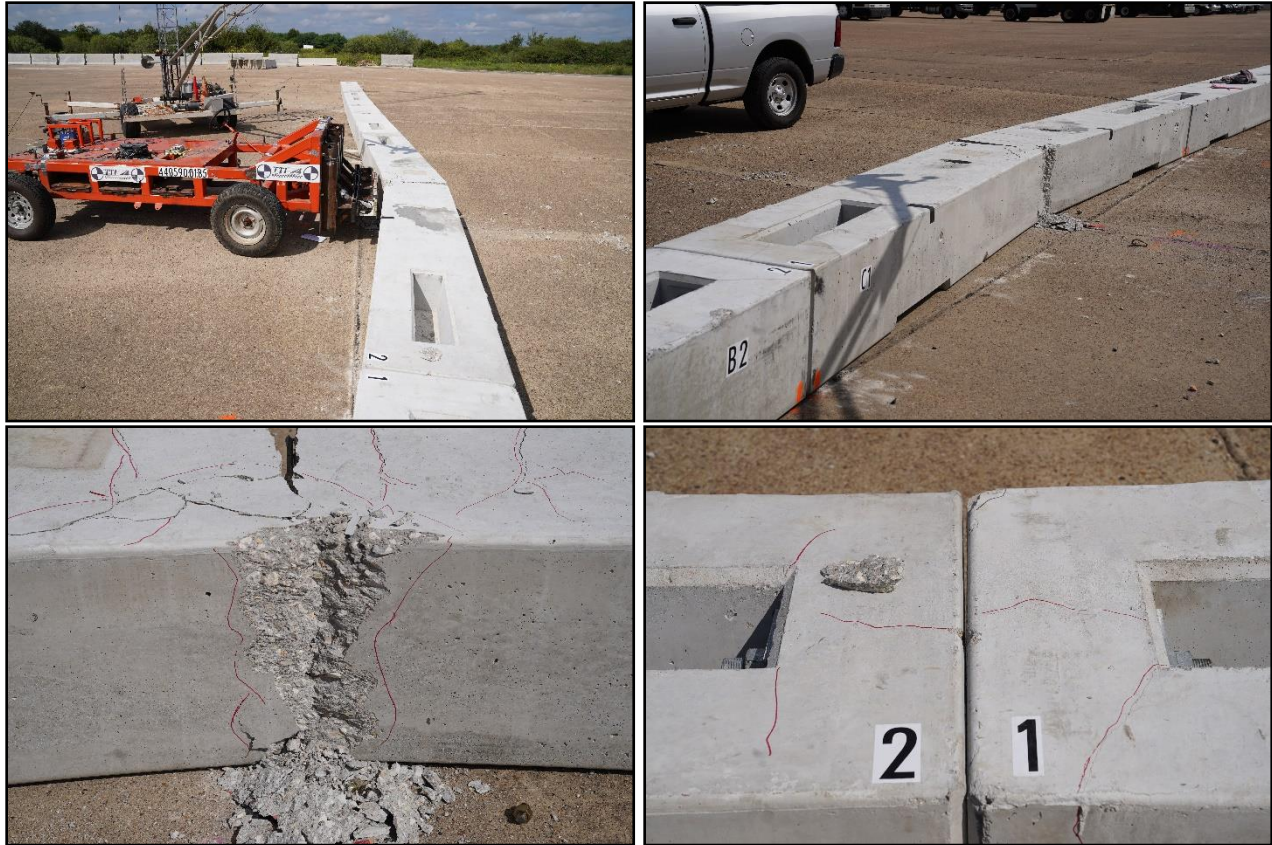
Figure 6.3. Low-Profile Barrier after Test No. 440591-01-B5.
