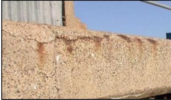
Figure 2.9. Crack Due to the Corrosion of Reinforcement (22).
