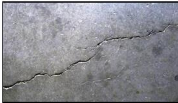
Figure 2.7. Shrinkage Cracks (18).
