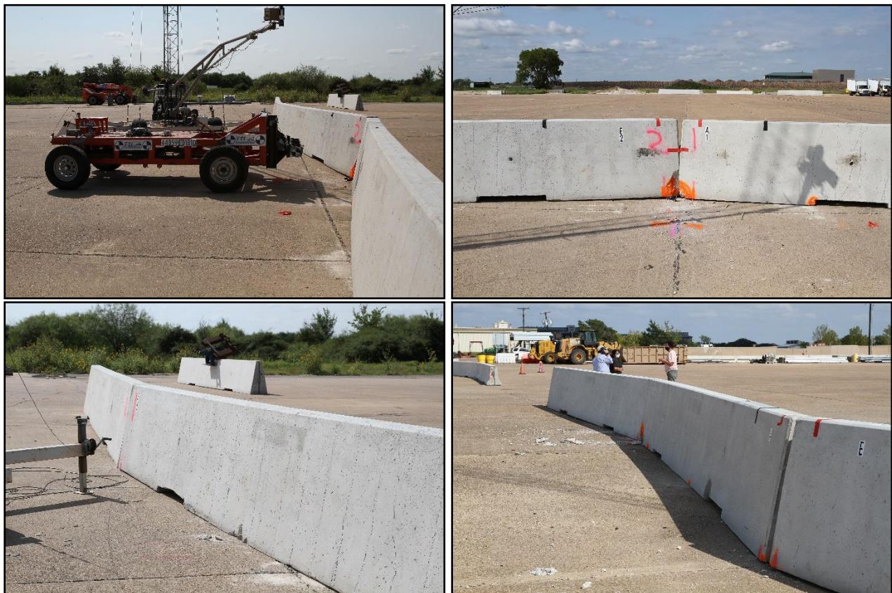
Figure 5.24. Single-Slope Barrier after Test No. 440591-01-B10.
