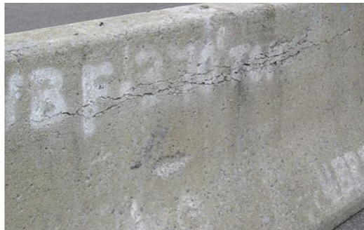
Figure 2.13. Longitudinal Cracks—NYSDOT (27).
