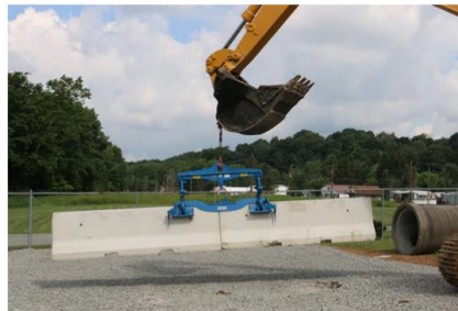
d. Two-point lifting (15)
