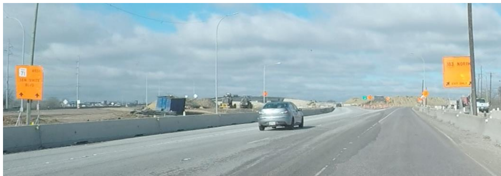
Figure 16. Temporary Lane Guidance Signs at Interchange Exit.
