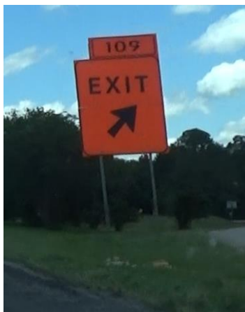
Figure 13. Exit Gore Sign for Exit 109.
