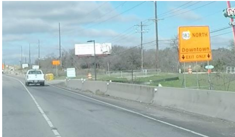
Figure 14. Temporary Lane Guidance Sign with Down Arrows Used on Roadside.
