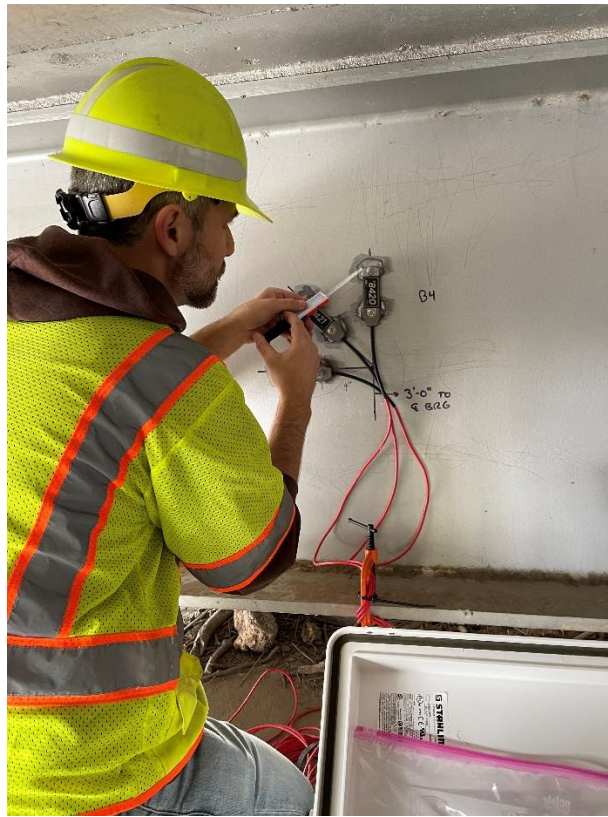
Figure 8.14. Apply Mix Epoxy around the Stain Gauge Tabs.
