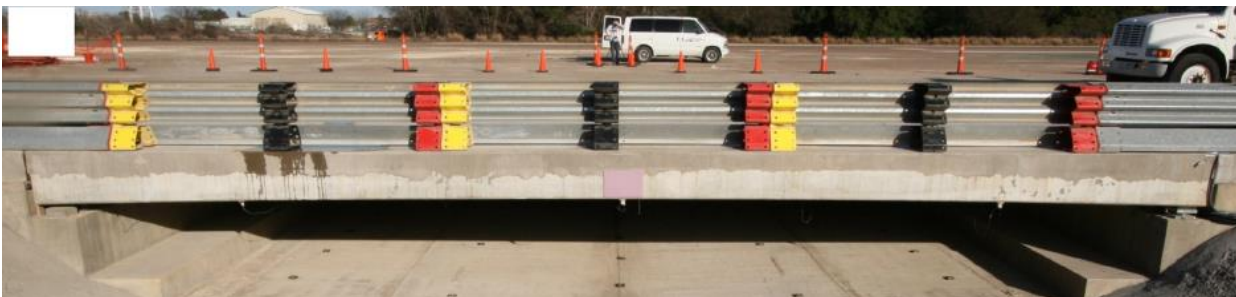
(c) Completed Bridge
