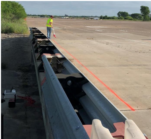
(b) Spray Paint to Mark the Lanes
