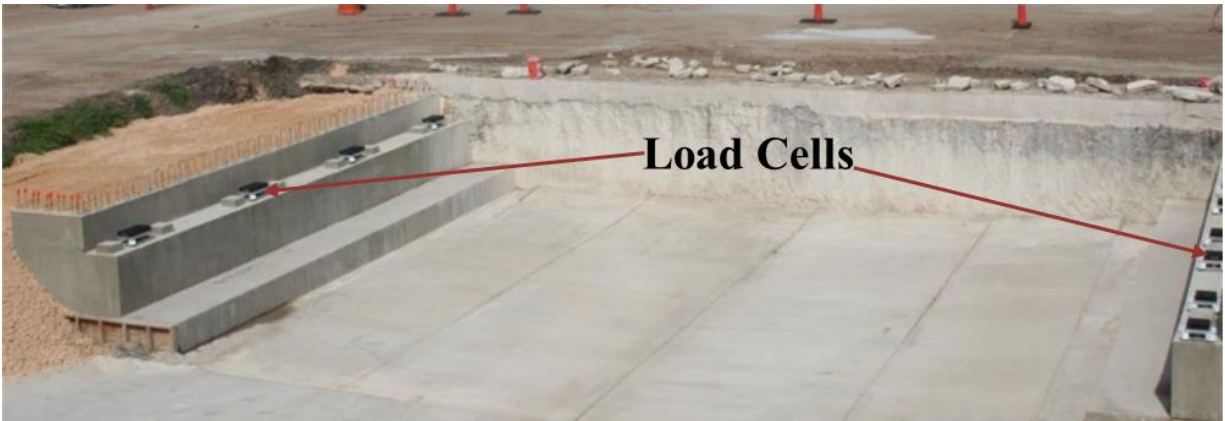
(a) Load Cells at South and North Ends
