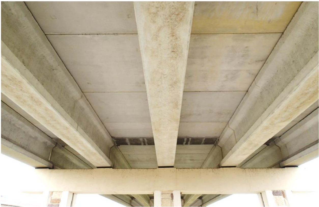
Figure 4.6: Bridge #2 Underside View.
