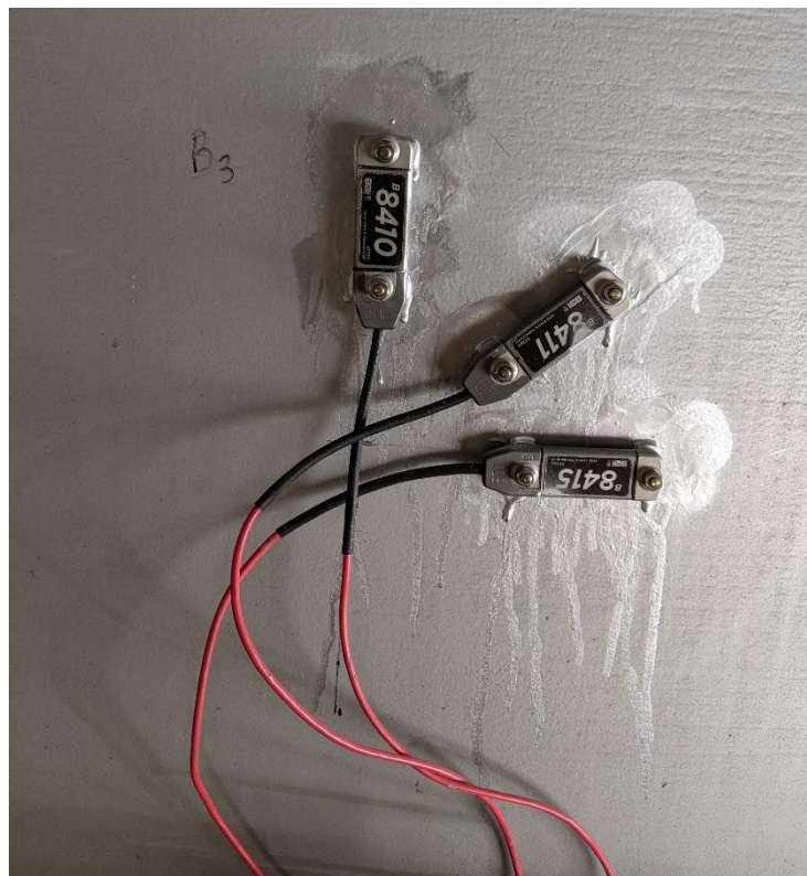
Figure 5.29. Strain Rosette at North End (Bridge #3).
