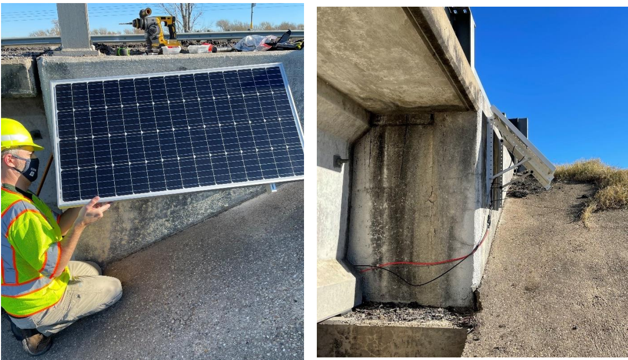
Figure 5.7. Installation of the Solar Panel.
