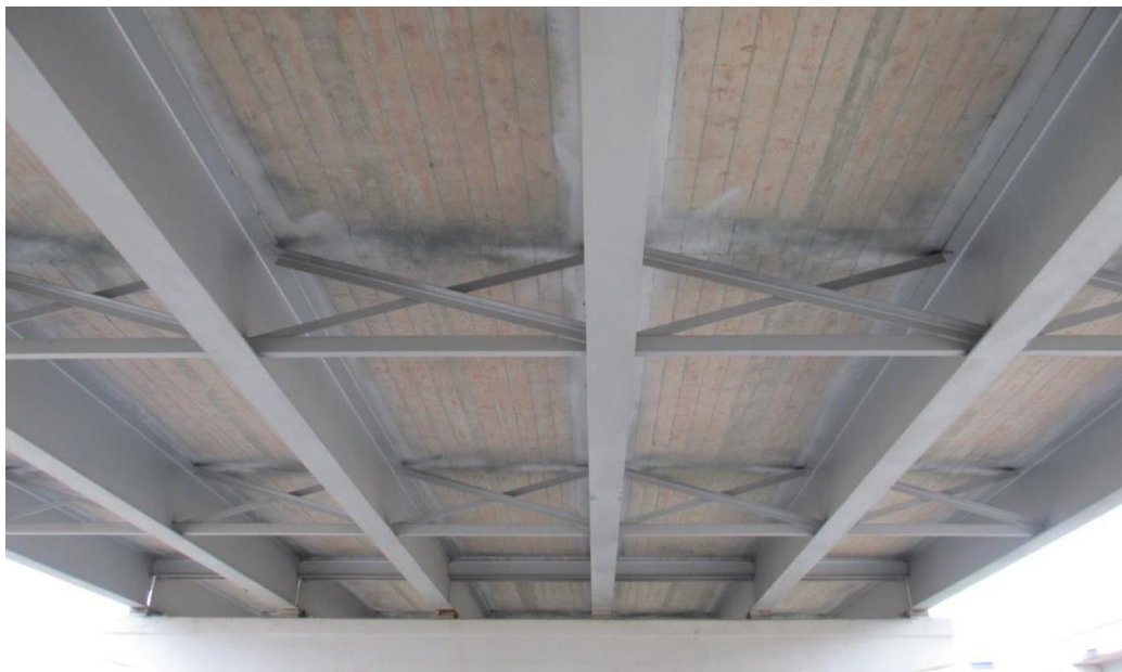
Figure 4.9: Bridge #3 Underside View.
