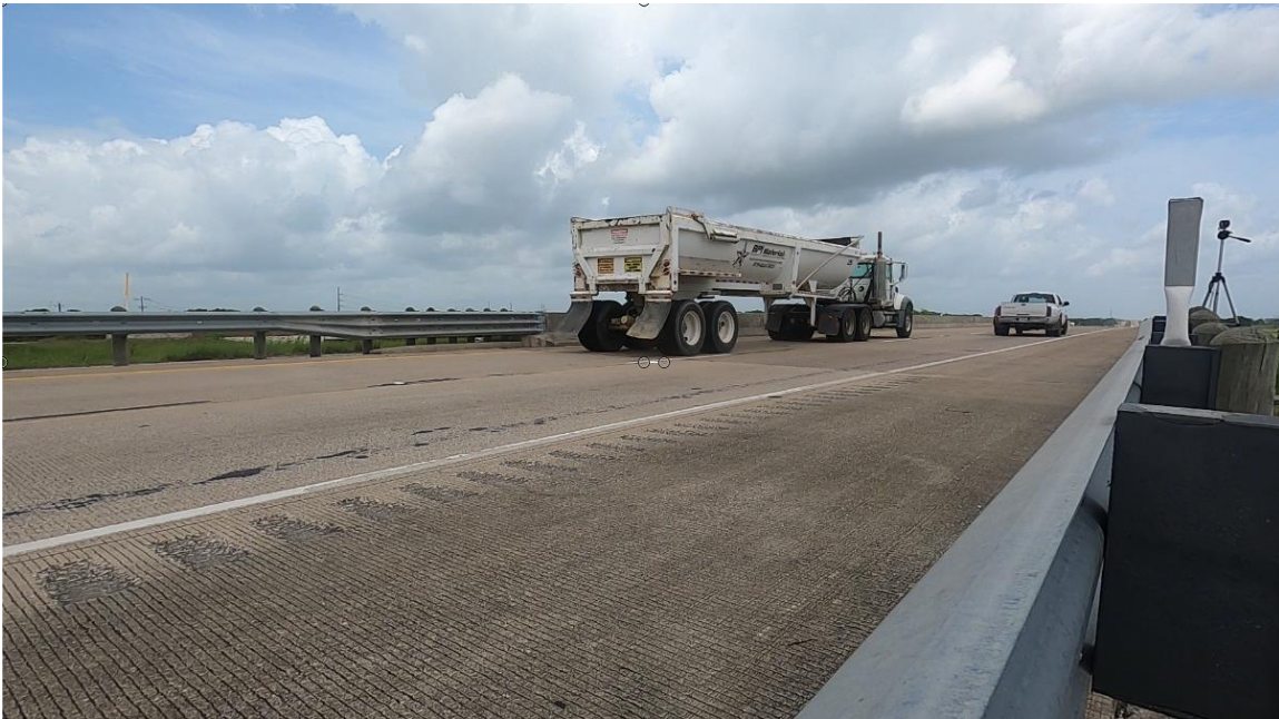
Figure 5.26. Truck Passing the Inside Lane (Bridge #2).
