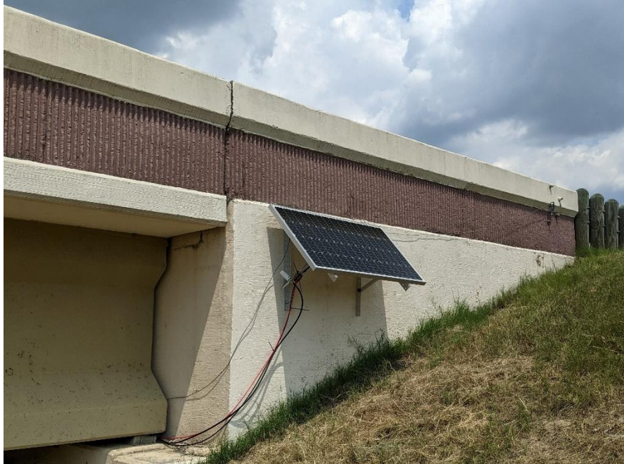
Figure 5.22. Installed Solar Panel (Bridge #2).
