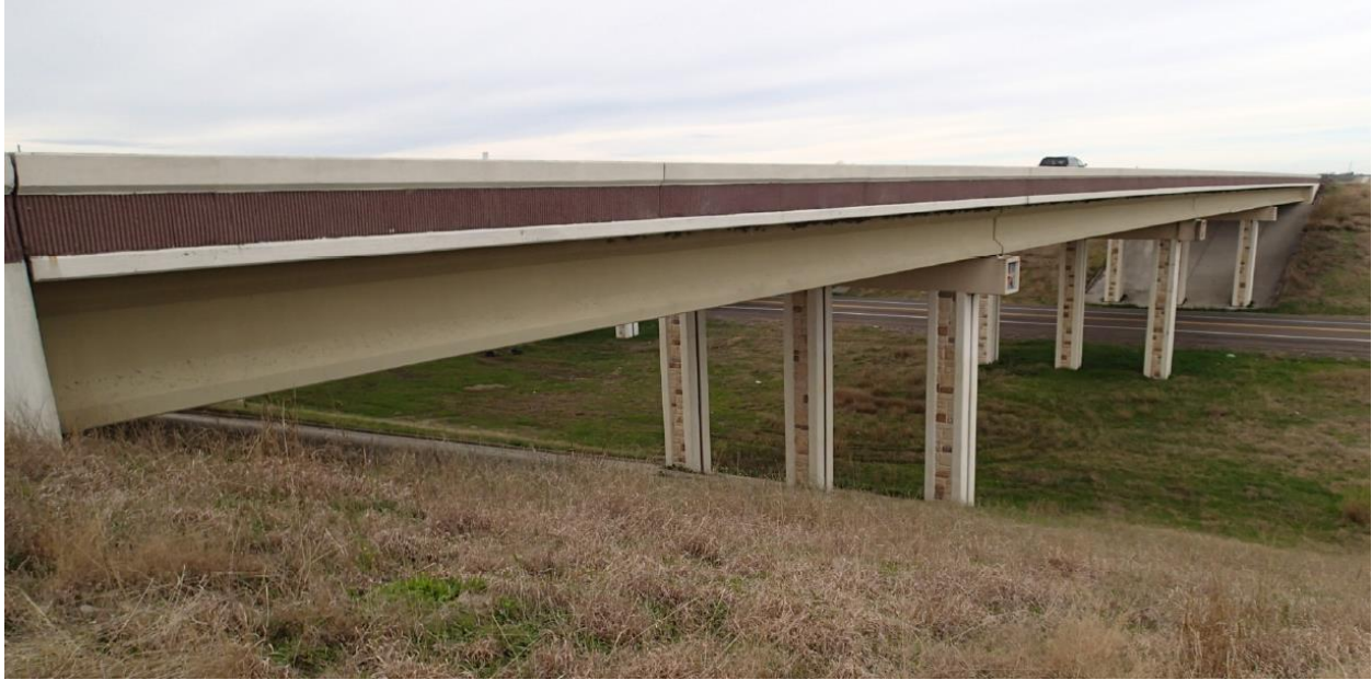
Figure 4.5: Bridge #2 Elevation View.
