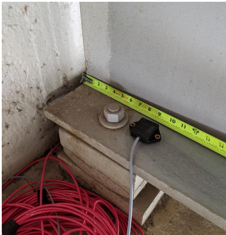
Figure 5.31. Accelerometer at North End (Bridge #3).
