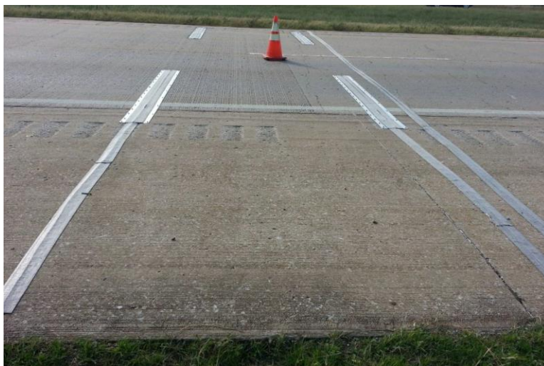
Figure 2.8. Two-Lane Portable WIM System Deployment (Refai et al. 2014).
