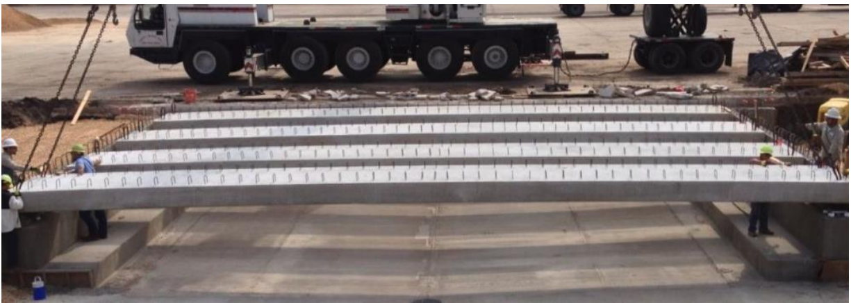
(b) Slab Beam Placement
