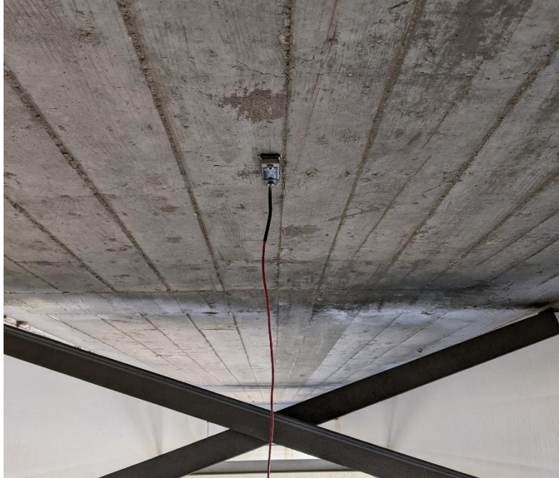
Figure 5.34. Strain Gauge Underneath the Bridge Deck (Bridge #3).
