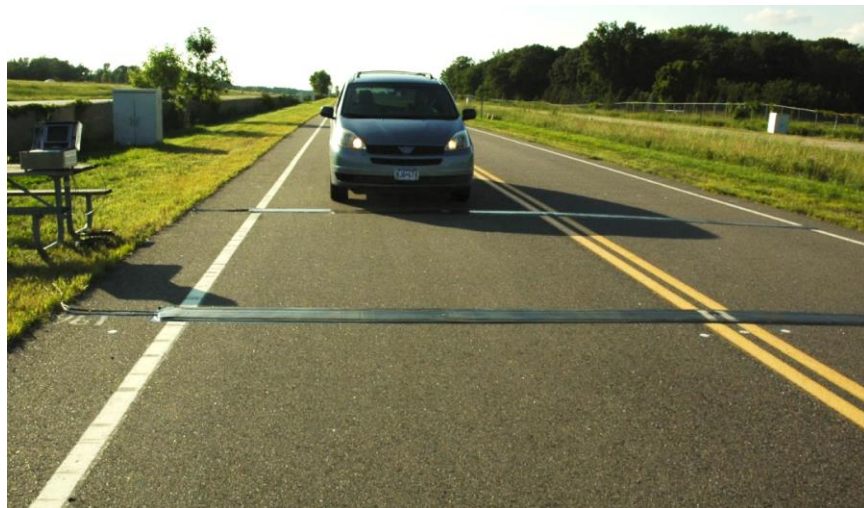
Figure 2.6. Installed Weigh Pads with Air Cavity and the Test Vehicle (Kwon 2012).
