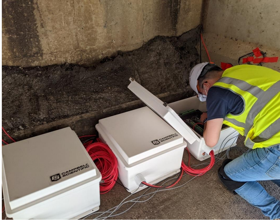
Figure 8.11. Placing Multiple Enclosures with Enough Distance.
