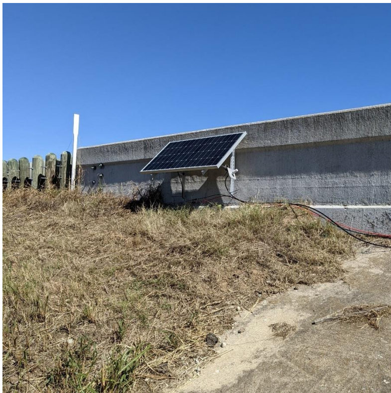
Figure 5.35. Installed Solar Panel (Bridge #3).
