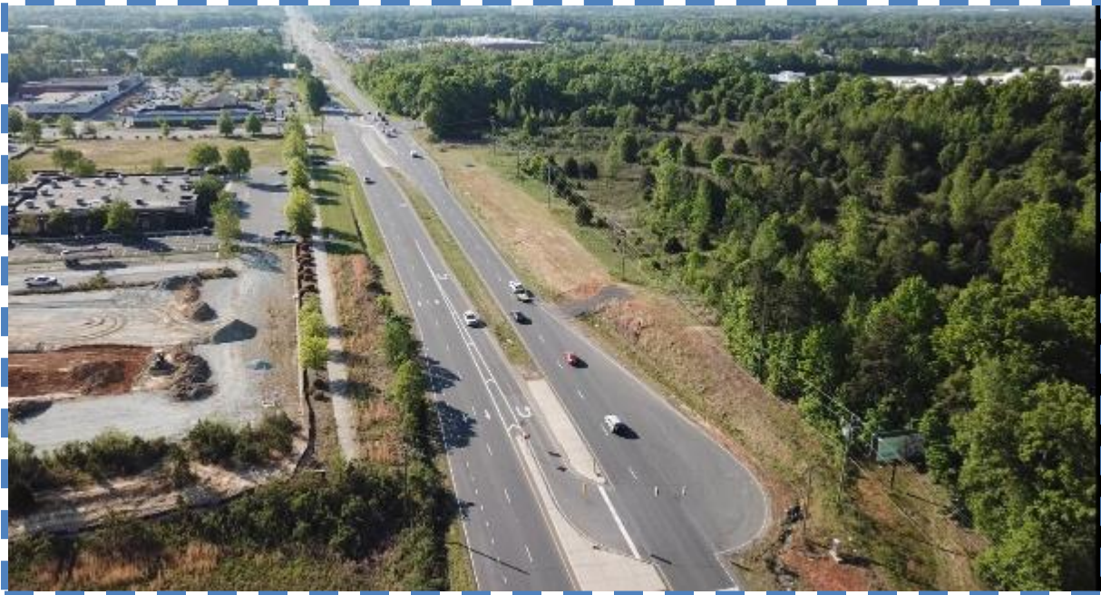
Figure 66. West Segment Camera View at Faith Church Road Site.
