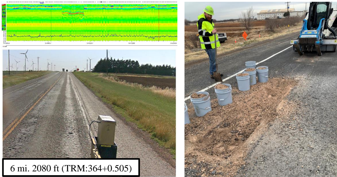
Figure 36. US 180 Initial Condition (Left) and Site Material Collection (Right).
