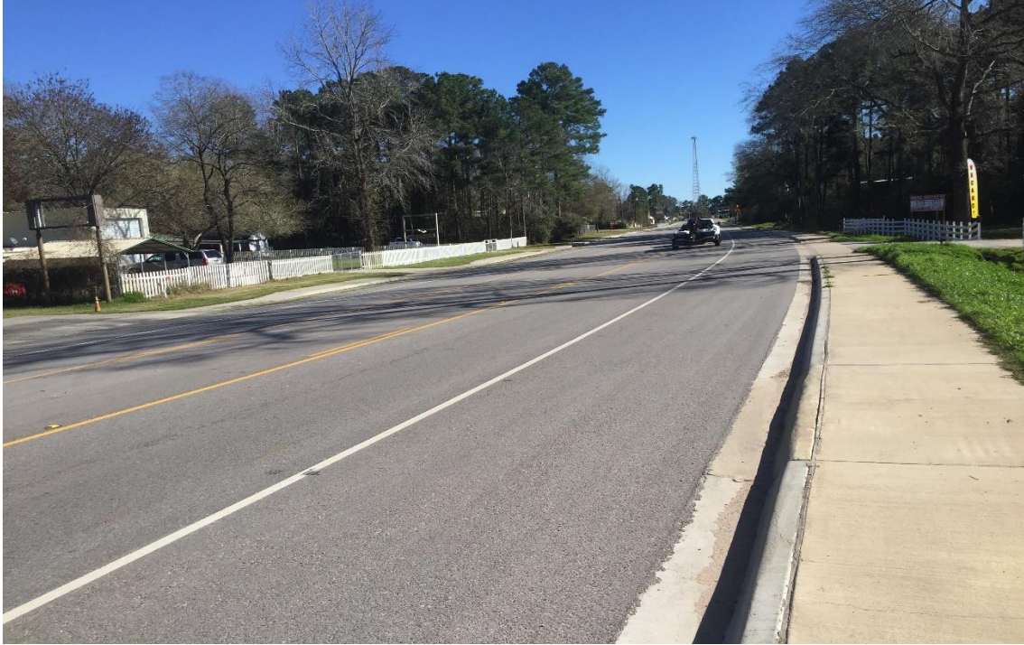
Figure 3-18. Photo Taken at the FM 356 Section in March 2020.
