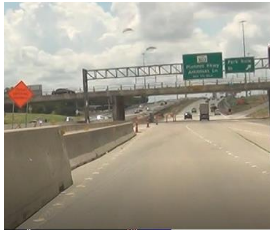
Figure 15. Example of Switching from a Single-Slope Barrier to an F-Shape Barrier near a Work Space Access Point.
