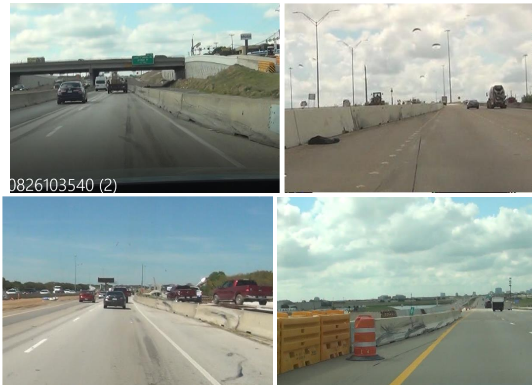
Figure 11. Examples Where Inconsistent Barrier Presence and Offset Distance Are Associated with Increased Tire Scuffs and Impact Scars.
