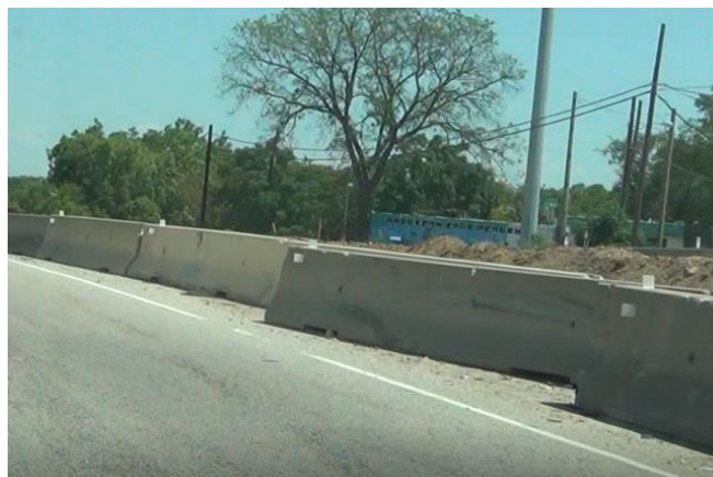
Figure 14. Example of an Unconnected Barrier Segment on a Horizontal Curve at an Entrance Ramp Merge Point.
