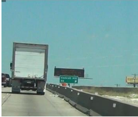
Figure 10. Example of a Large Truck Shying Away from the Work Zone Barrier.
