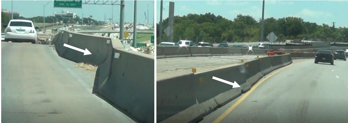
Figure 9. Examples of Barriers Deflected by Traffic Impacts (Left) or Construction Equipment (Right).
