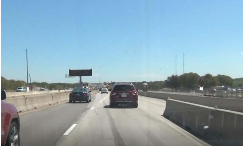
Figure 16. Example of a Short Acceleration Lane Adjacent to a Barrier at a Work Space Access Point.
