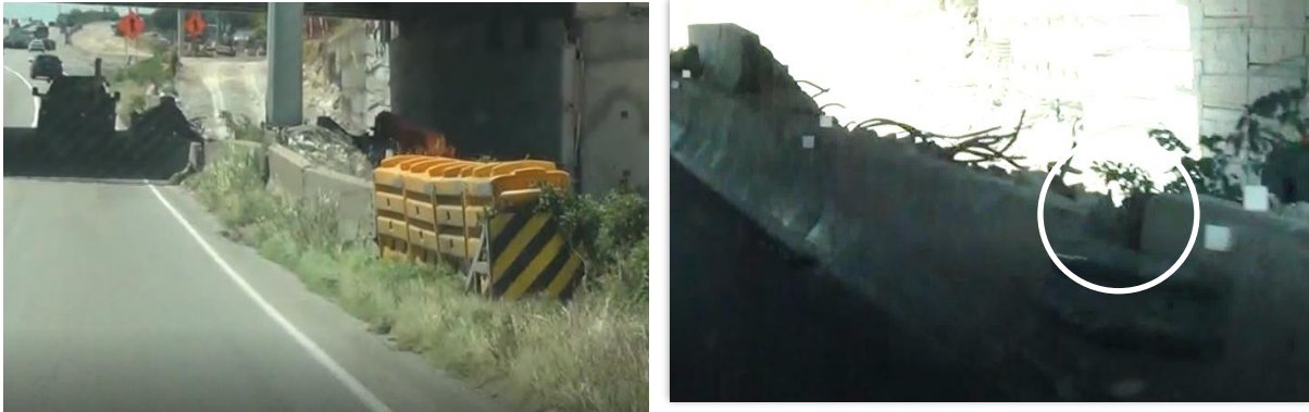
Figure 13. Barrier Segments with Nonstandard Deployment Heights and Connections.
