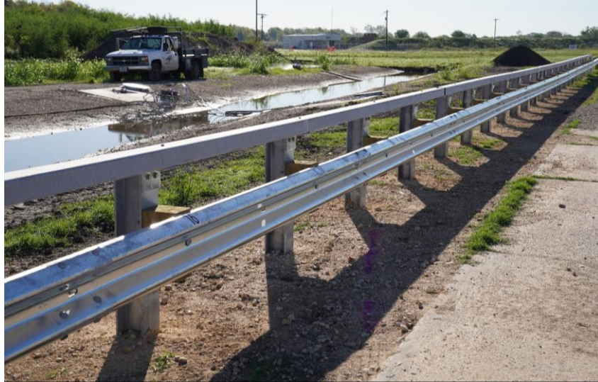
Figure 1. MASH TL-4 Guardrail Design.
