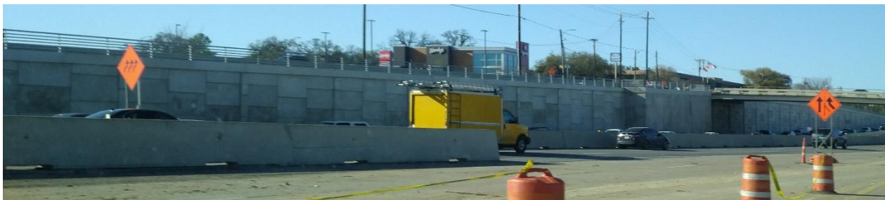
Figure 101. Retaining Wall B35.
