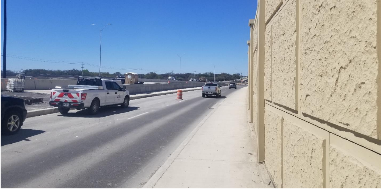
Figure 152. North-Facing View of SWNB04.
