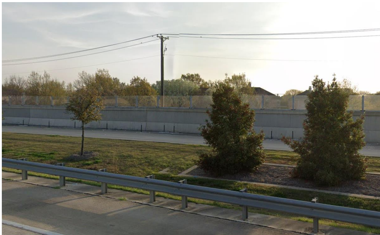
Figure 177. Noise Wall, President Bush Turnpike, Freeway Side.
