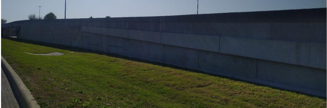
Figure 89. Retaining Wall B05B.
