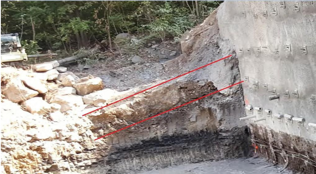
Figure 9. Encased Conduit Located during Construction (37).
