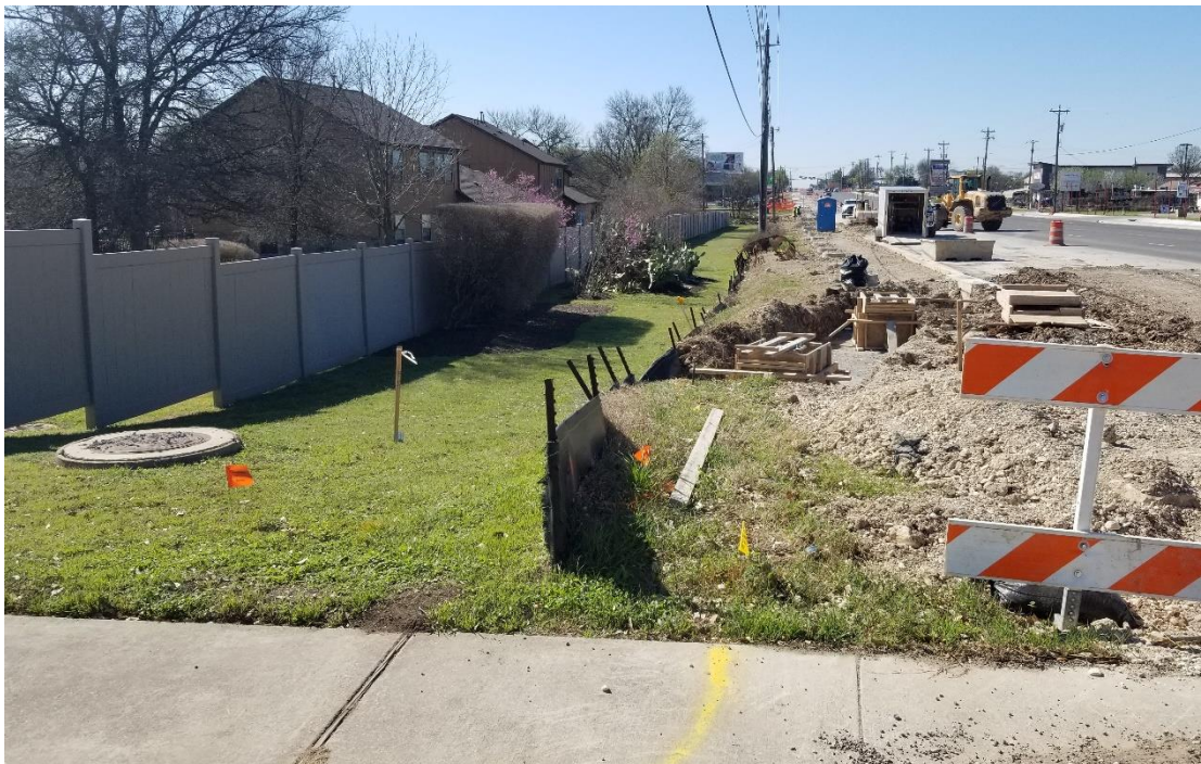
Figure 42. South-Facing View at North End of 1B.
