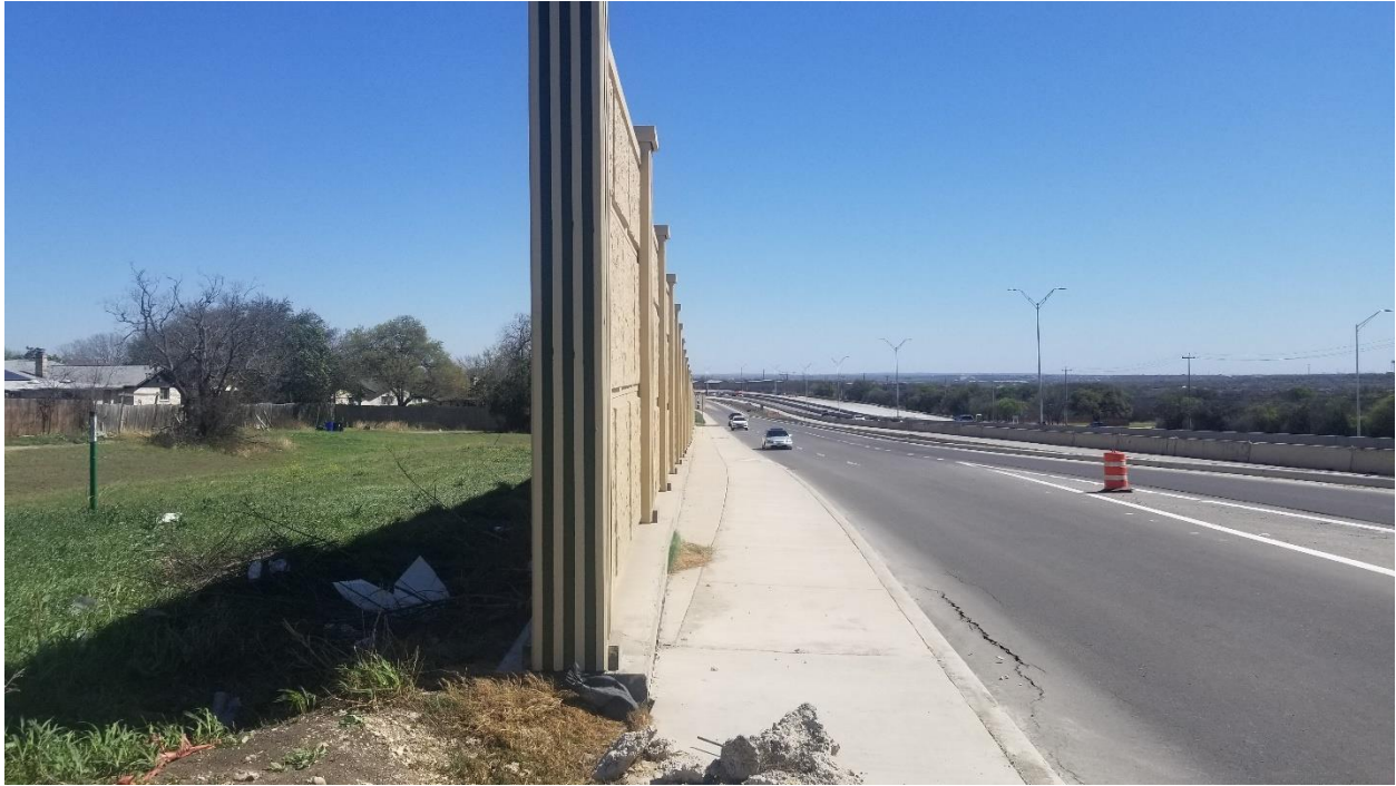
Figure 134. South-Facing View at North End of SWNB01.
