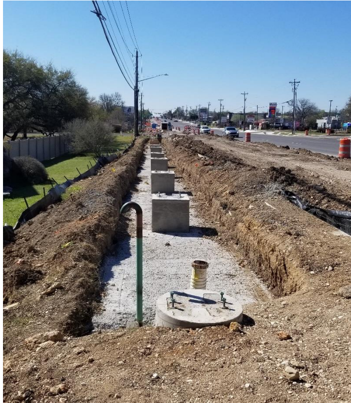
Figure 36. South-Facing View at 1A, North End of Spread Footing.
