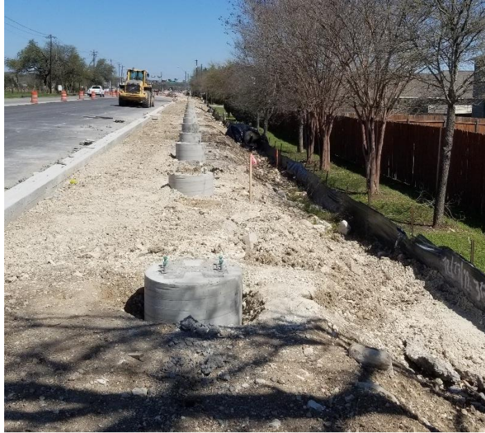
Figure 49. North-Facing View at South End of 2C.
