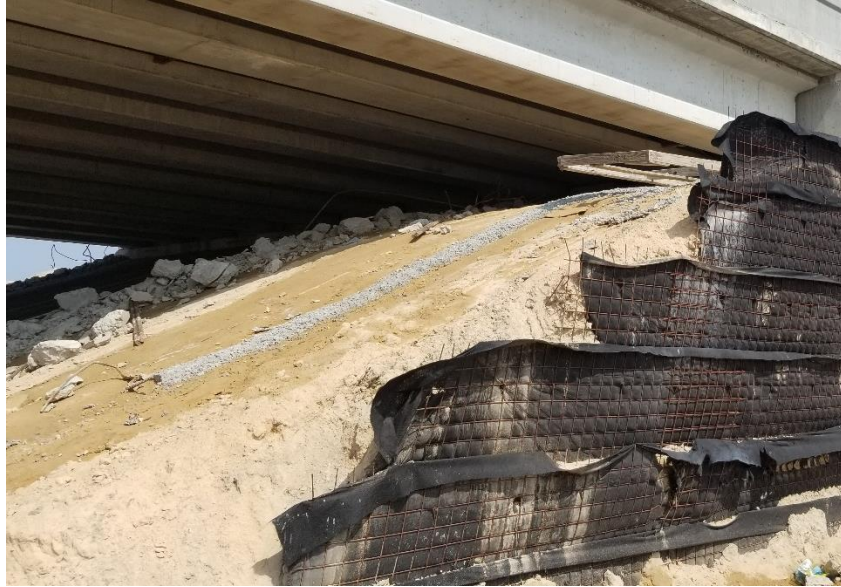
Figure 117. Southbound Side of RW 10.
