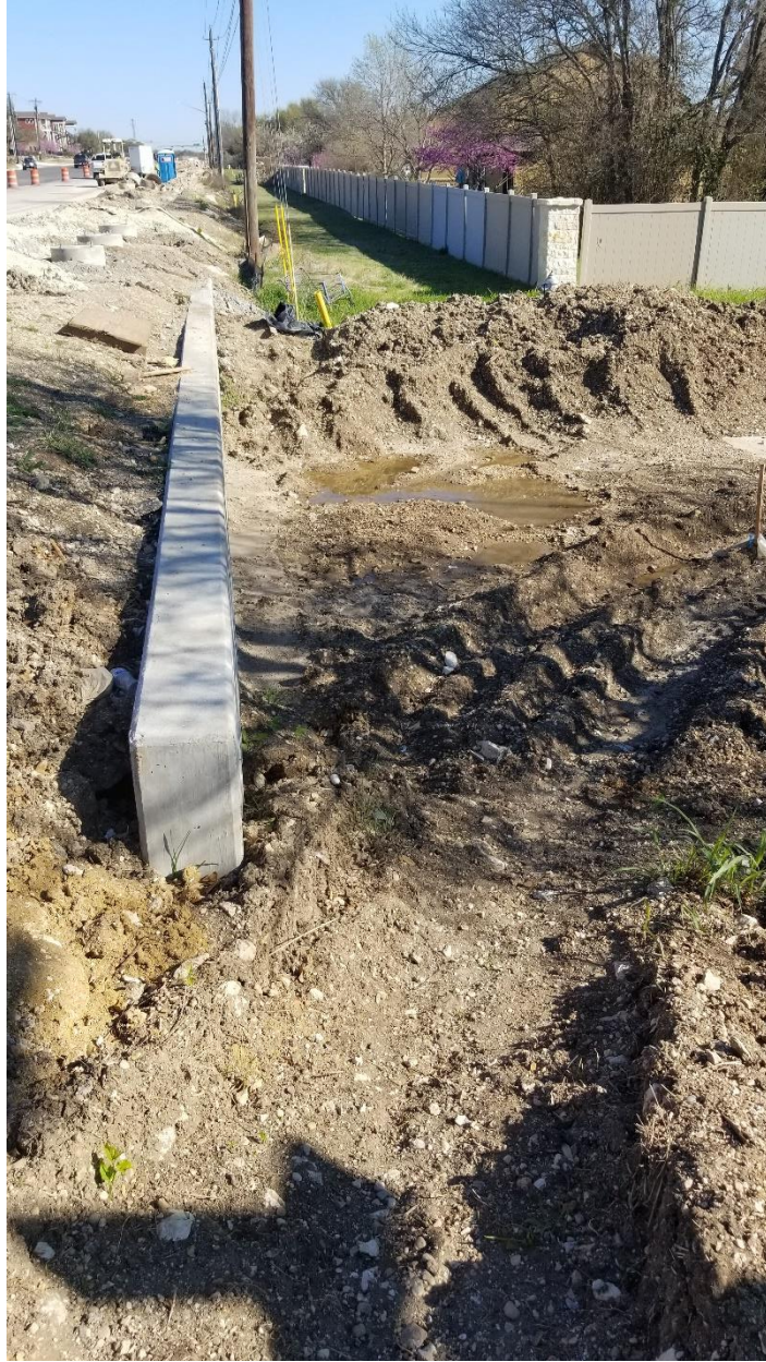
Figure 57. North-Facing View of Northbound Headwall.
