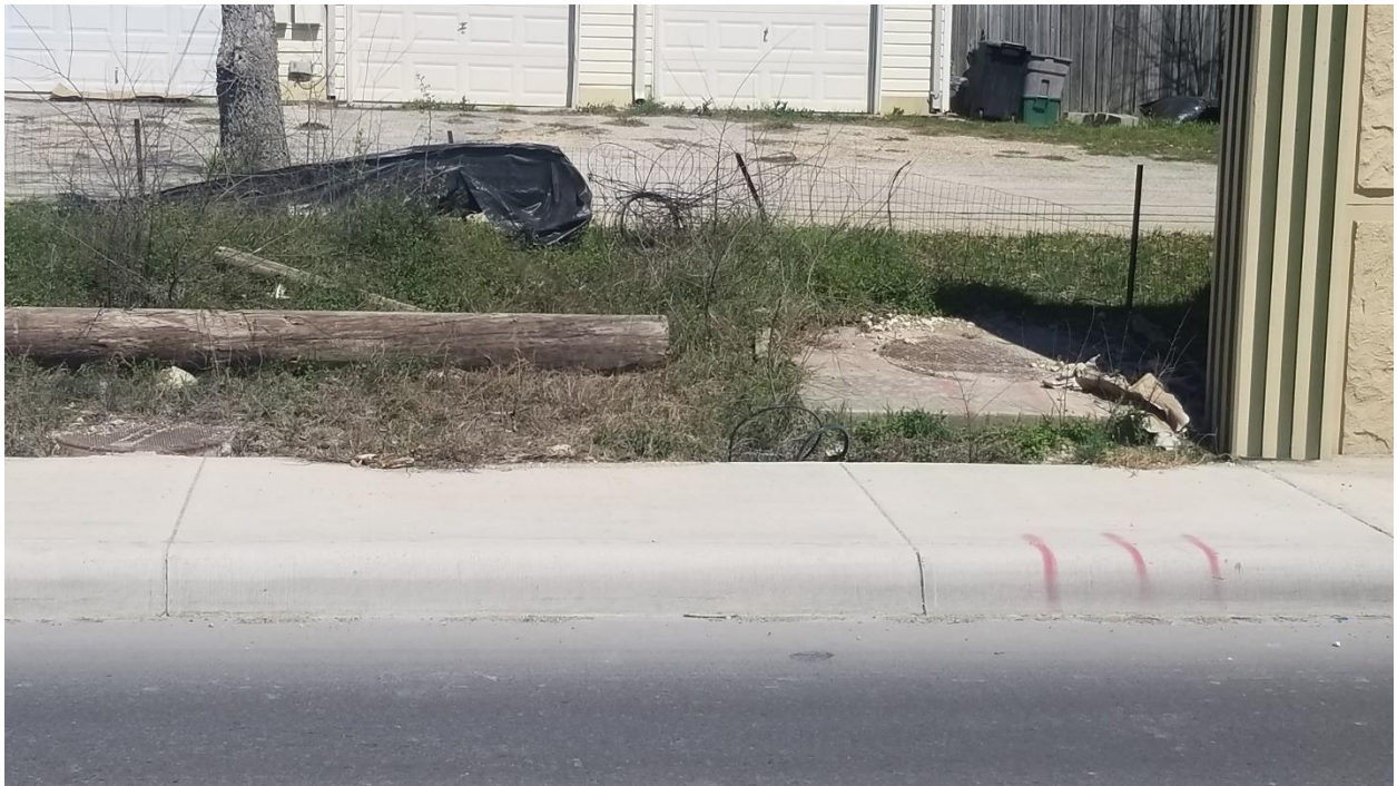
Figure 150. Manhole and Vault at North End of SWNB04.
