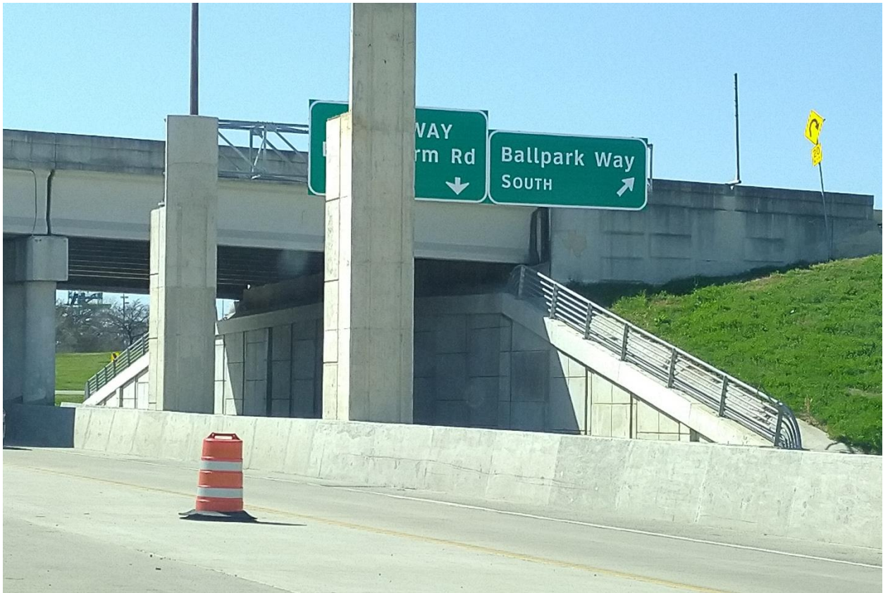
Figure 86. Retaining Wall B02B.
