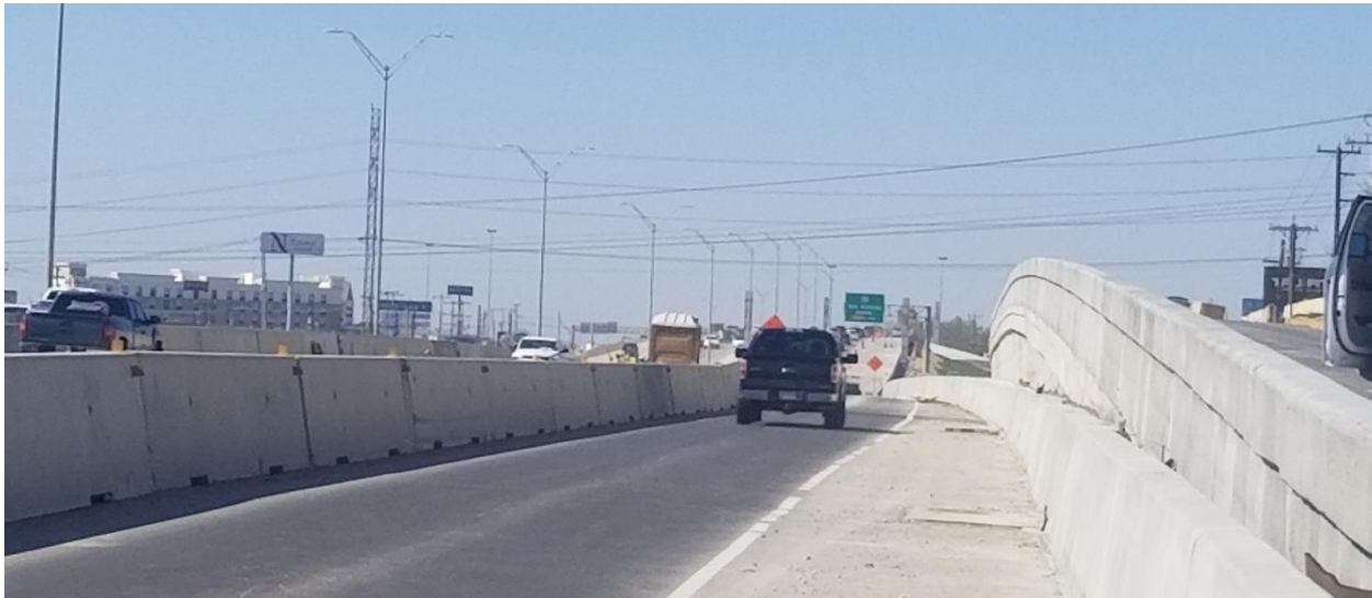
Figure 155. North-Facing View at South End of RWNB01.
