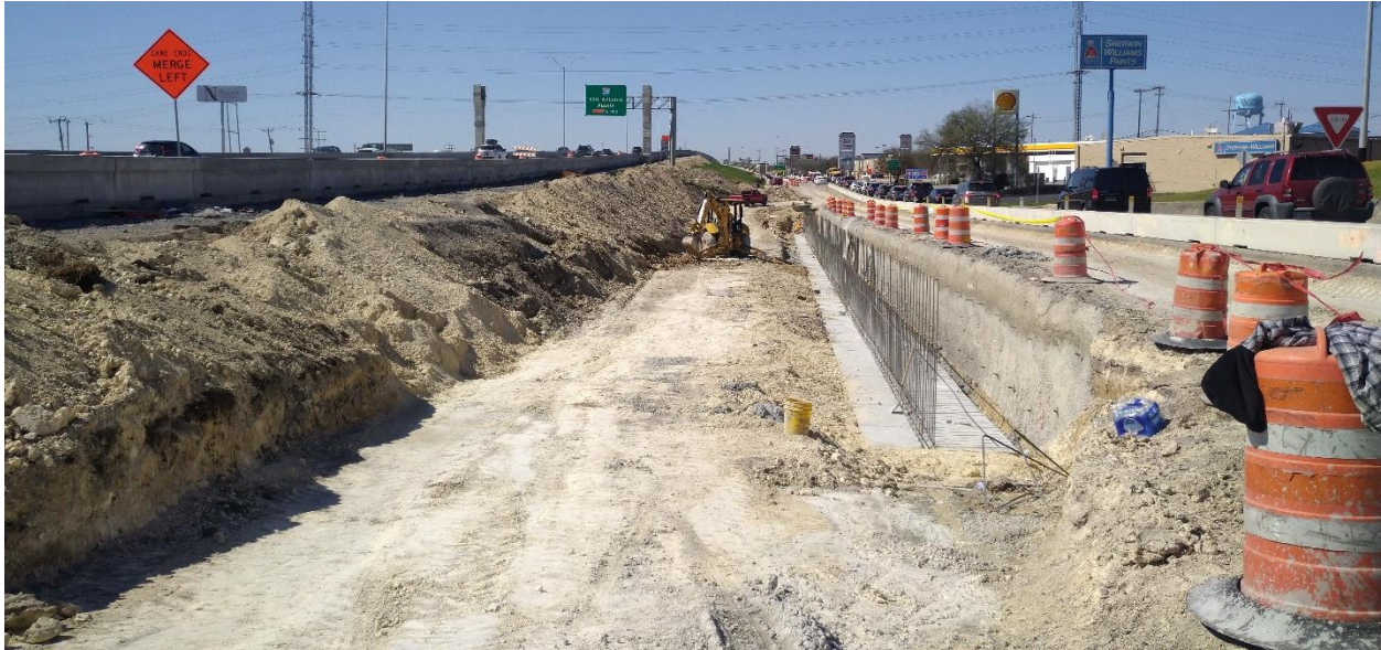
Figure 170. North-Facing View at South End of RWDET01.
