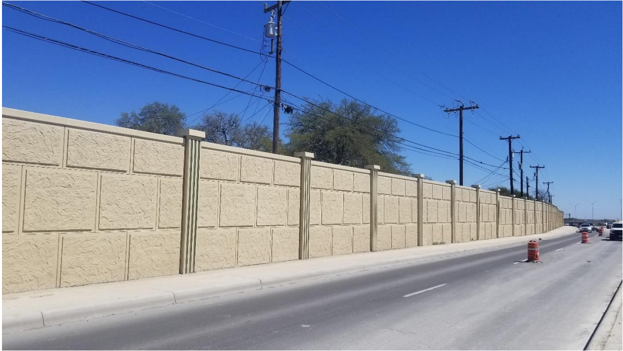
Figure 146. Noise Wall SWNB04.
