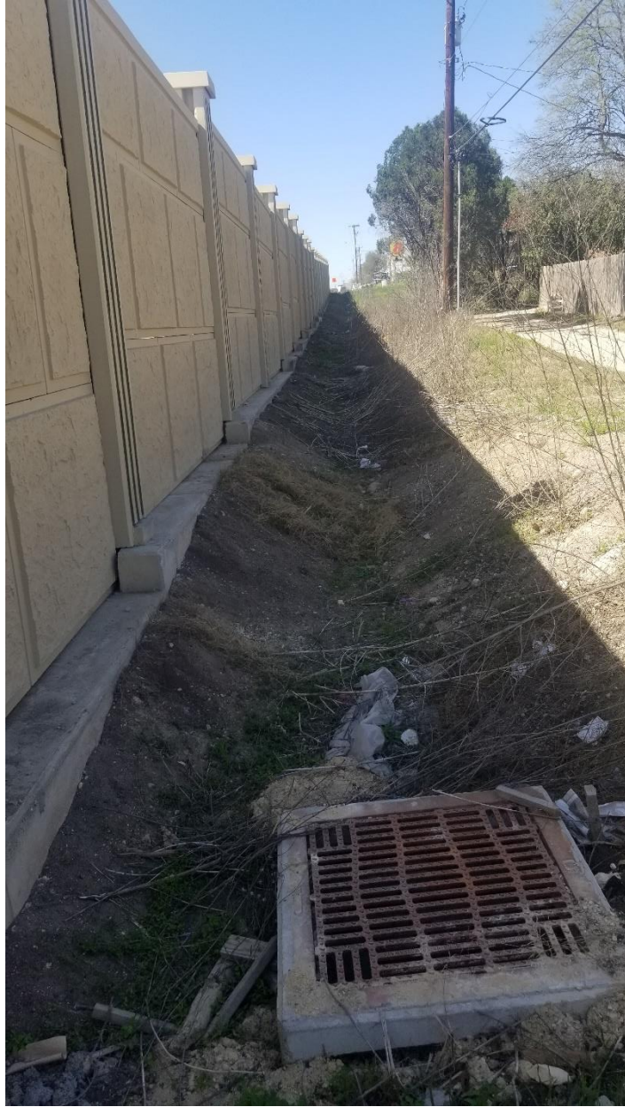
Figure 133. Drainage behind SWNB01.
