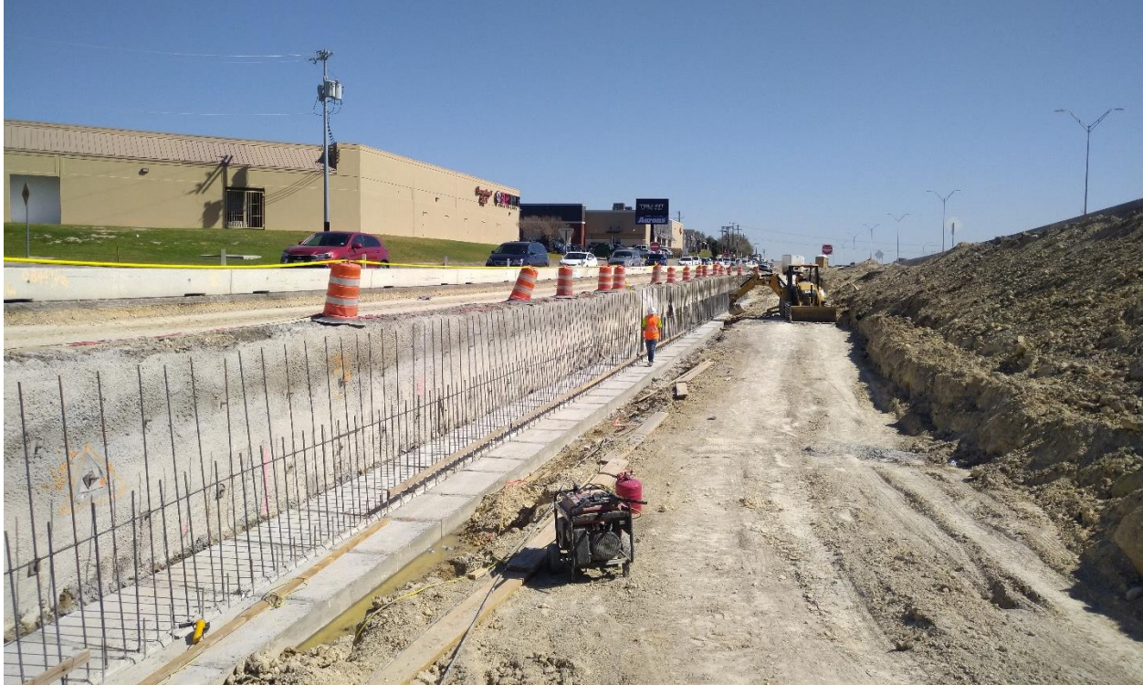
Figure 172. South-Facing View at North End of RWDET01.
