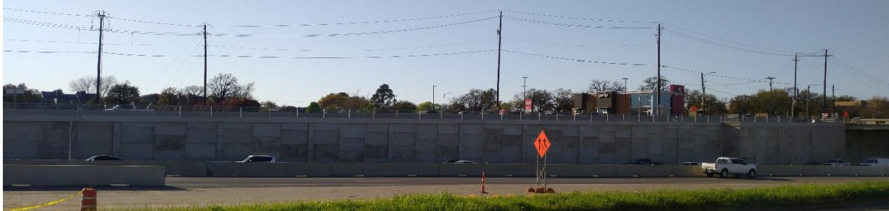
Figure 99. Retaining Wall B30C.
