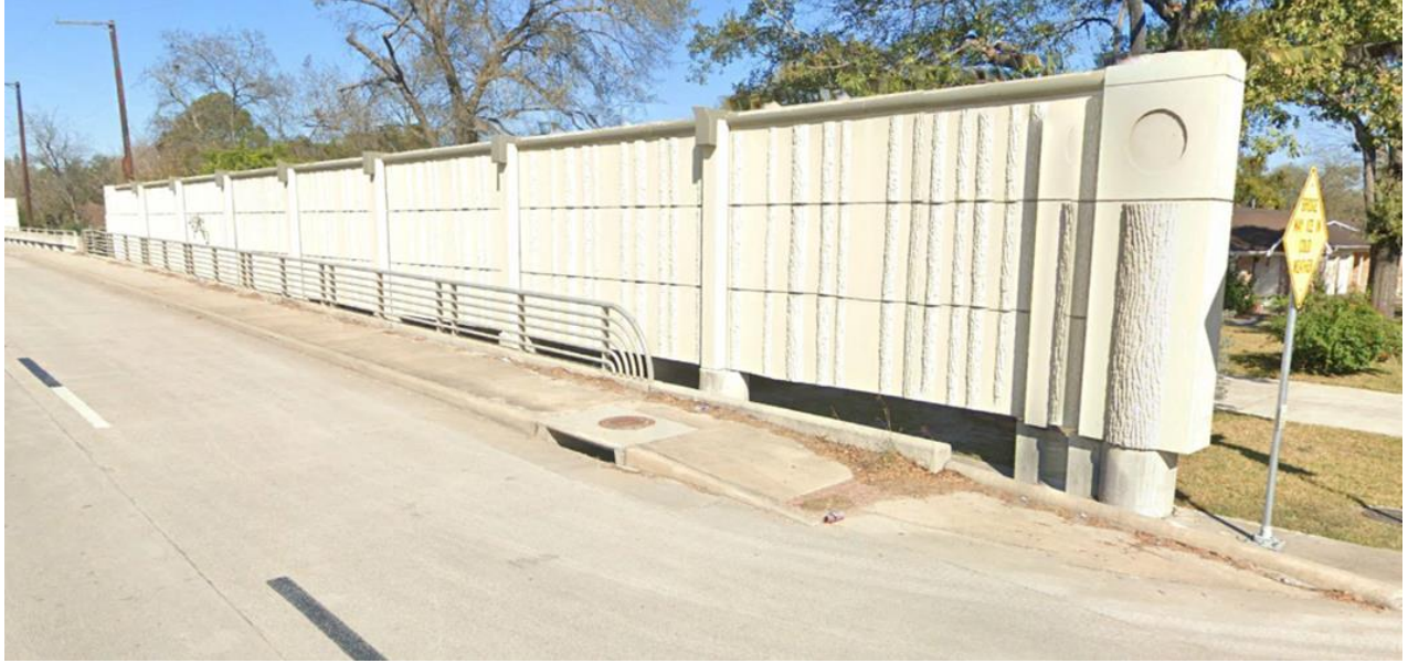
Figure 181. Noise Wall at Brickhouse Gully.
