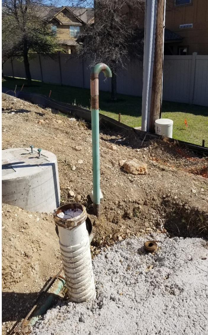
Figure 37. Relocated Gas Valve and Appurtenances at 1A Spread Footing.
