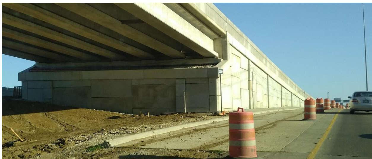
Figure 103. Retaining Wall B42B and B42C.
