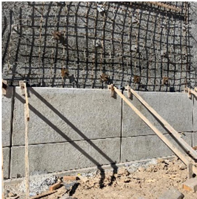
Figure 182. Metro Bus Lane Construction.
