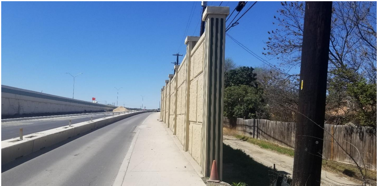
Figure 147. North-Facing View at South End of SWNB04.
