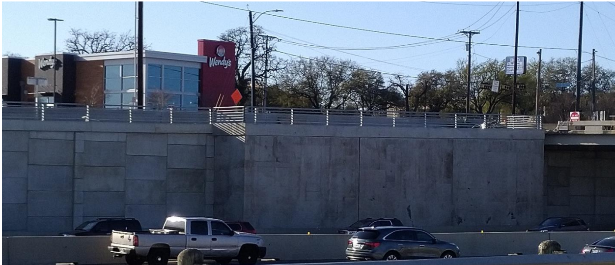
Figure 100. Retaining Wall B30C, Drilled Shaft Portion.
