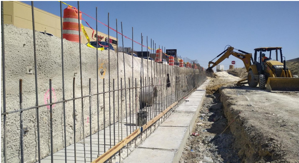
Figure 171. South-Facing View of RWDET01.
