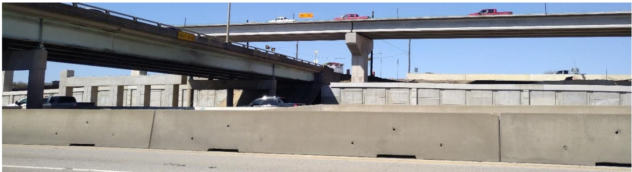
Figure 95. Retaining Wall B19.
