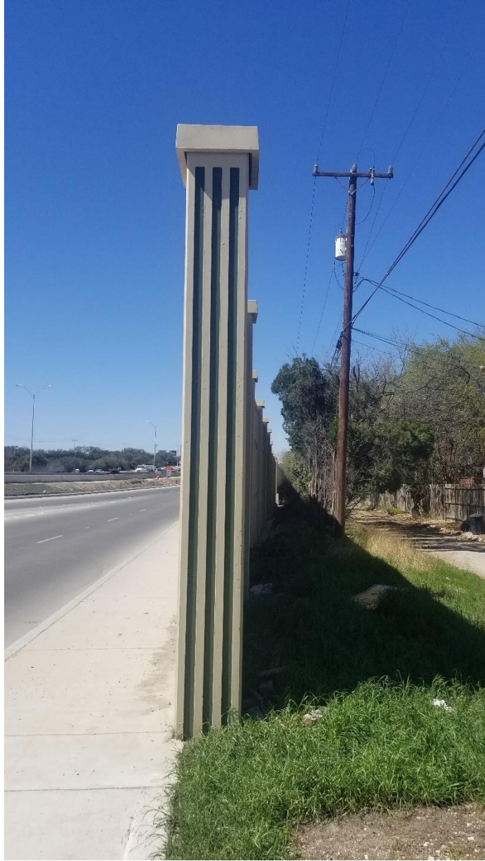
Figure 143. North-Facing View at South End of SWNB03.
