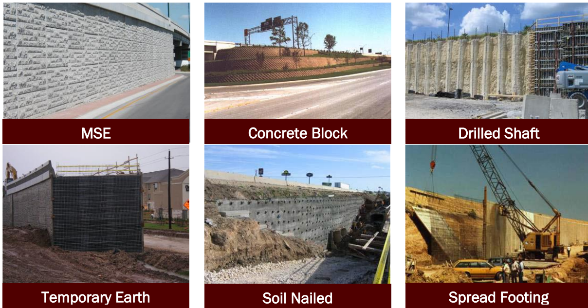
Figure 3. Types of Retaining Walls (15).
