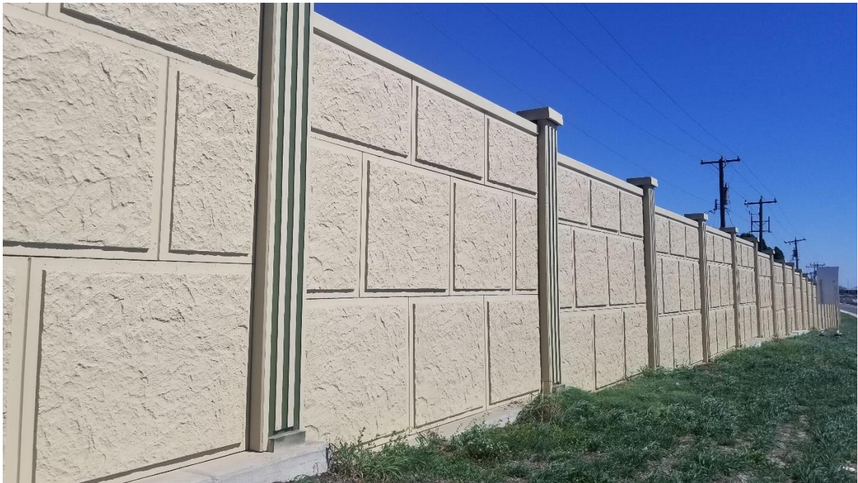
Figure 140. Noise Wall SWNB02.
