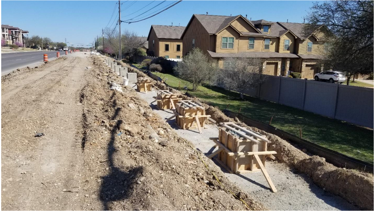
Figure 34. South End of Noise Wall 1A.
