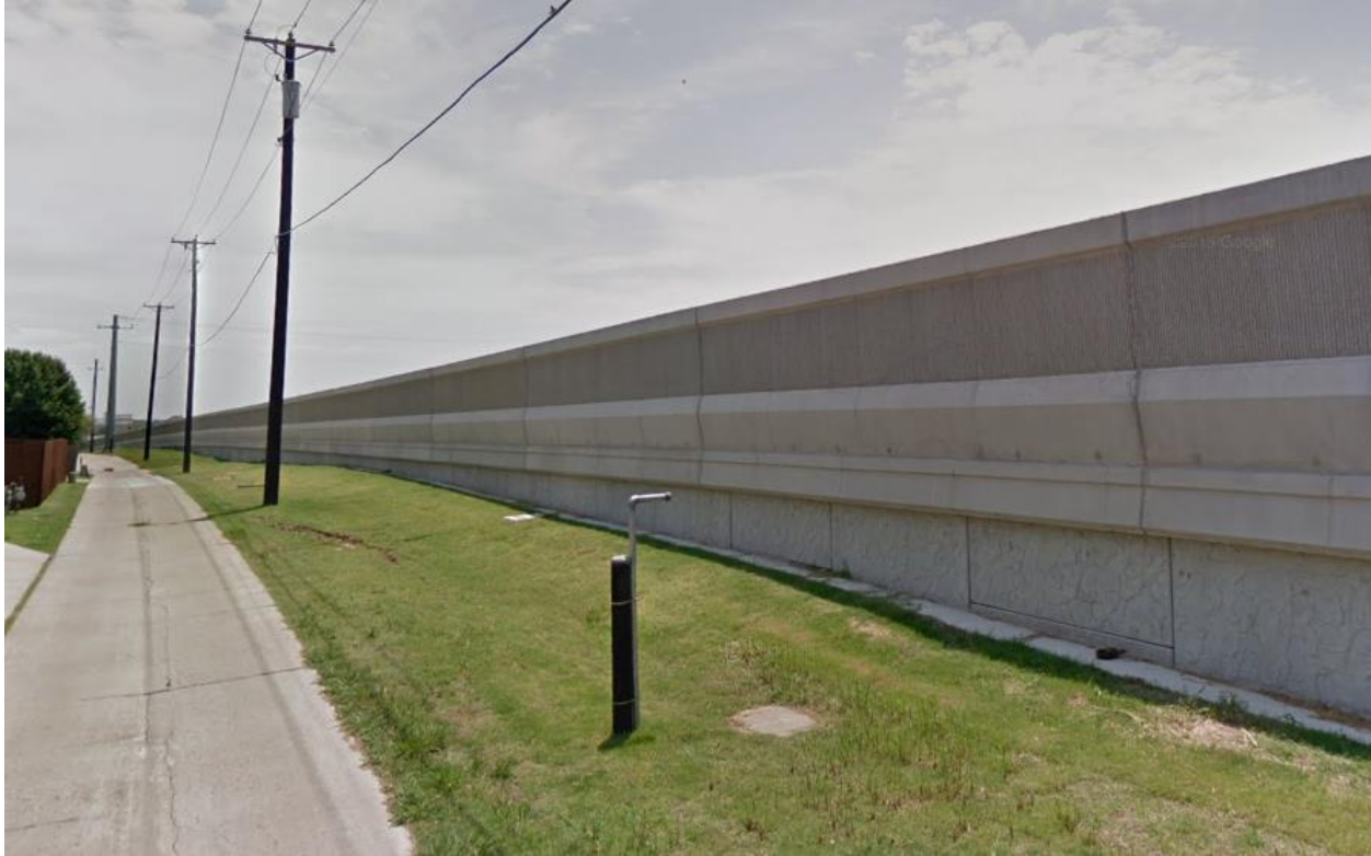
Figure 178. Noise Wall, President Bush Turnpike, Residents' Side, Before Construction.
