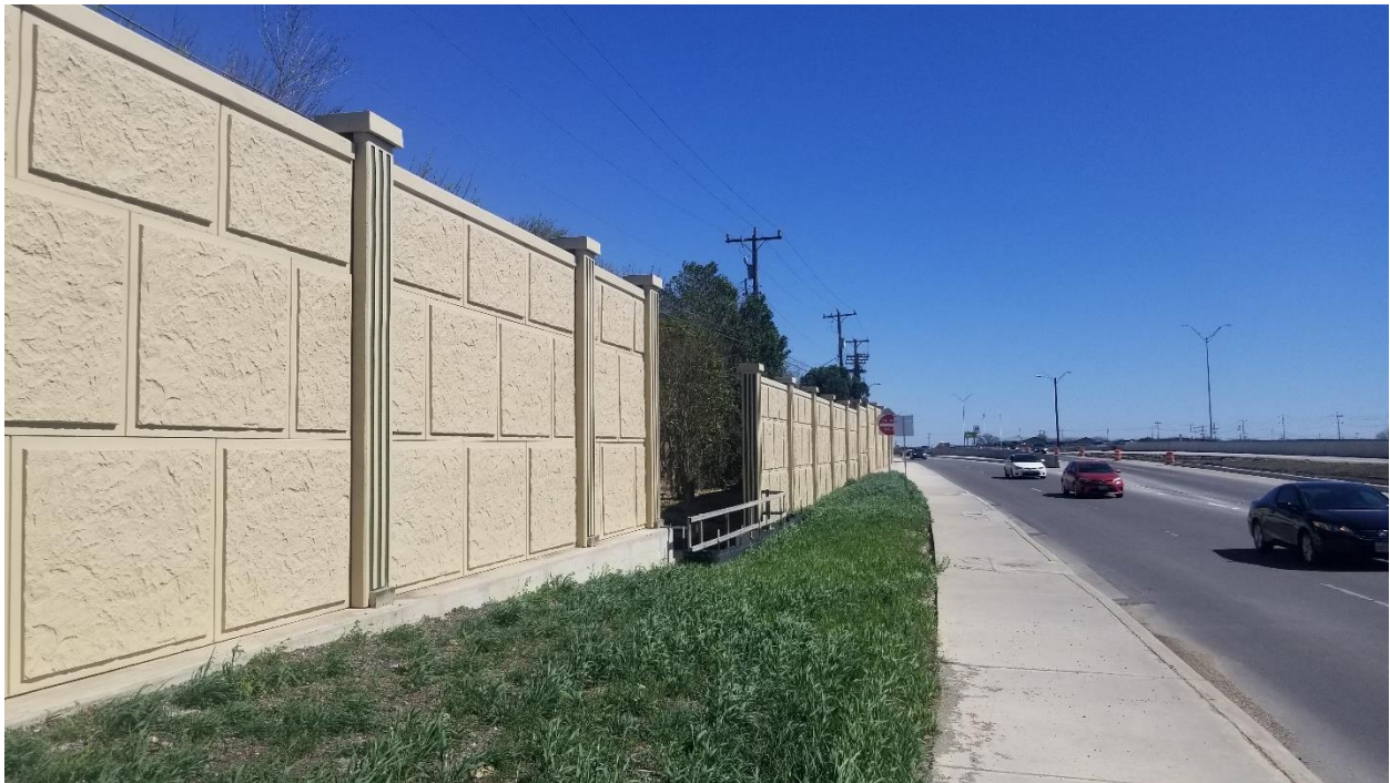
Figure 138. South-Facing View of South End of SWNB02 and North End of SWNB03.
