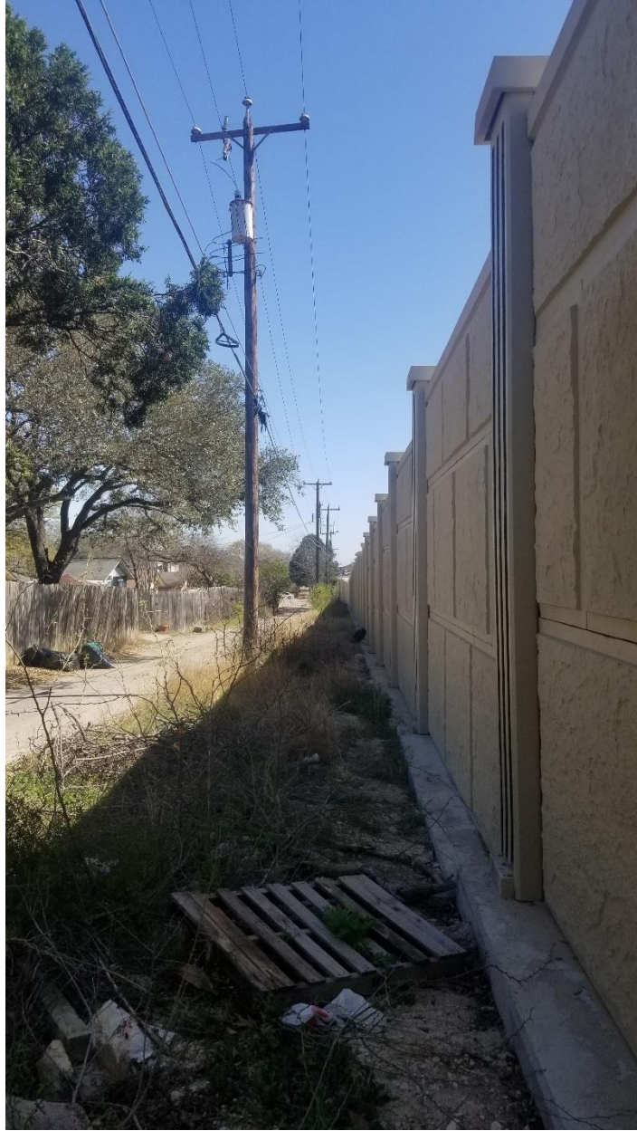
Figure 141. Receptor Side of SWNB02, South Facing.
