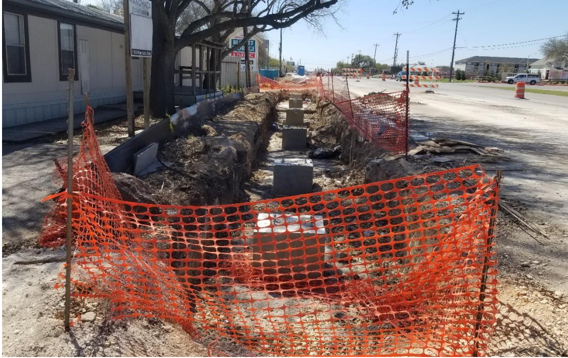
Figure 52. South-Facing View at North End of 3B.
