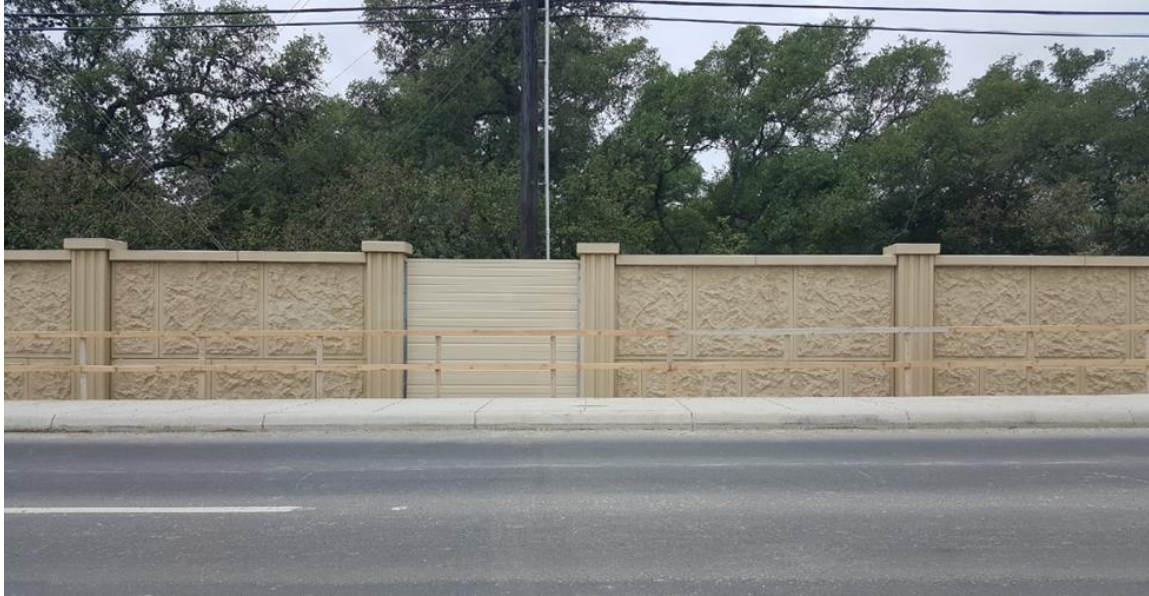
Figure 10. Utility Pole Access Panel in Noise Wall on TxDOT Project 1 .
