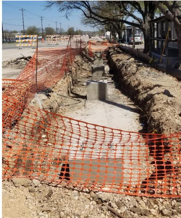
Figure 53. North-Facing View at South End of 3B.
