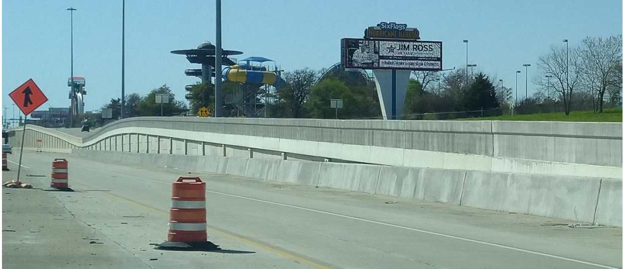
Figure 85. Retaining Wall B01.
