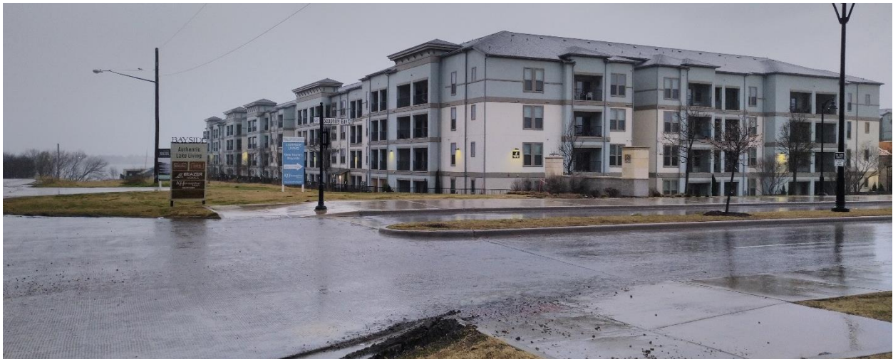
Figure 73. West View of Proposed AK Location.
