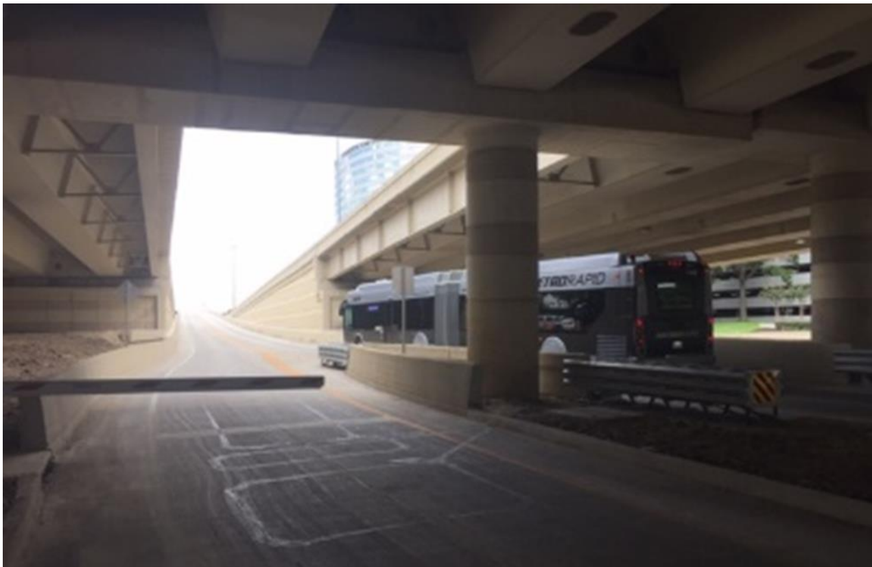
Figure 184. Completed Metro Bus Lane at IH 610 at Post Oak, View B.
