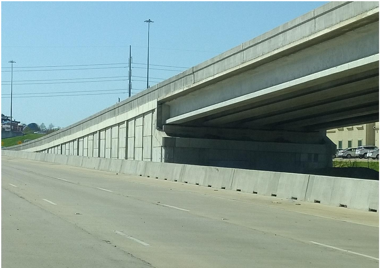
Figure 88. Retaining Wall B06B and B06C.
