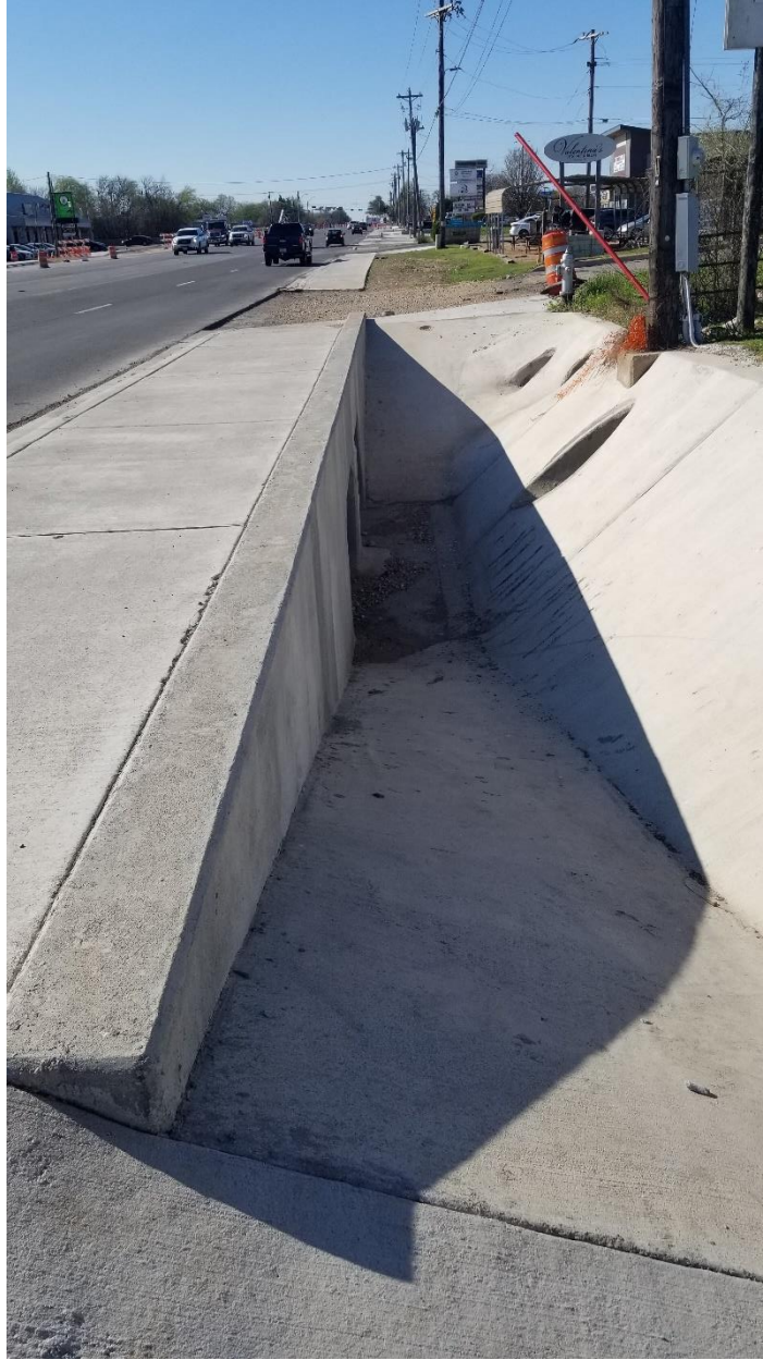
Figure 54. Headwall on Southbound Side.
