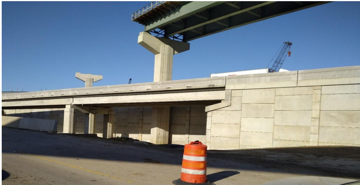
Figure 102. Retaining Wall B36A and B36C.
