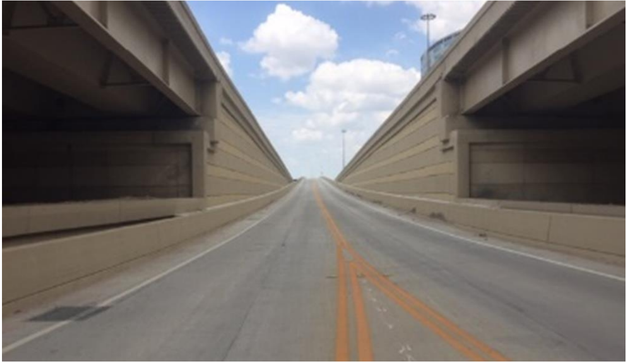
Figure 183. Completed Metro Bus Lane at IH 610 at Post Oak, View A.
