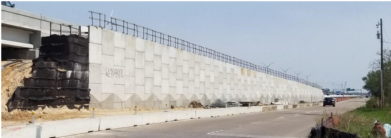
Figure 120. South-Facing View of RW 12.
