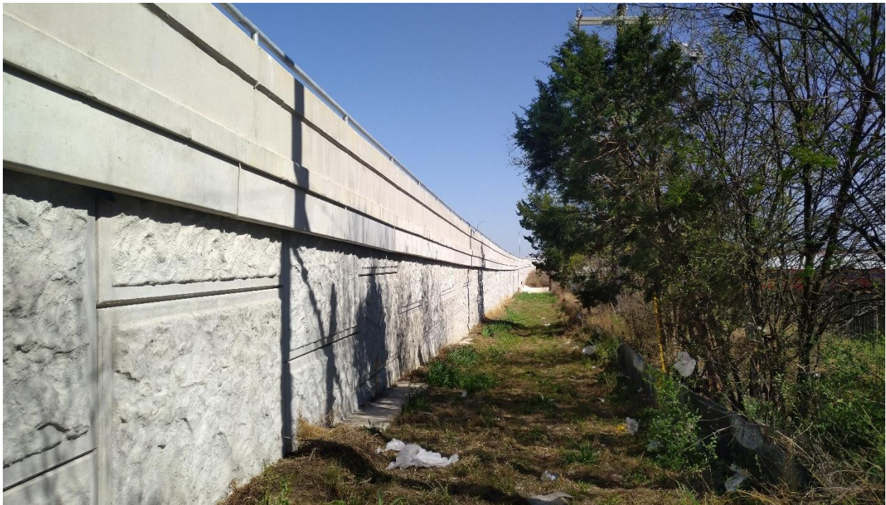
Figure 168. South-Facing View of RWSB02.
