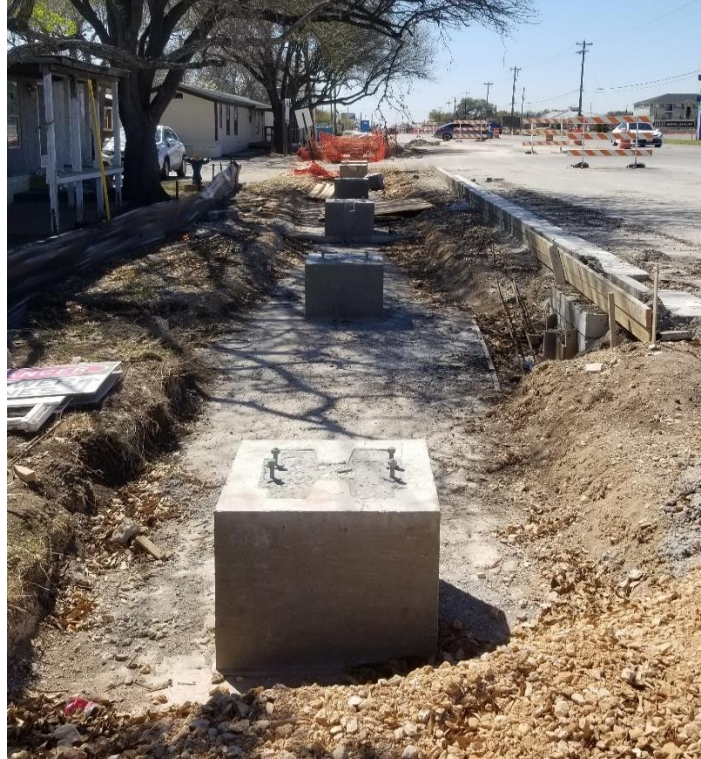
Figure 50. South-Facing View at North End of 3A.
