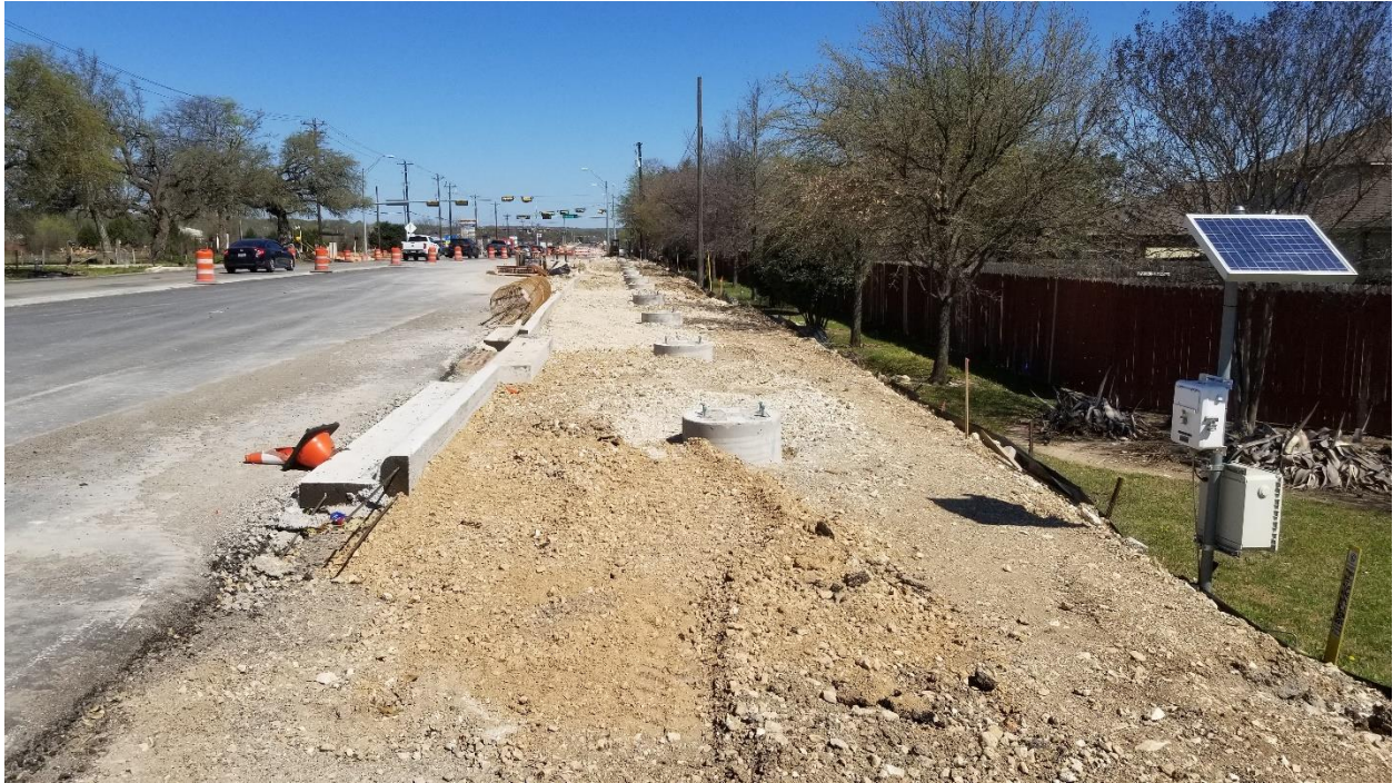
Figure 47. North-Facing View at South End of 2B.
