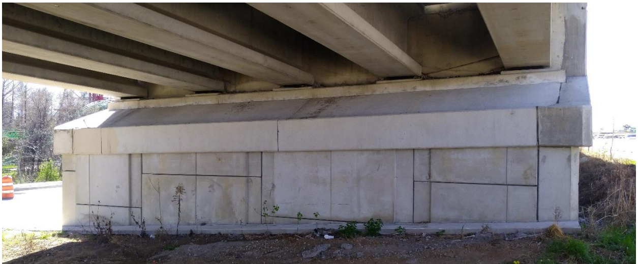
Figure 92. Retaining Wall B08B.
