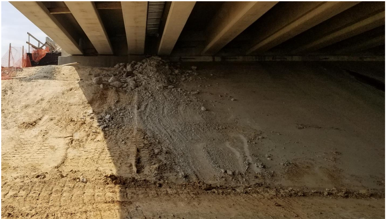
Figure 116. Southbound Side of RW 9.
