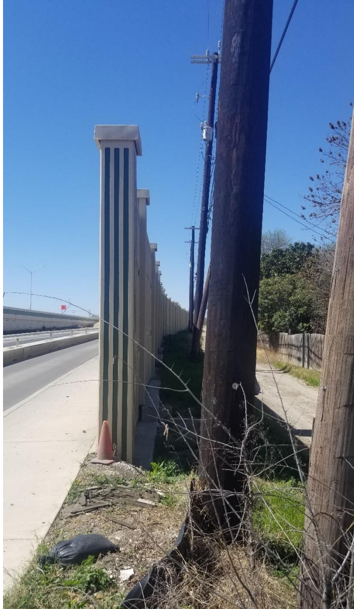
Figure 148. North-Facing View at South End of SWNB04, Receptor Side.
