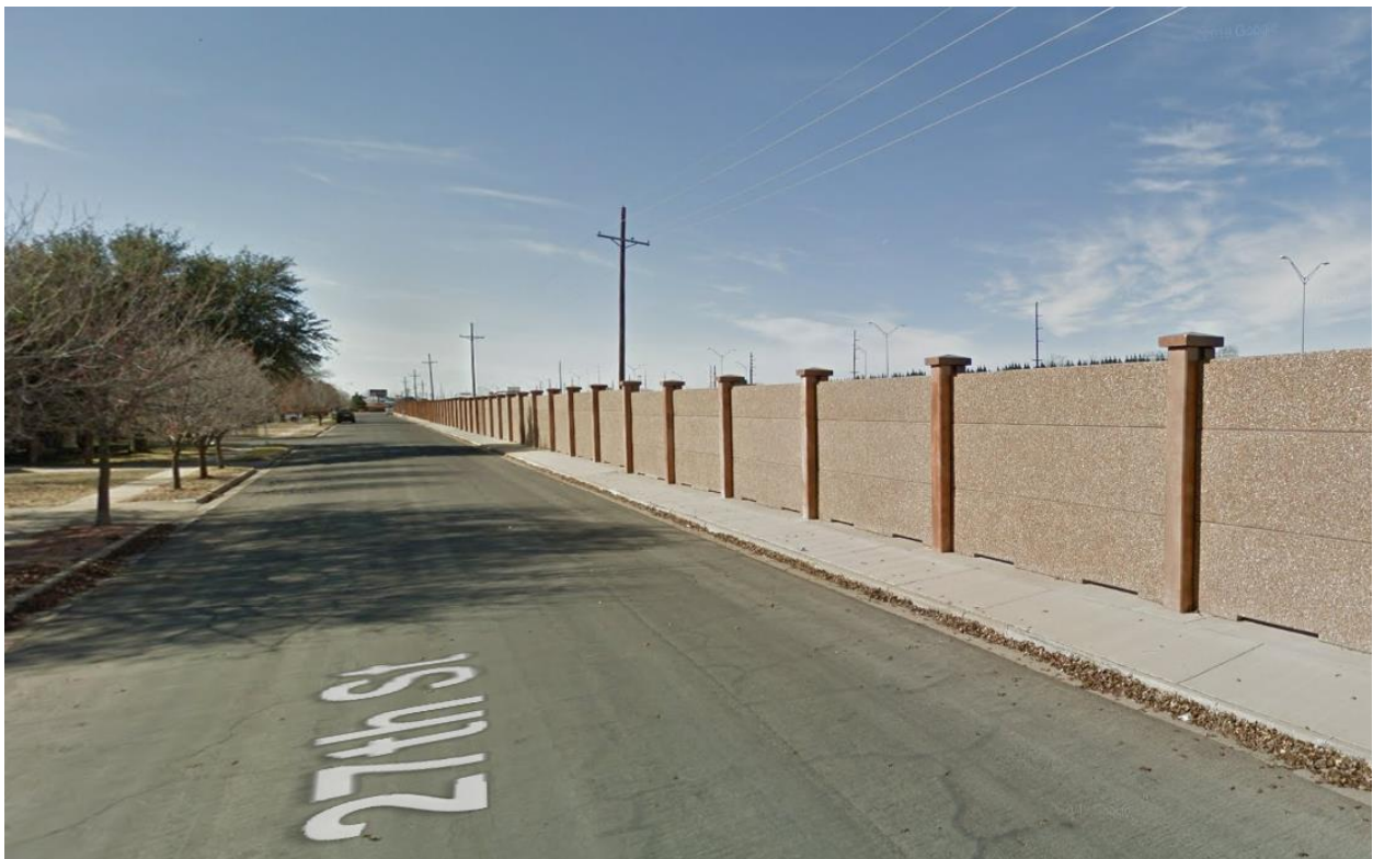
Figure 175. Noise Wall on Marsha Sharp Freeway in Lubbock, Residents' Side.
