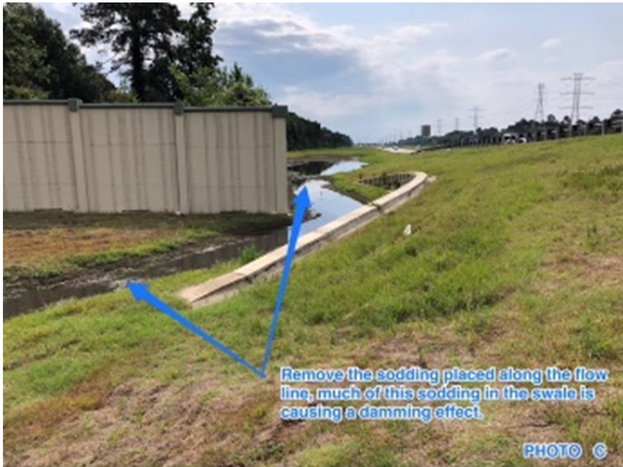
Figure 179. Mossy Oak Retaining Wall and Noise Wall.
