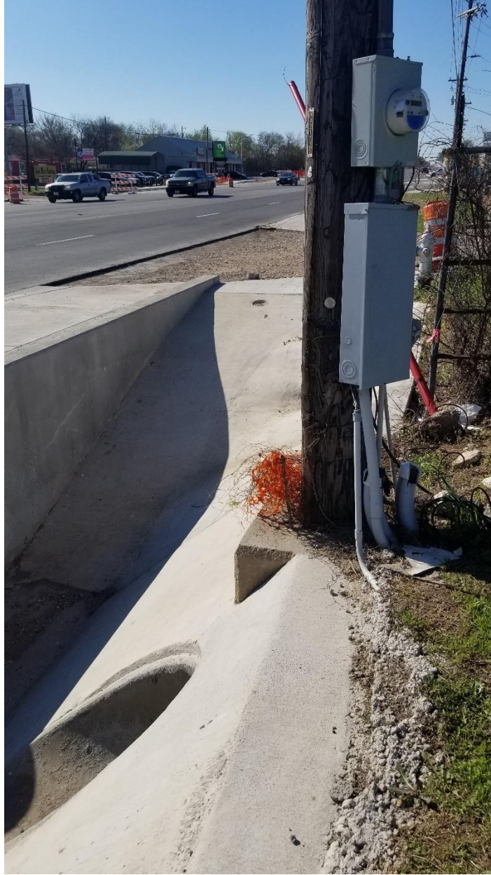
Figure 56. Close-Up of Utility Pole Adjacent to Southbound Headwall.
