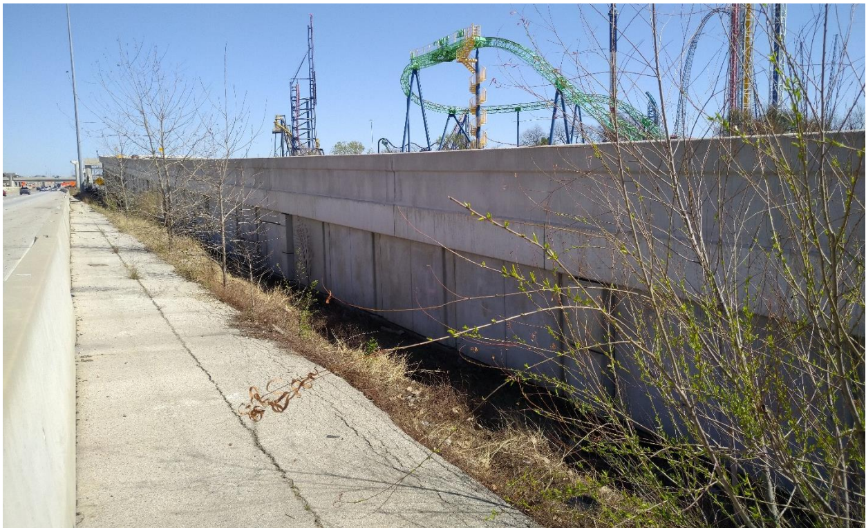
Figure 90. Retaining Wall B08A.
