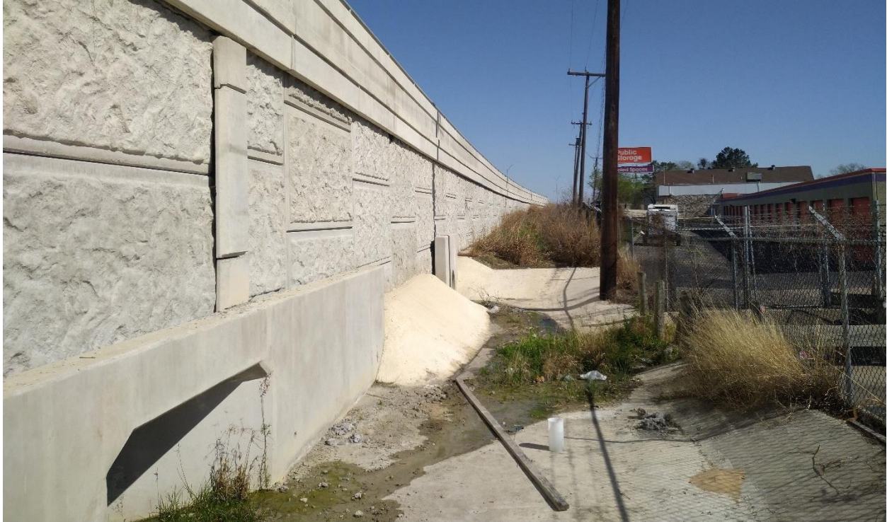
Figure 167. Drainage at Face of RWSB02.
