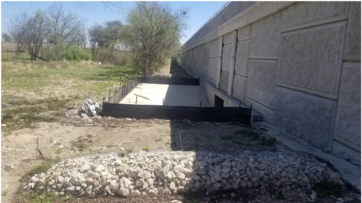
Figure 160. Box Culvert at RWNB02.
