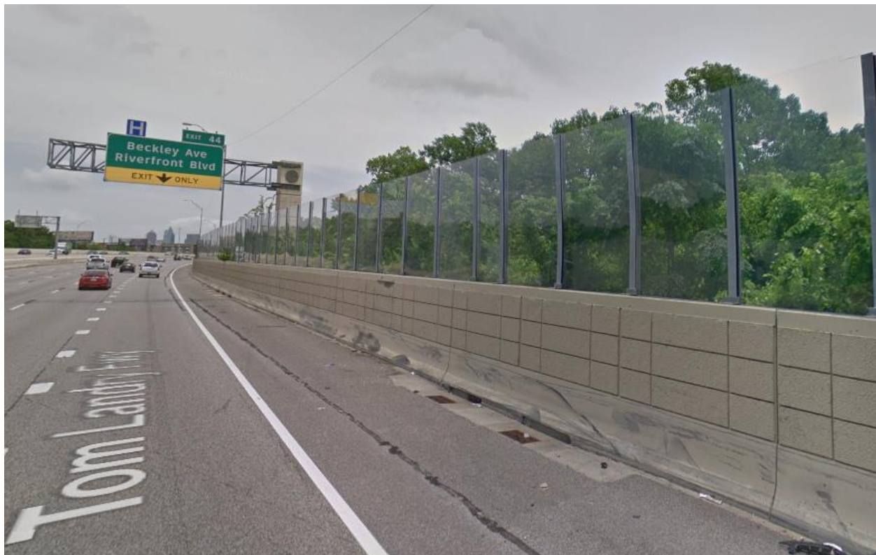
Figure 176. Noise Wall on I-30 in Central Dallas.
