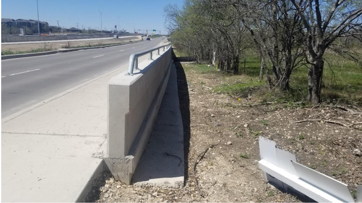
Figure 158. North-Facing View at South End of RWNB02.
