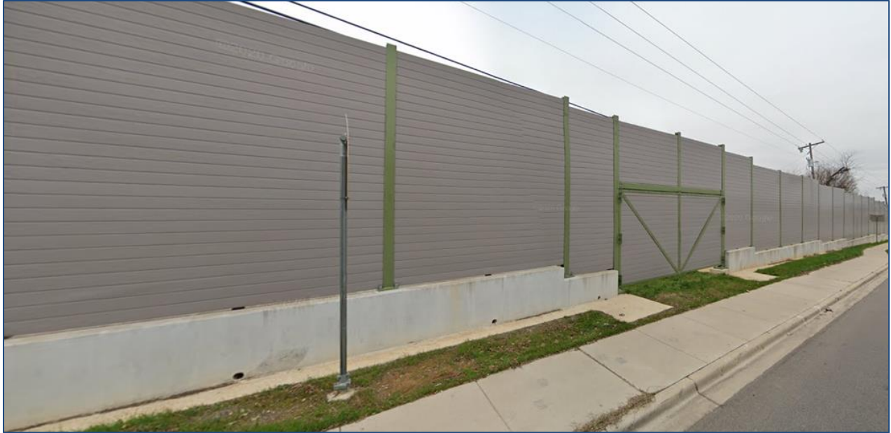
Figure 30. Plastic Noise Wall with Access Gate (Source: Google Street View).
