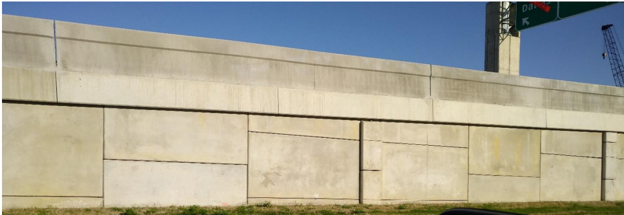
Figure 97. Retaining Wall B25.
