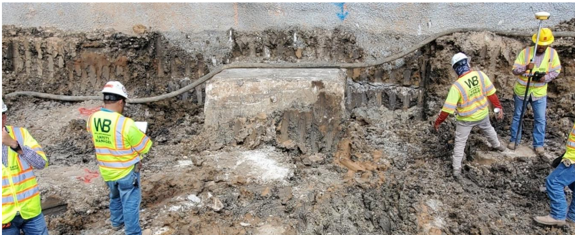
Figure 123. Existing Culvert at RW 12.
