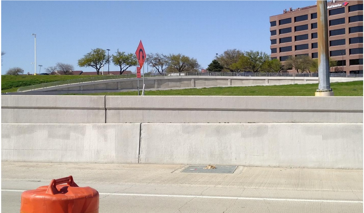
Figure 87. Retaining Wall B03.
