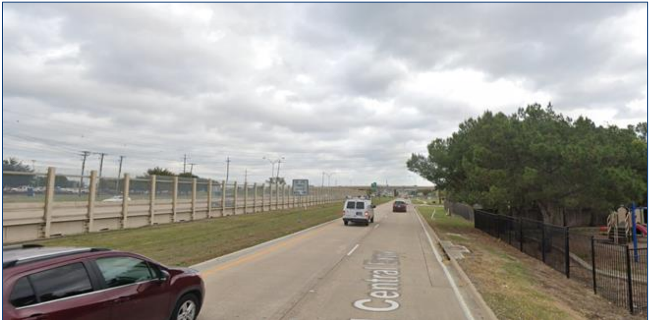
Figure 26. Transparent Noise Wall Located between Frontage Road and Main Lanes (Source: Google Street View).
