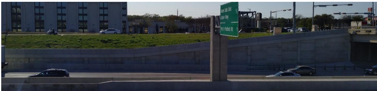
Figure 98. Retaining Wall B30A.
