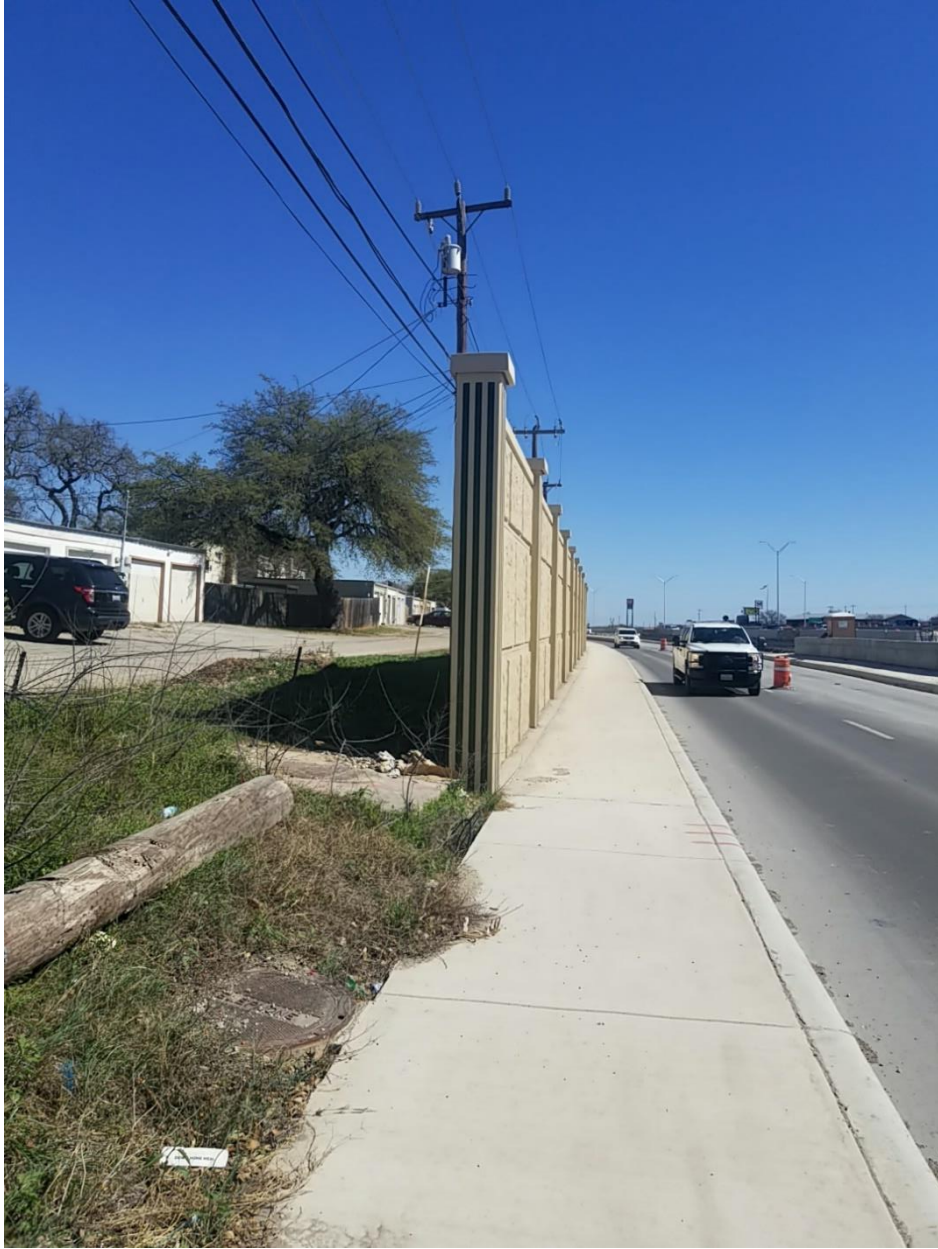
Figure 151. Manhole and Vault at North End of SWNB04, South Facing.
