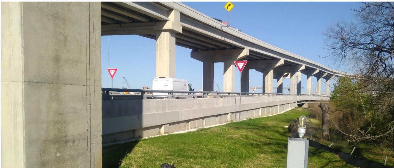
Figure 94. Retaining Wall B10A.
