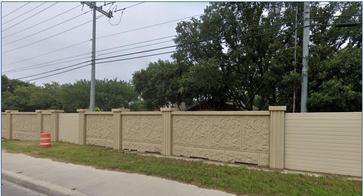
Figure 29. Fiberglass Noise Wall Panels (Source: Google Street View).
