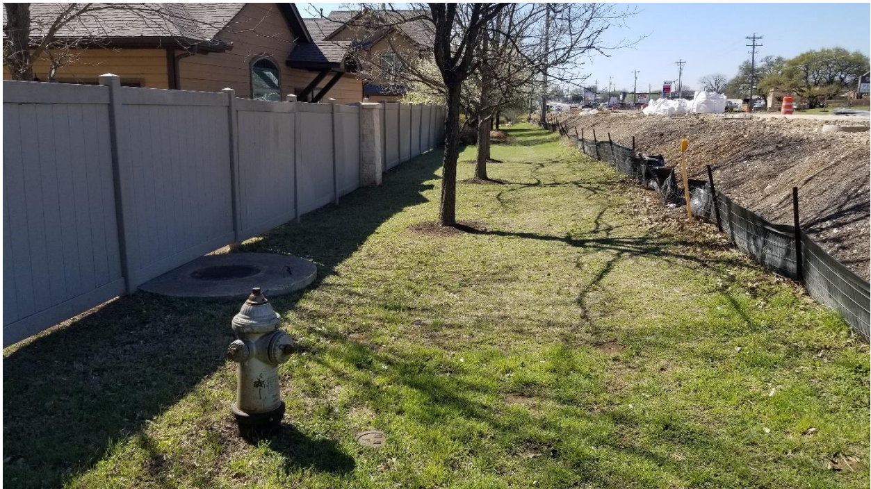
Figure 39. Existing Fire Hydrant behind 1A.
