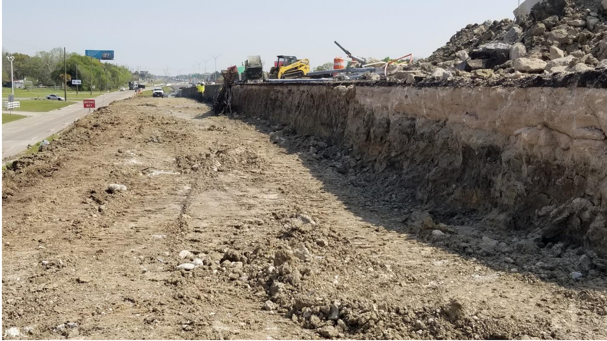
Figure 119. South-Facing View of RW 11.
