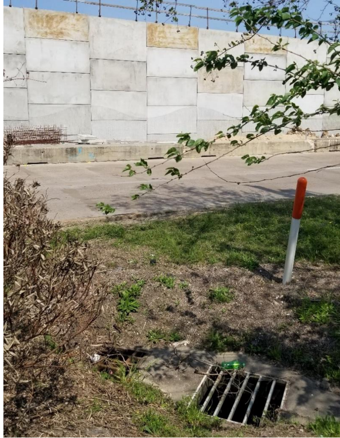
Figure 124. East-Facing View of Drainage at RW 12.
