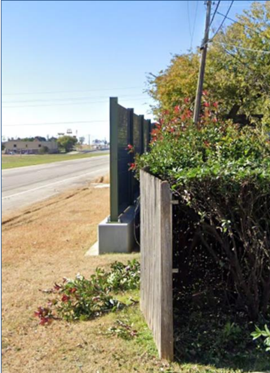
Figure 24. Plastic Noise Wall Installed near Right-of-Way Line (Source: Google Street View).
