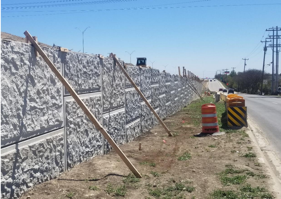
Figure 164. Temporary Construction Bracing at Face of RWSB01.
