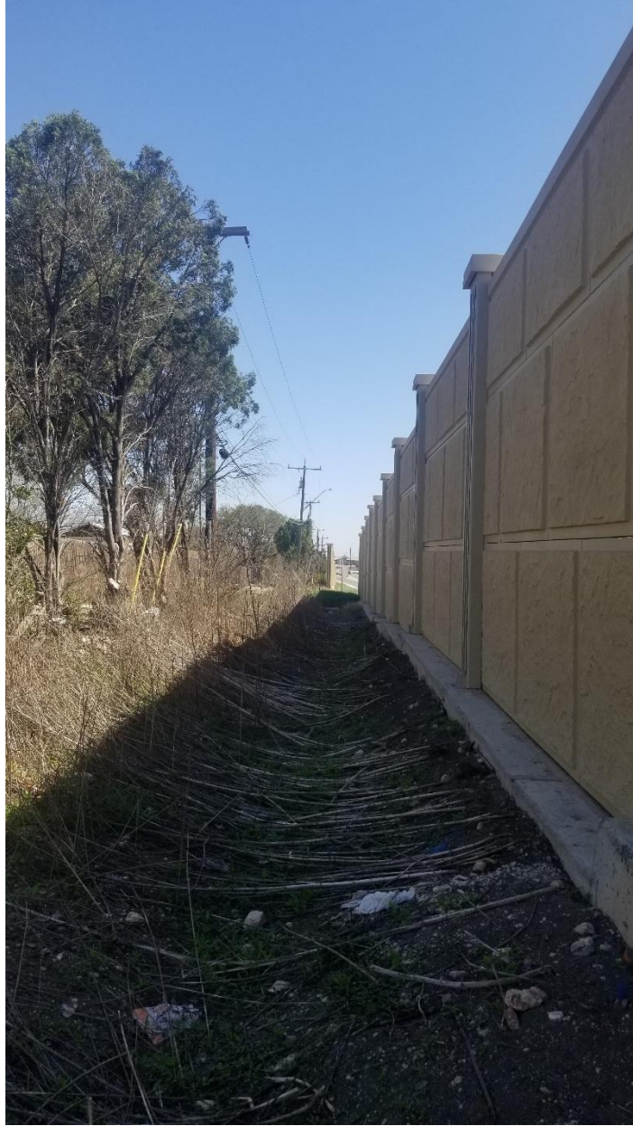
Figure 136. Receptor Side of SWNB01, South Facing.
