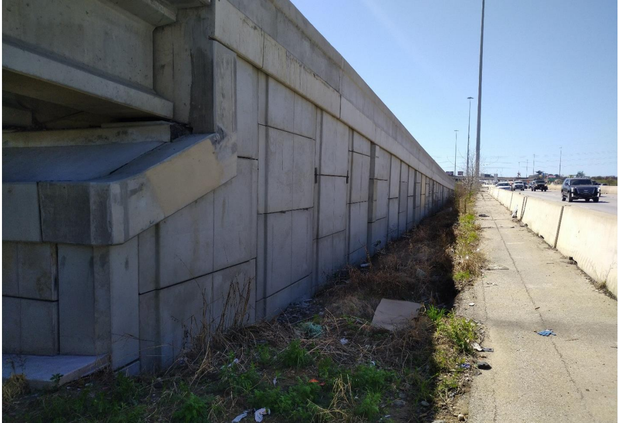
Figure 91. West-Facing View at East Side of B08A.
