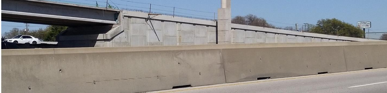
Figure 96. North-Facing View of Retaining Wall B21B and B21C.
