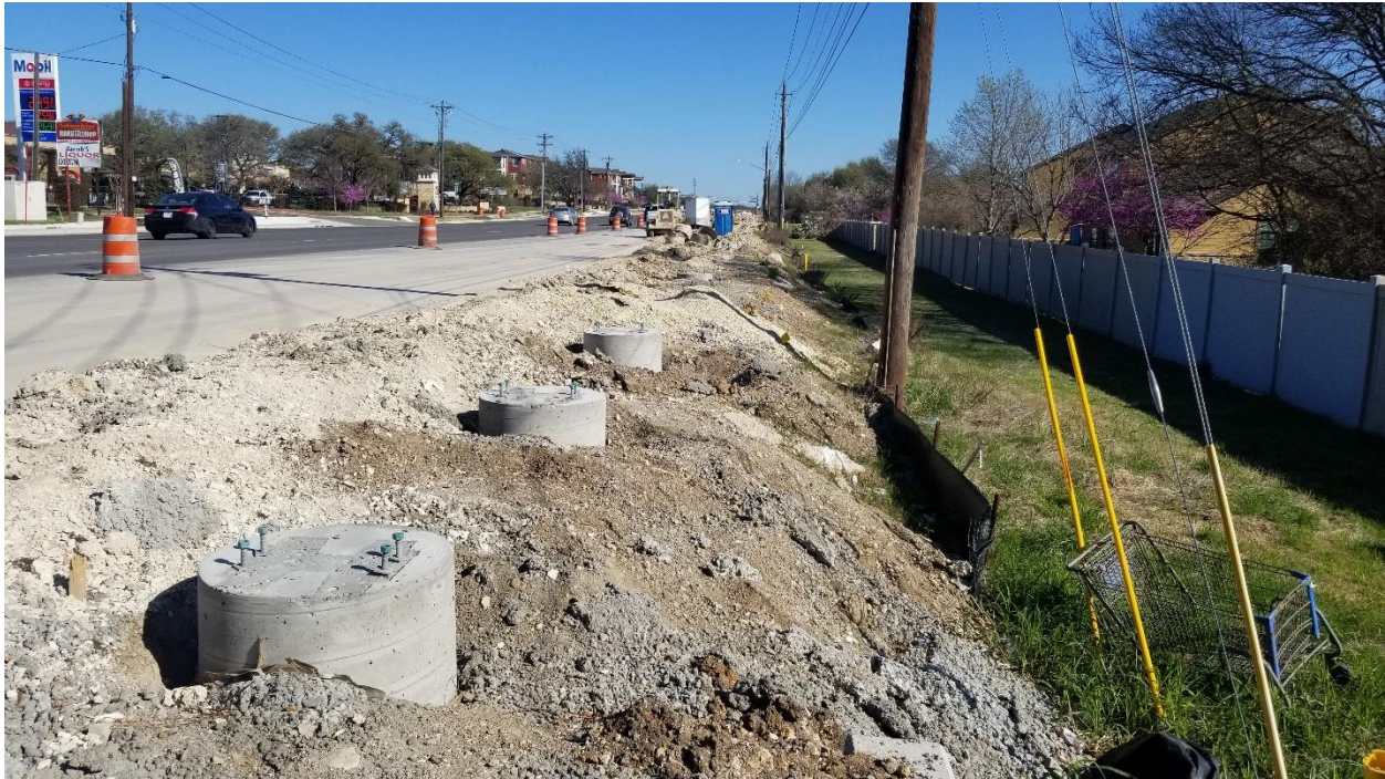
Figure 40. North-Facing View at South End of 1B.
