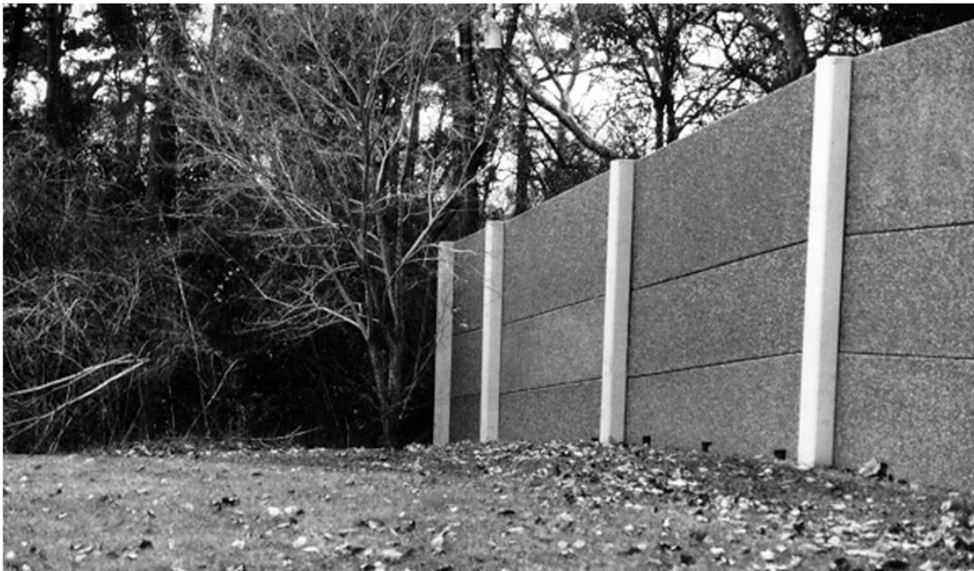
Figure 5. Example of Post-and-Panel System Using Concrete Posts (4).
