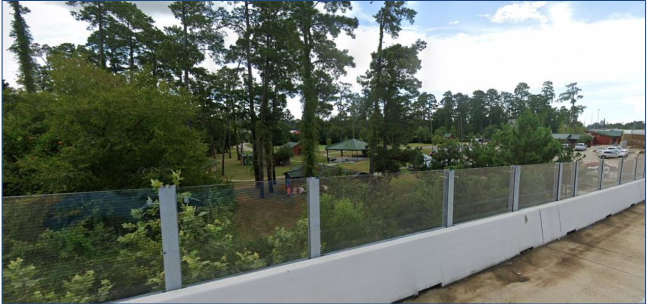
Figure 28. Transparent Noise Wall (Source: Google Street View).
