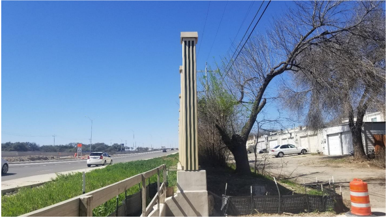
Figure 137. North-Facing View at South End of SWNB02.
