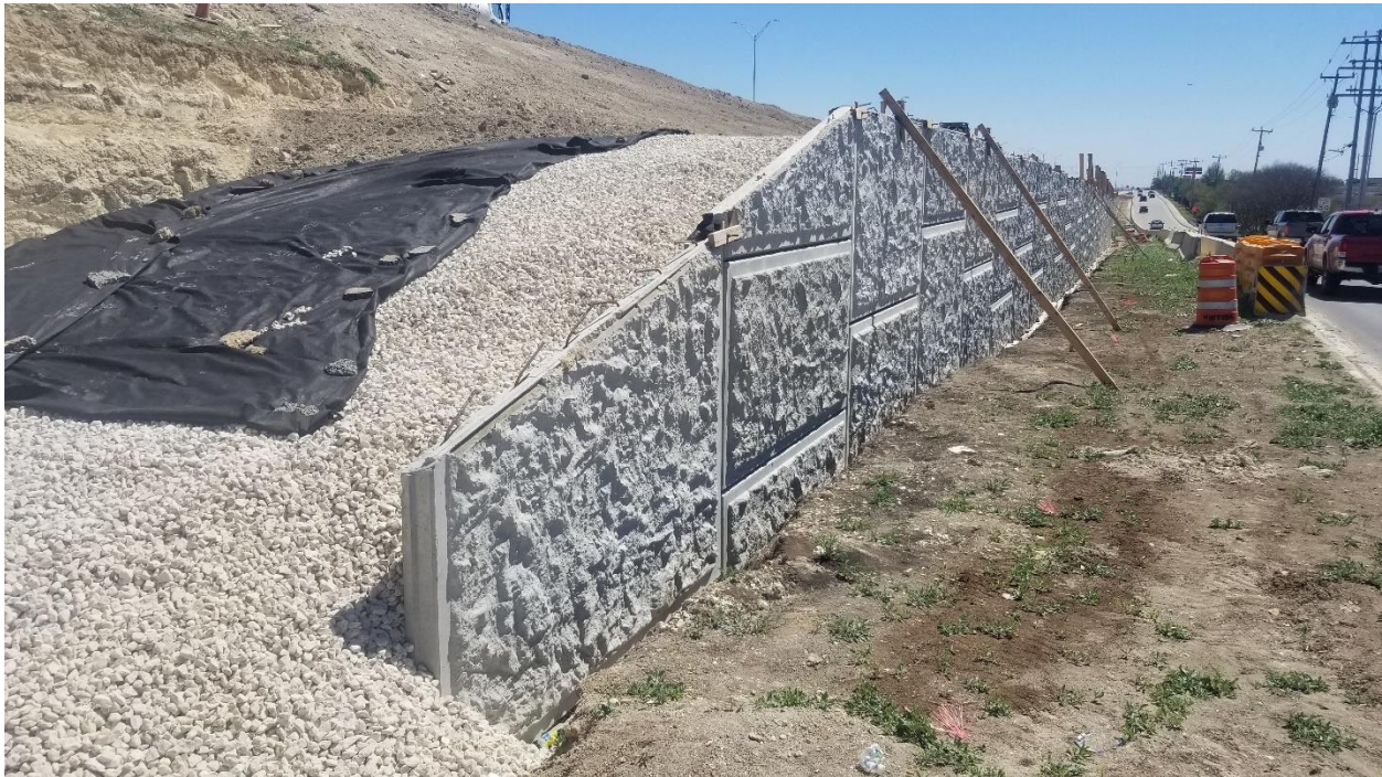
Figure 163. South-Facing View at North End of RWSB01.
