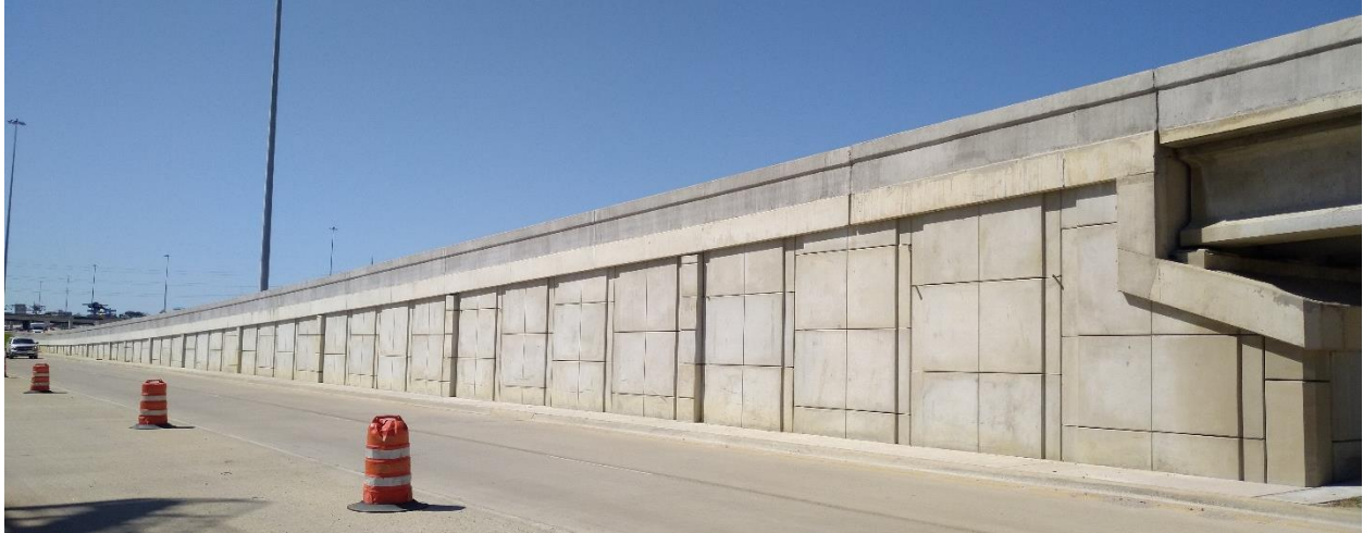
Figure 93. Retaining Wall B08C.
