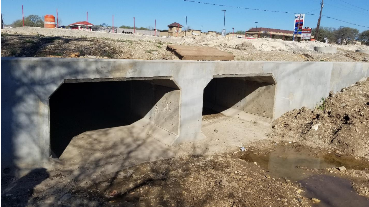
Figure 58. Headwall on Northbound Side.
