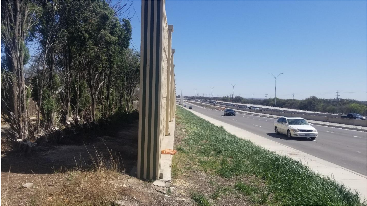
Figure 139. South-Facing View at North End of SWNB02.
