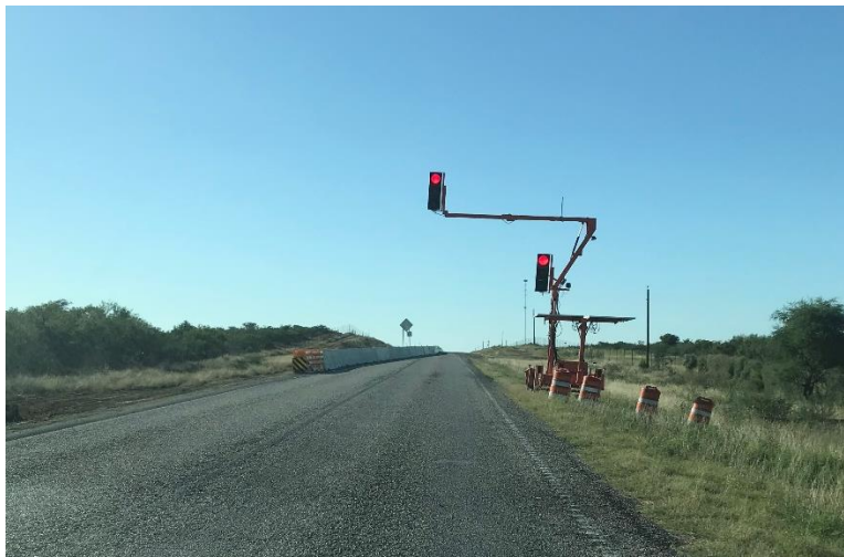
Figure 19. PTS Deployed in TxDOT Construction Work Zone.
