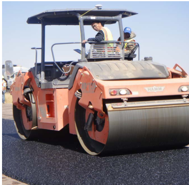
Figure 5-14. Compaction of the SMA.
