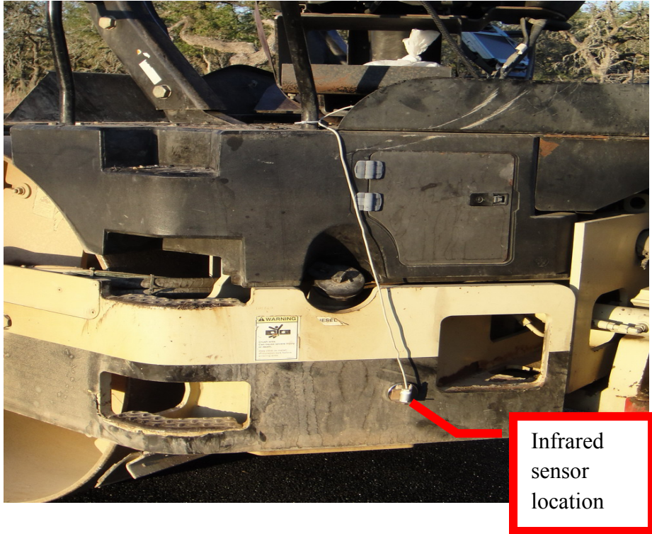
Figure 5. Infrared Sensor Installation.
