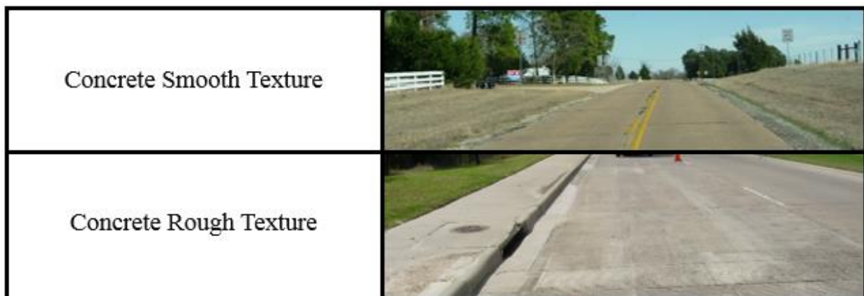
Figure 5: Pavement Condition—Concrete Pavement
