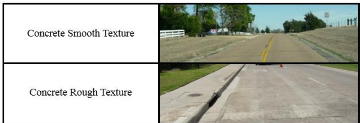
Figure 2: Pavement Condition—Concrete Pavement
