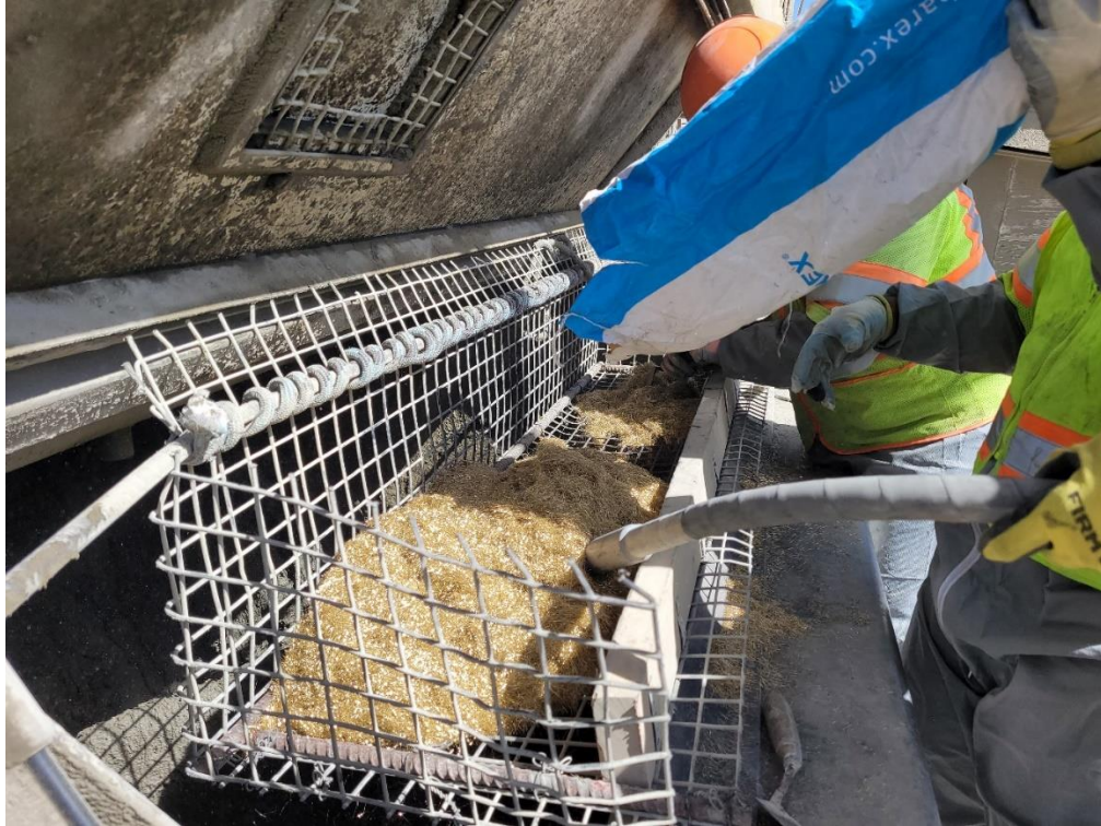
Figure 2.4. Screen and Vibrator used for Fiber Addition.
