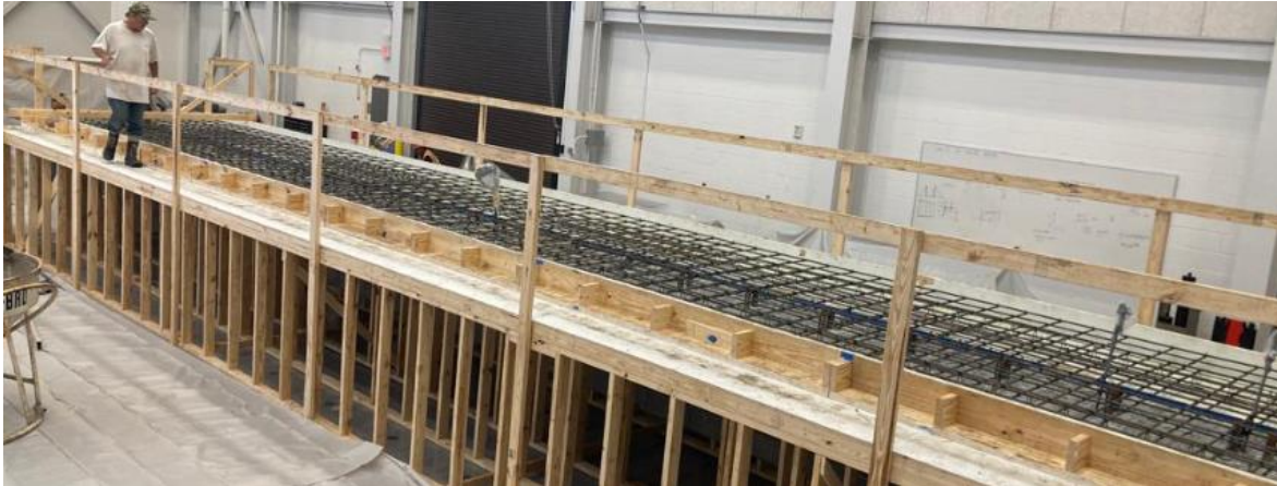
Tx34-1 Deck Formwork and Reinforcement Mesh
