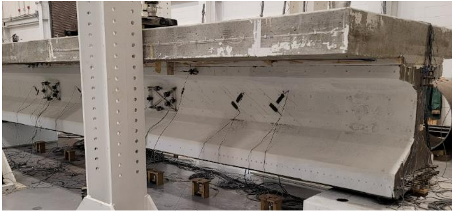
(a) North Face with LVDT and SG (Reinforced West End)
