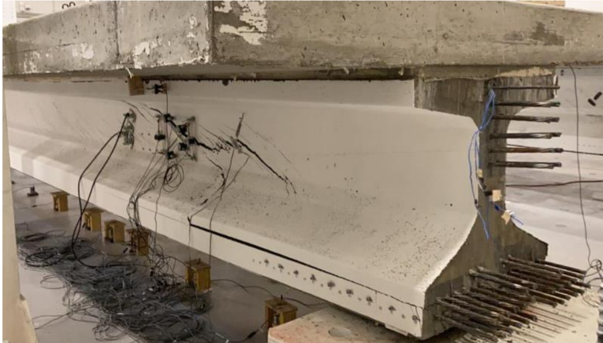
(a) Unreinforced End of Tx34-2 after Shear Failure
