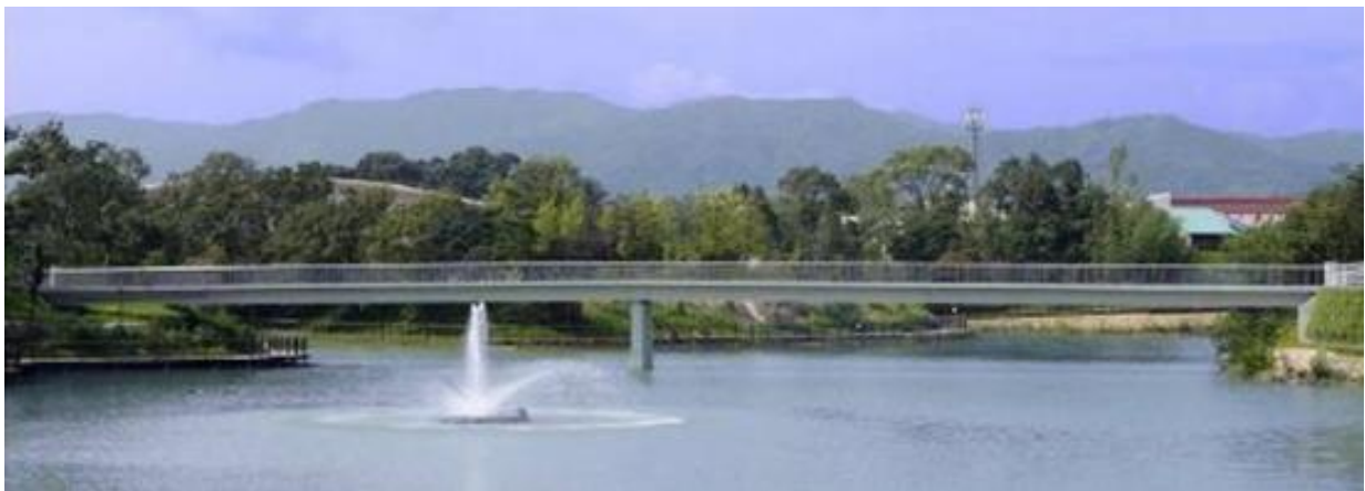
(e) Mikaneike Footbridge
