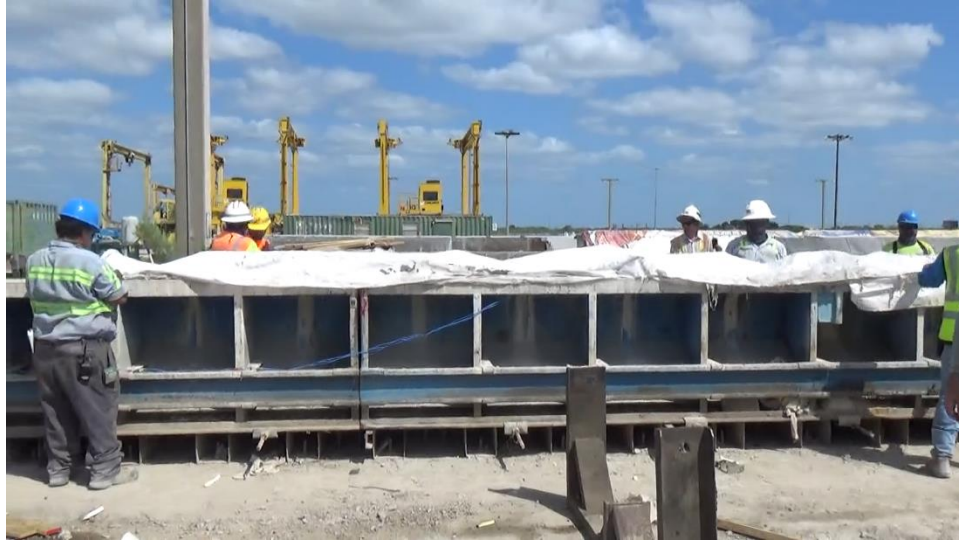
Figure 6.8. UHPC Covered between Placements.
