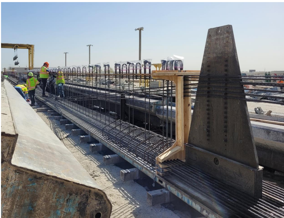
Figure 6.19. Tx54 Prestressing and Reinforcement on the Casting Bed.
