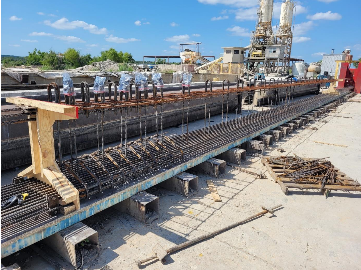
Figure 6.2. Tx34-1 Prestressing and Reinforcement on the Casting Bed.
