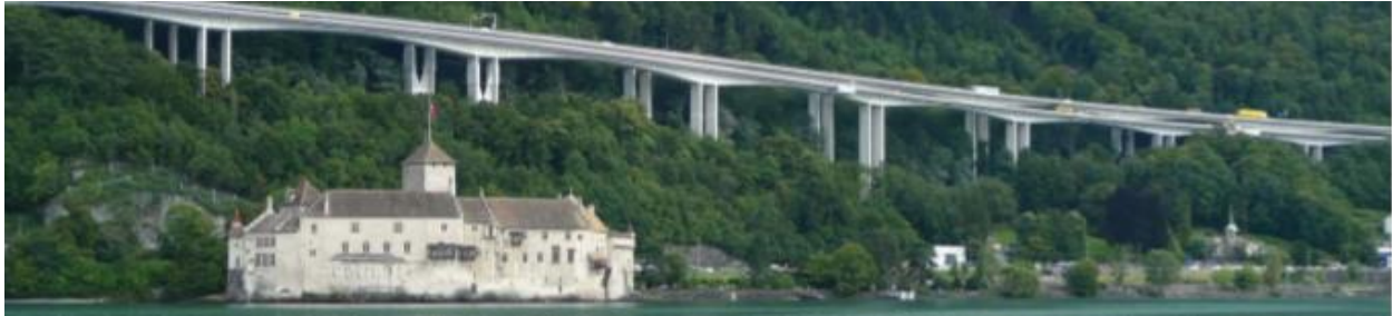
Figure 2.26. Chillon Viaduct, Switzerland (Brühwiler et al. 2015).
