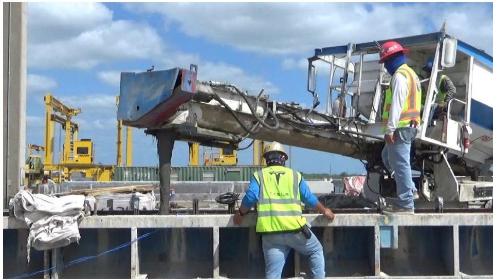
Figure 6.7. Placement of Fresh UHPC Using a Tuckerbuilt.
