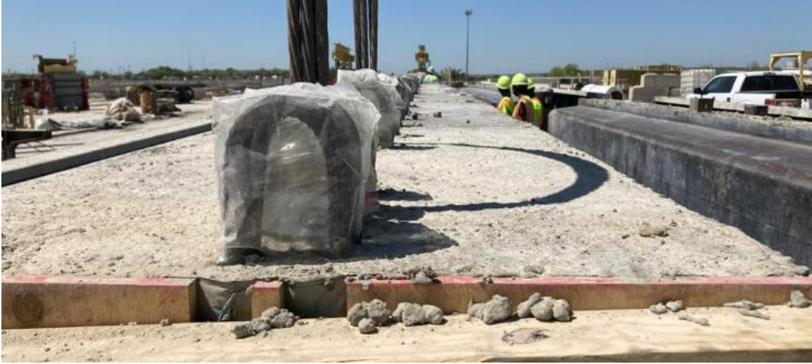
(a) SCC Topping at Top Flange at End without Stirrups
