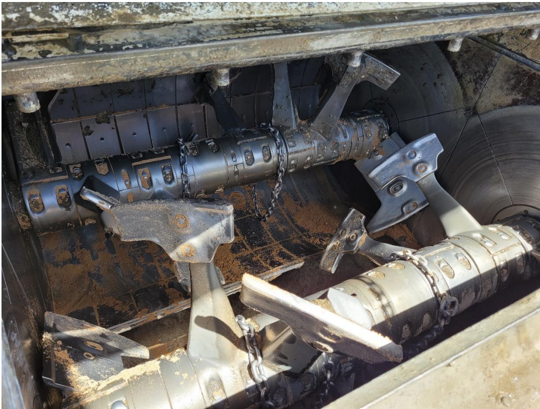
Figure 6.20. Removal of Residual Water Using Dry Sand inside the Mixing Drum.
