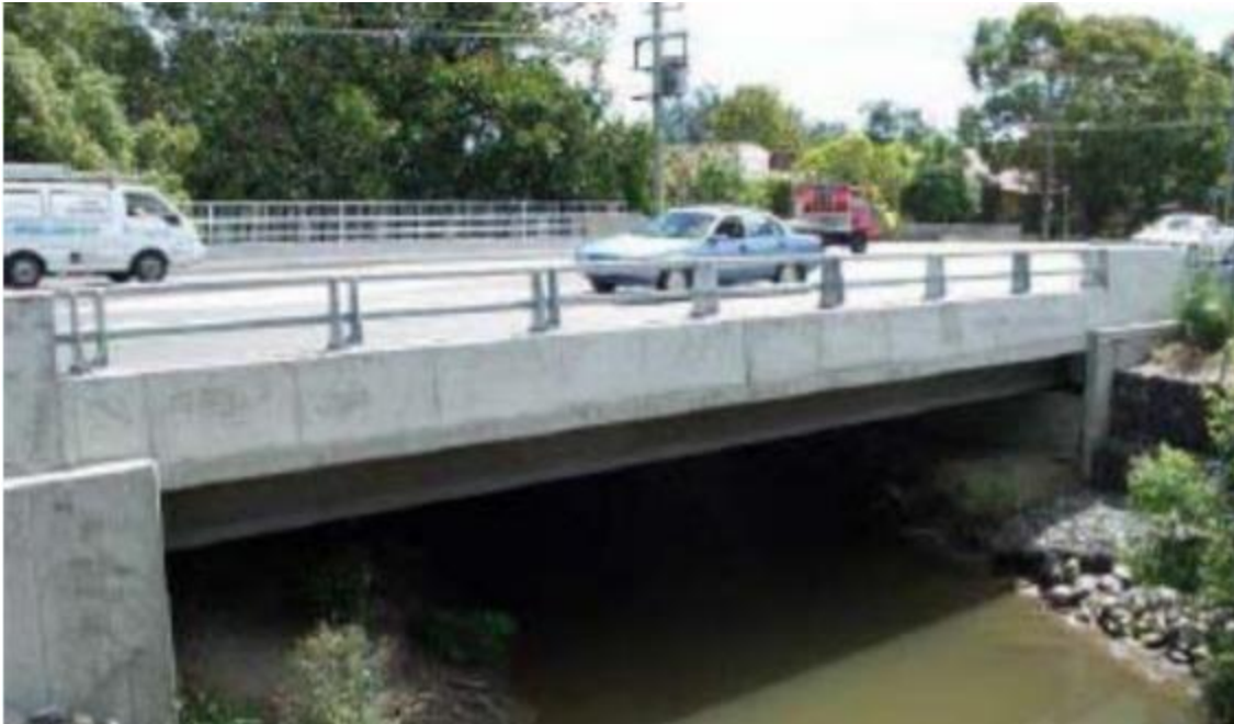
Figure 2.20. Shepherds Creek Road Bridge, Australia (Rebentrost et al. 2008).
