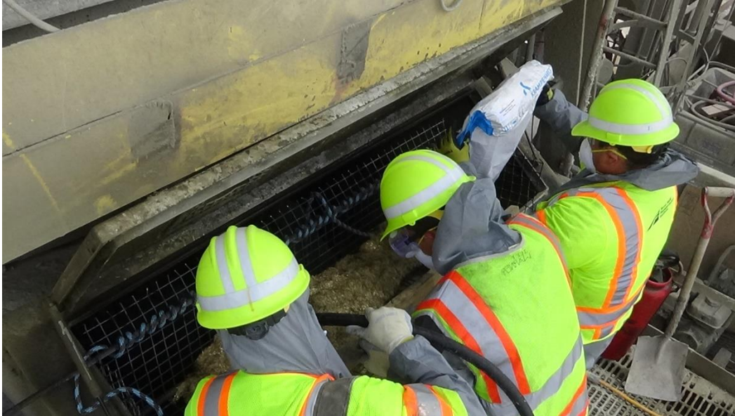
Figure 6.14. Manual Addition of Steel Fibers Using Screen and Concrete Vibrator.
