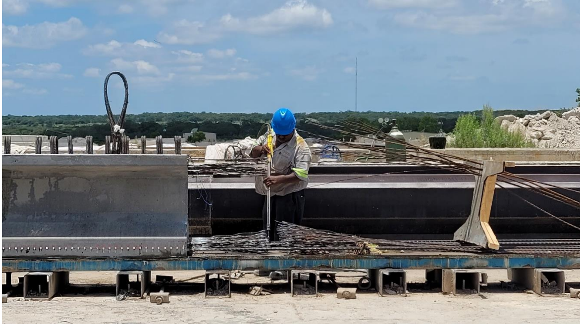
Figure 6.9. Prestress Releasing (Flame Cutting Strands).
