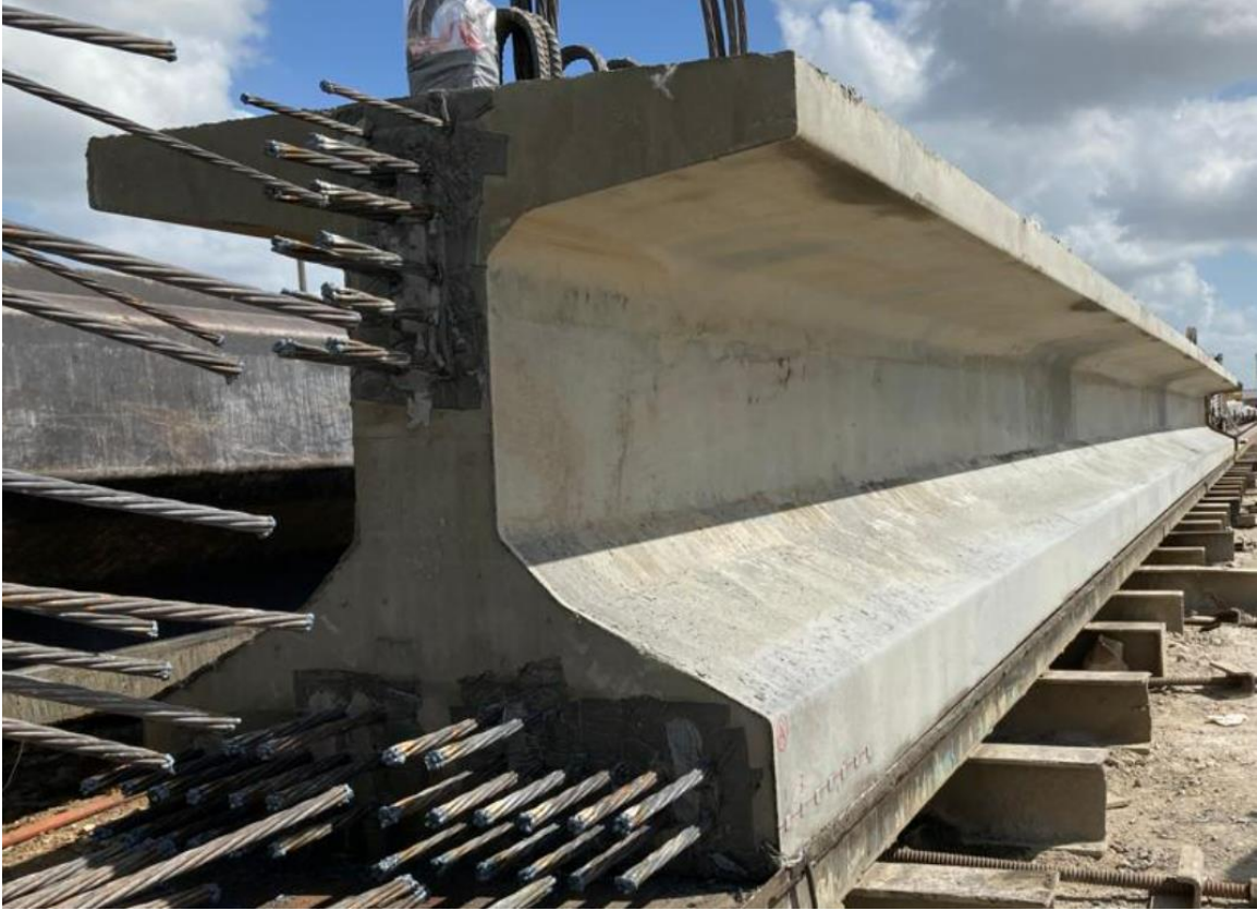
(a) Transition Lines between Batches
