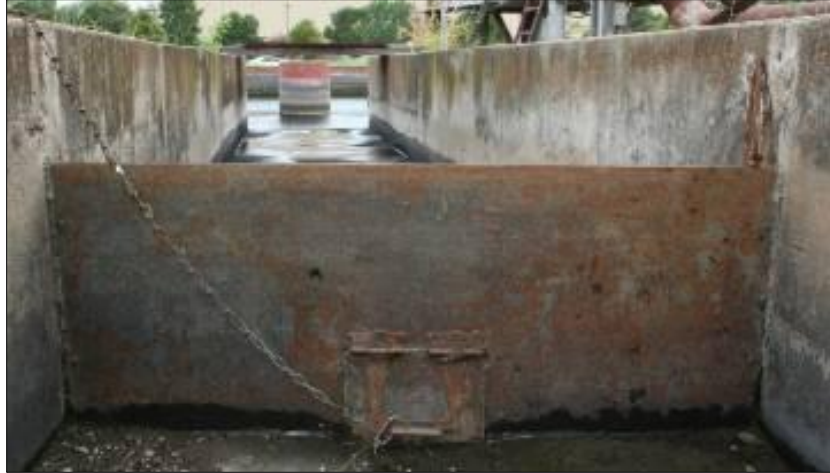
Figure 5.14. Discharge Weir and Gate.
