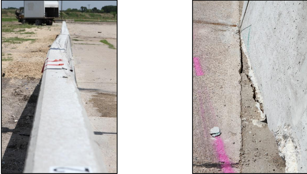
Figure 11.4. Movement of Barrier after Test No. 469760-06-3.
