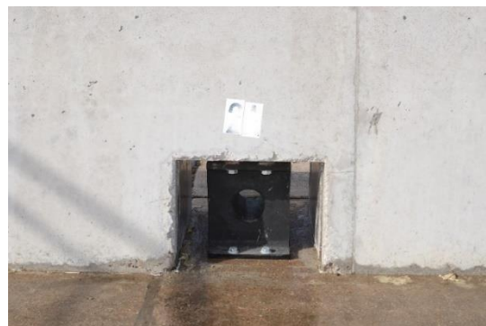
Figure 2.16. Opening in Concrete Barrier to Allow for Rubber Block Installation.
