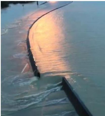
(b) Barrier pushed away from the roadway and finally split apart on Texas USHwy 59 (5).
