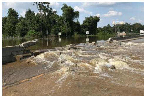
(a) In Beaumont, Texas, several sections of median barrier were exploded to help mitigate the increased flooding being caused by the solid concrete barrier (2).
