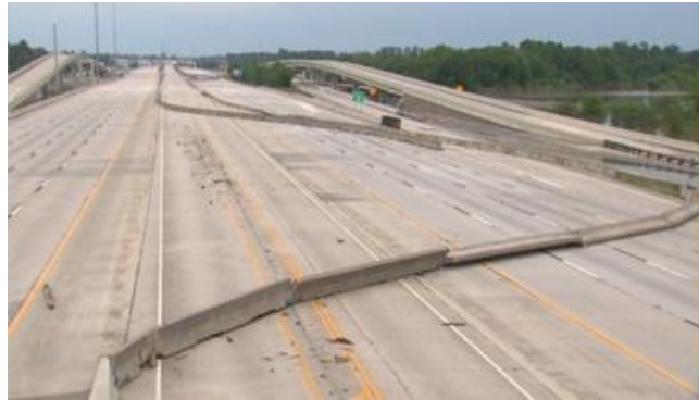
(a) Portable concrete median barrier on the Eastex Freeway was broken and thrust aside after Hurricane Harvey in Humble, Texas (left and above) (4).
