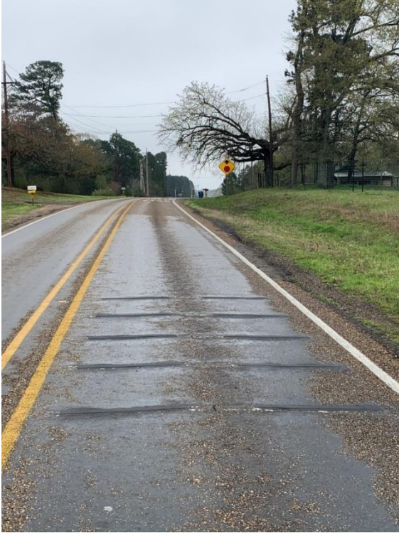
a. Transverse Rumble Strips and Stop Ahead Sign.
