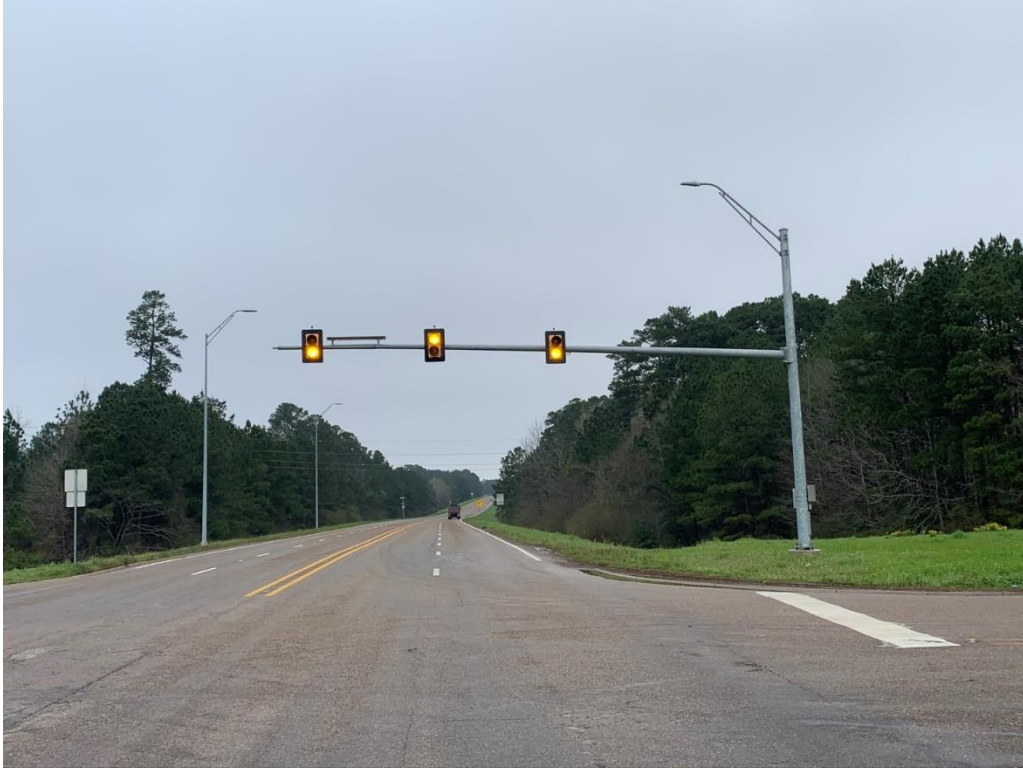
Figure 30. Intersection Improvements on SL 390.
