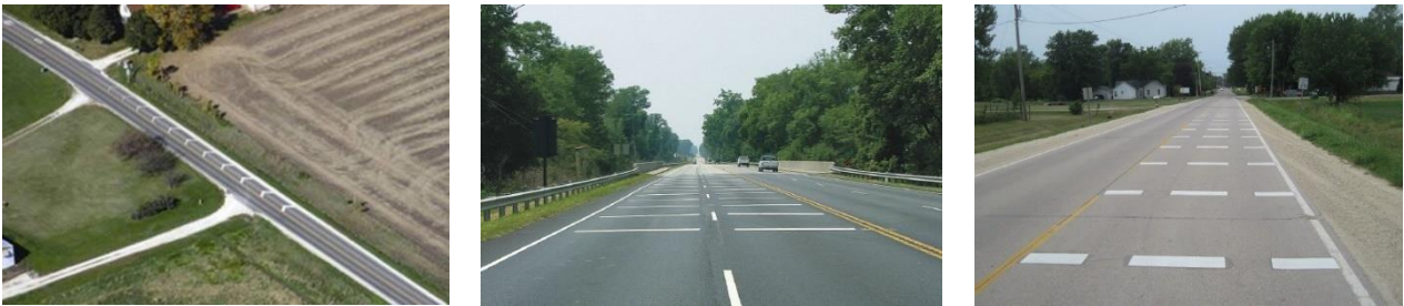
Figure 18. Other Types of Optical Speed Bars (22).
