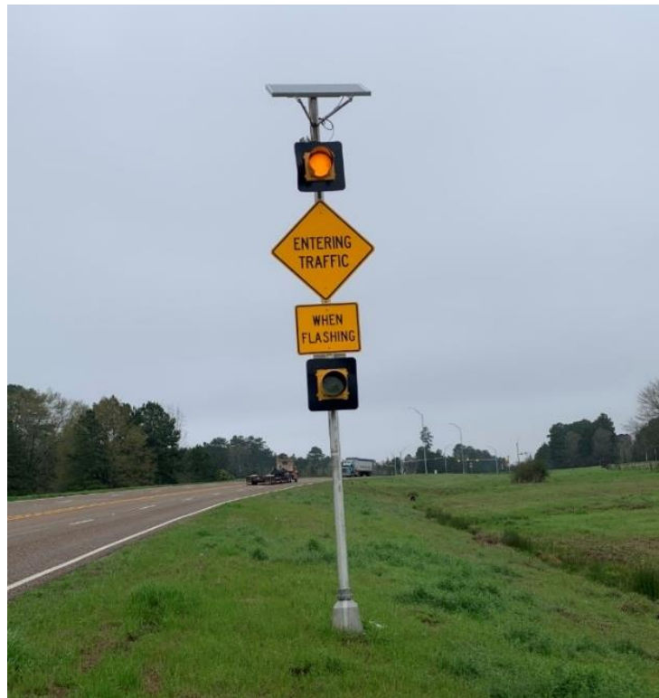
Figure 32. Example of a Solar-Powered RFBA on the Major Street.
