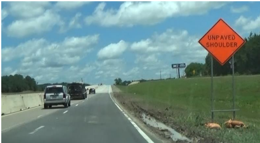
Figure 50. Unpaved Shoulder Warning Sign at Site 3.
