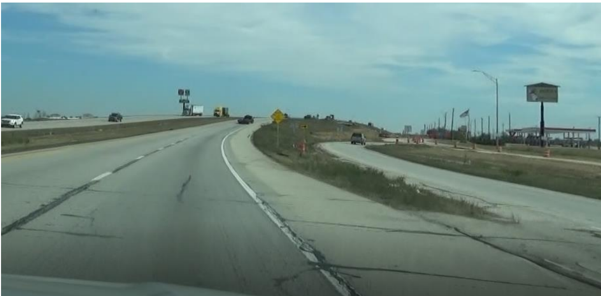
Figure 56. Exit Gore Sign Missing at Site 4.
