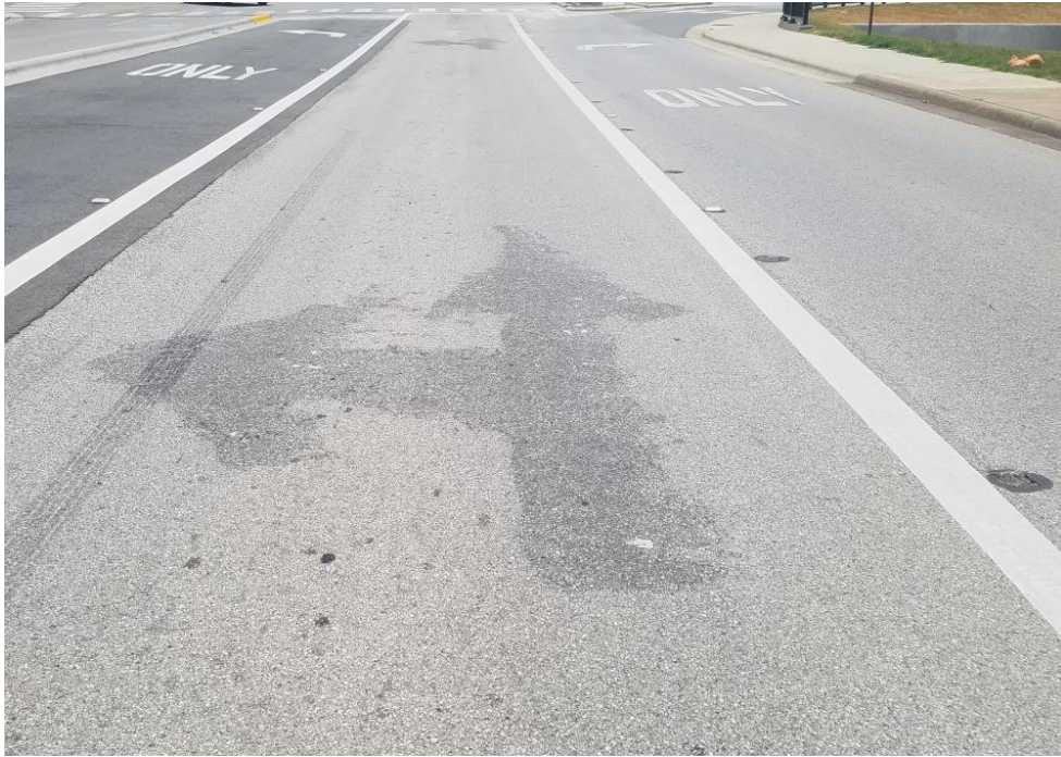
Figure 39. Hand-Operated Flailing Removal on Asphalt.
