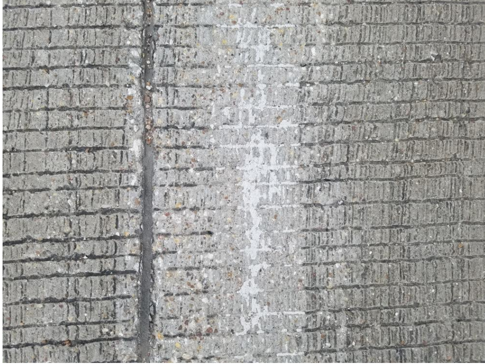
Figure 37. Flailing Removal on Grooved Concrete—Marking Remnants in Grooves.
