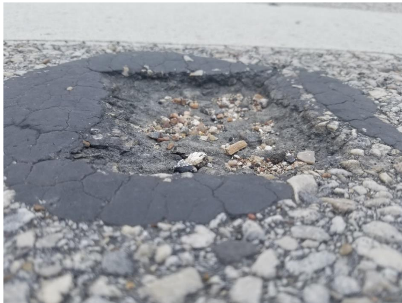
Figure 40. Marker Removal on Asphalt.
