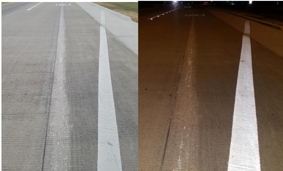
Figure 36. Flailing Removal of Edge Line on Grooved Concrete (Day and Night).
