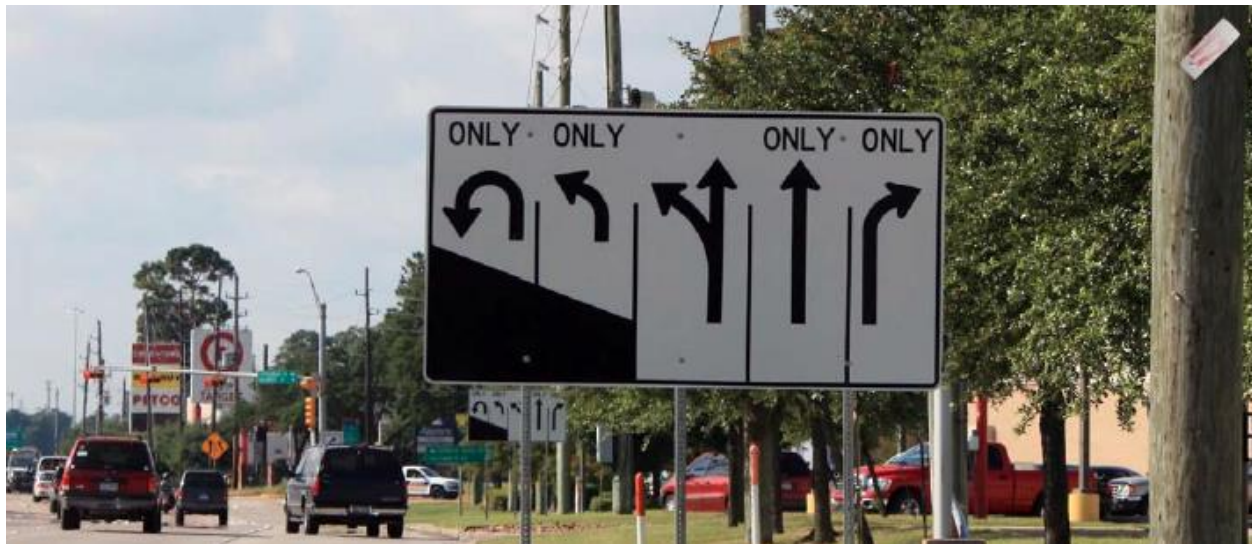
Figure 12. Close-Up of Alternative Advance Intersection Lane Control Sign (12).
