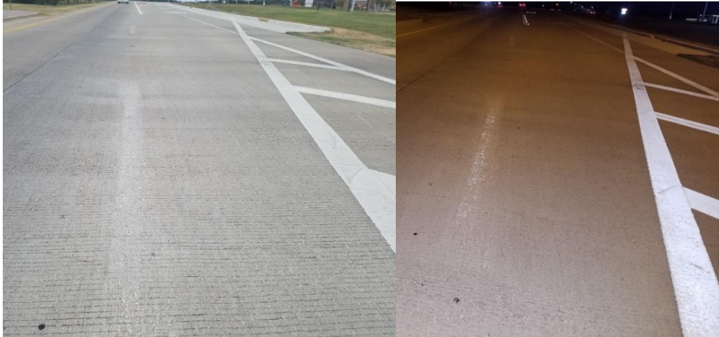
Figure 35. Flailing Removal of Lane Line on Grooved Concrete (Day and Night).
