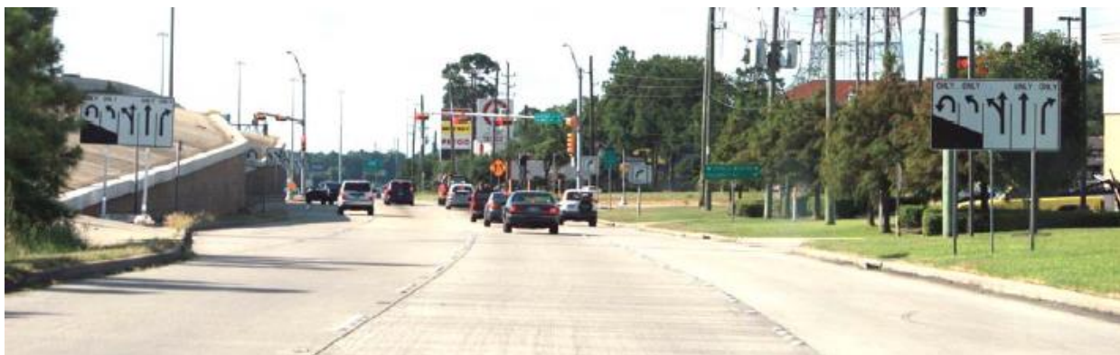
Figure 13. Set of Alternative Advanced Intersection Lane Control Signs at IH-45 Southbound at Cypresswood Drive in Houston (12).
