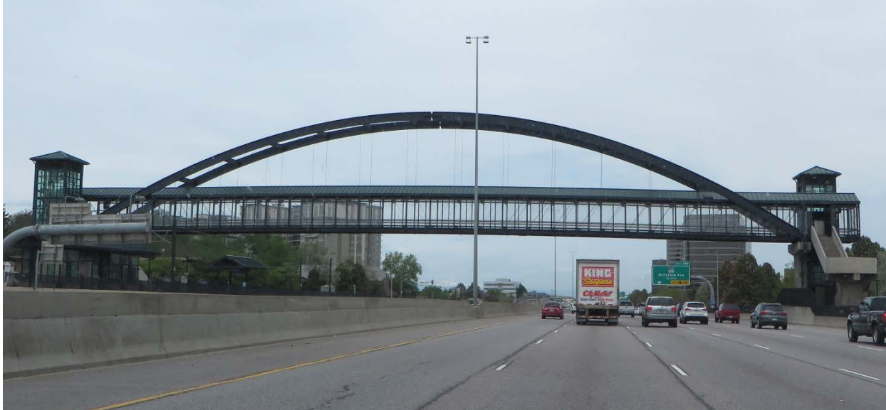
Figure 13. Pedestrian Overpass on I-25 in Denver, CO.
