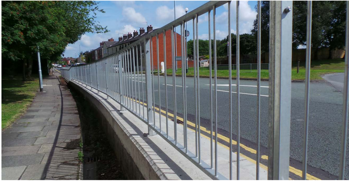
Figure 14. Example of Pedestrian Barrier Fence along Edge of Right of Way (Source: http://www.triadfabs.com/product/pedestrian-guard-rails ).
