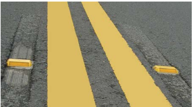
(c) Groove-Recessed RRPMs.
