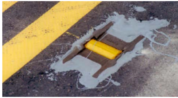
(b) Snowplowable RRPMs with Cast Metal Housing.
