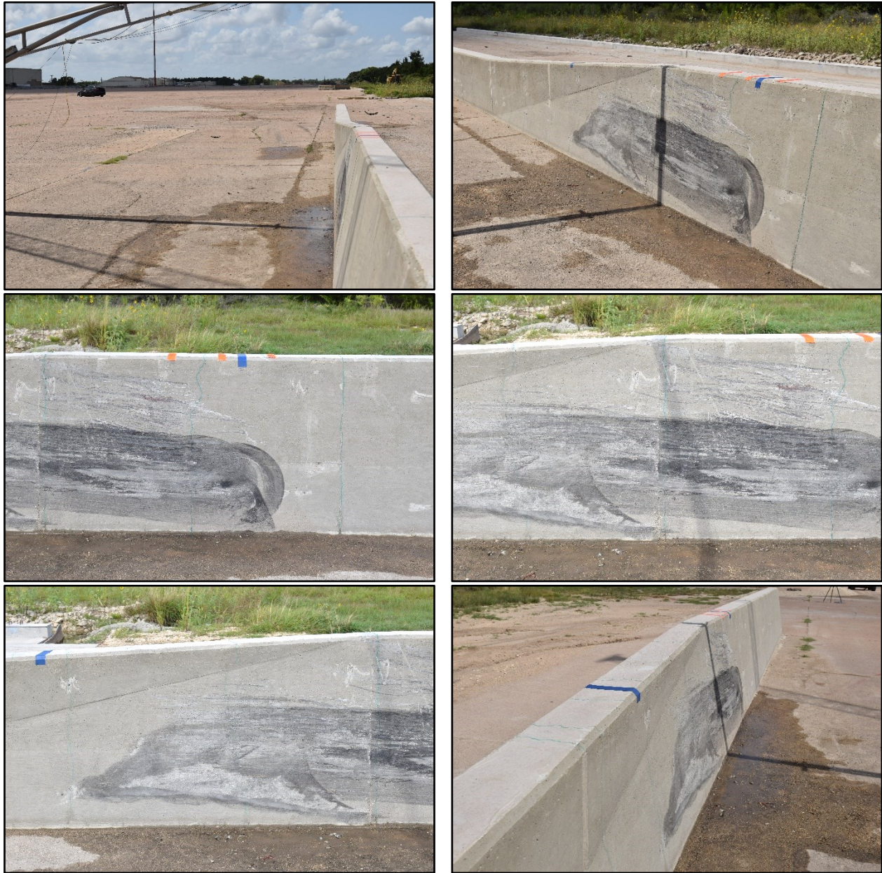
Figure 6.3. T221 vertical wall to SSCB transition after Test No. 469689-2-1.
