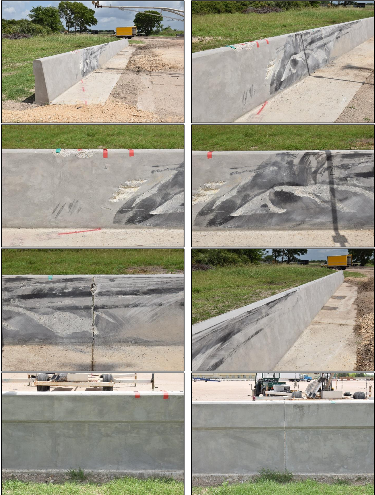
Figure 6.3. Barrier after Test No. 469689-3-3.
