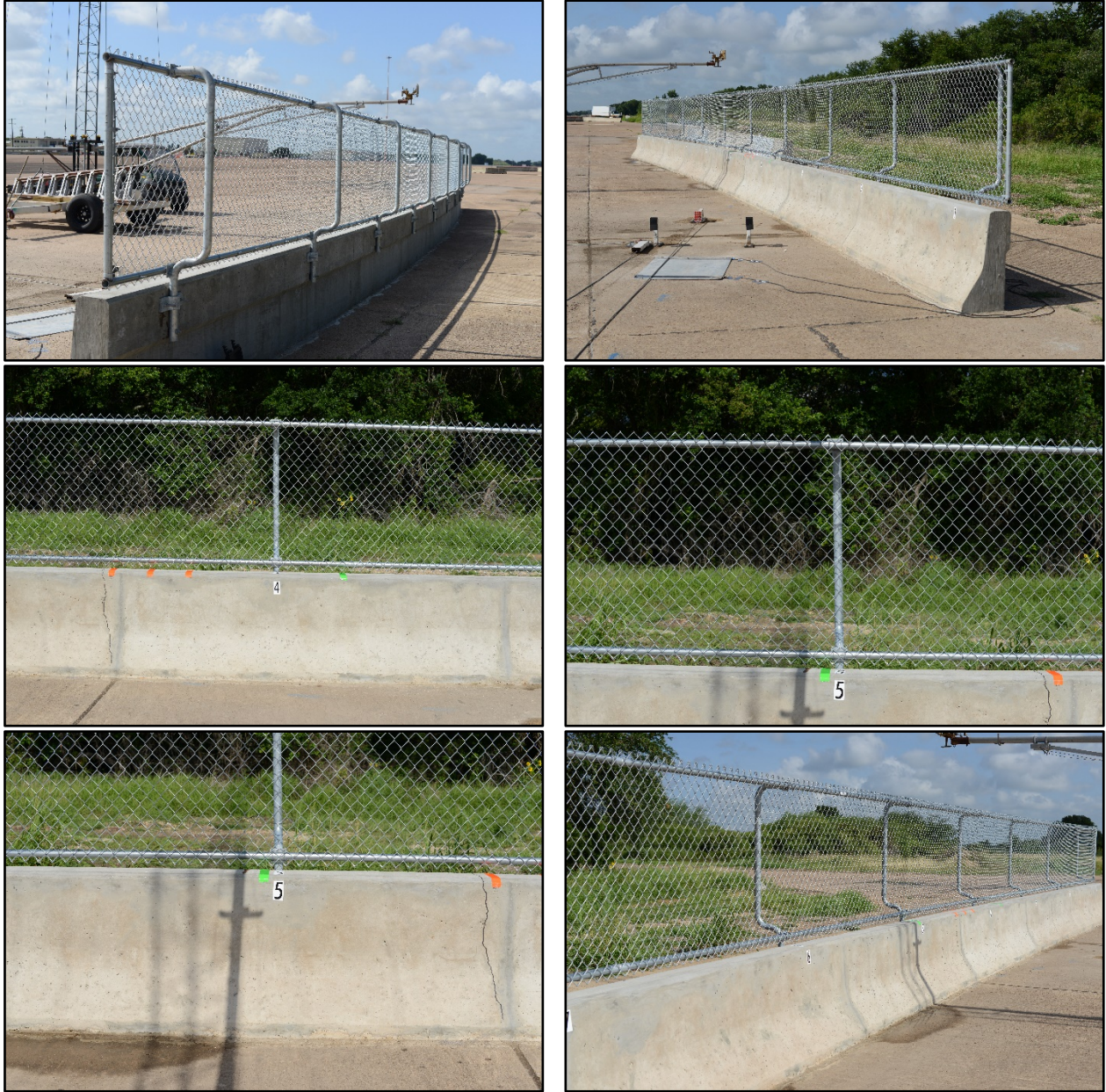
Figure 6.2. TxDOT Fence Barrier for Motorcycles prior to Testing.
