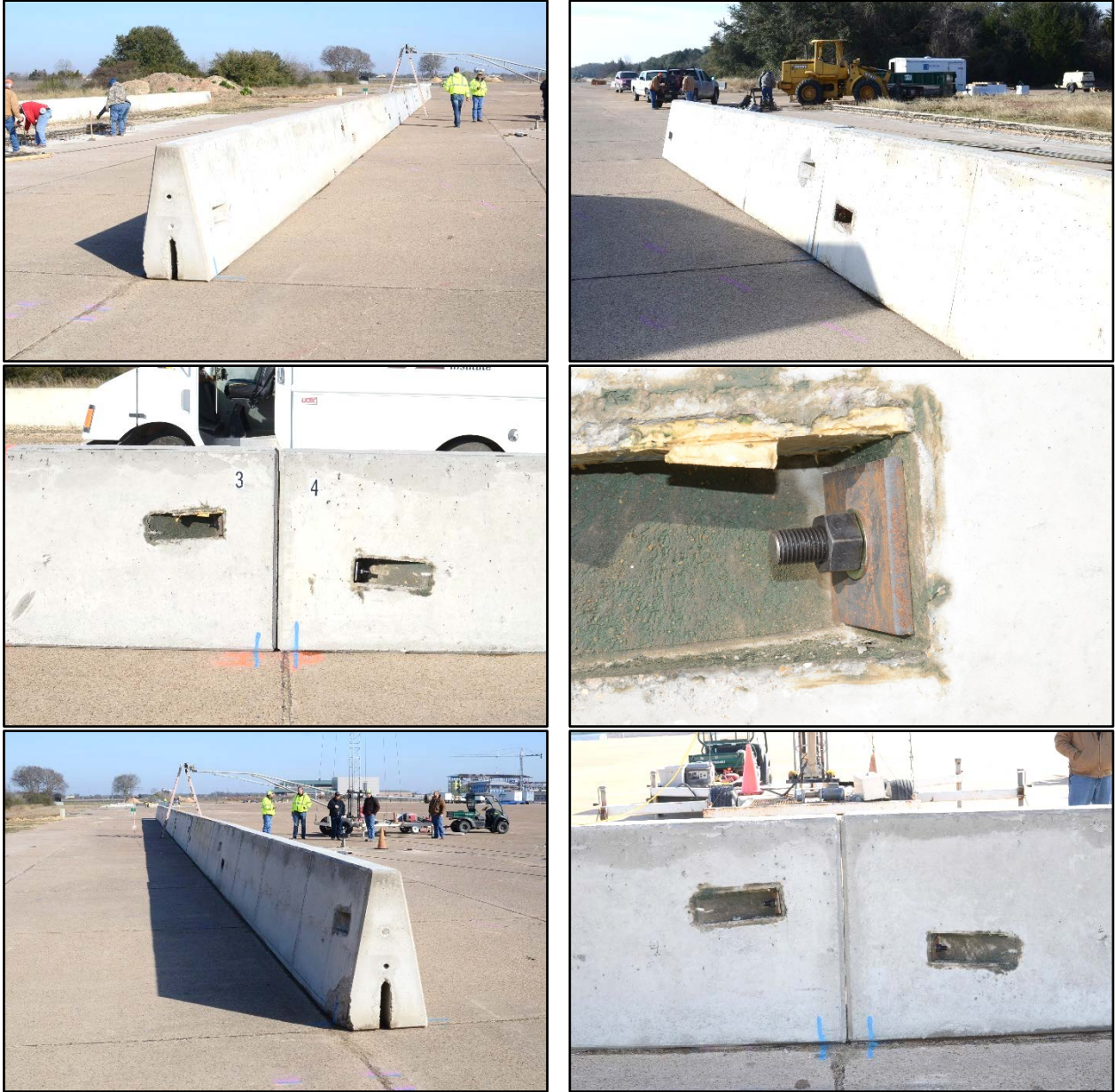
Figure 2.2. Free-Standing SSCB with Cross-Bolt Connection prior to Testing.
