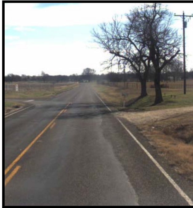
Figure 46. FM 339 Example of Flushed Left Wheel Path, Partially Flushed between Wheel Paths, and Better Right Wheel Path.
