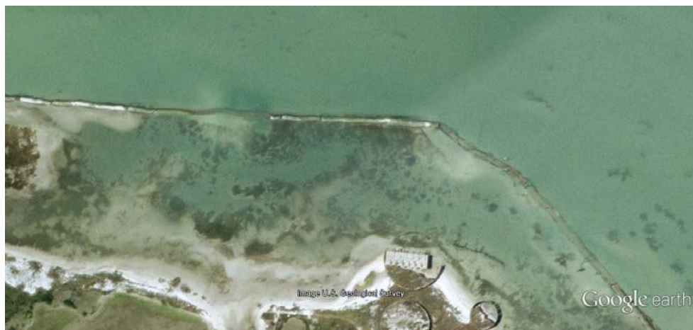
Figure 9. Close-Up of Geotextile Tubes in 2004 Failing.
