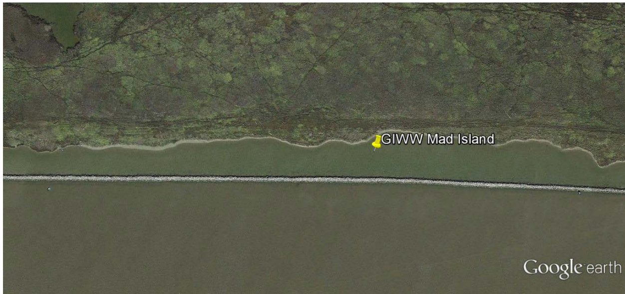
Figure 25. Shorelines of GIWW (Stations 826+000 to 828+000) at Mad Island after Installation of Rock Breakwater, January 2014.
