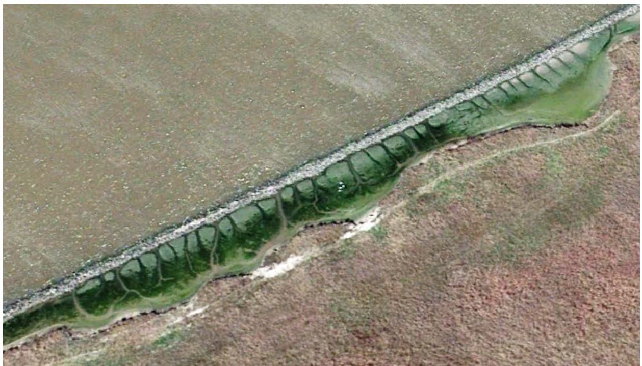
Figure 41. Sediment Distribution Pattern between Rock Breakwater and Shoreline at GIWW McFaddin Refuge Shoreline Protection Project Site in 2010.
