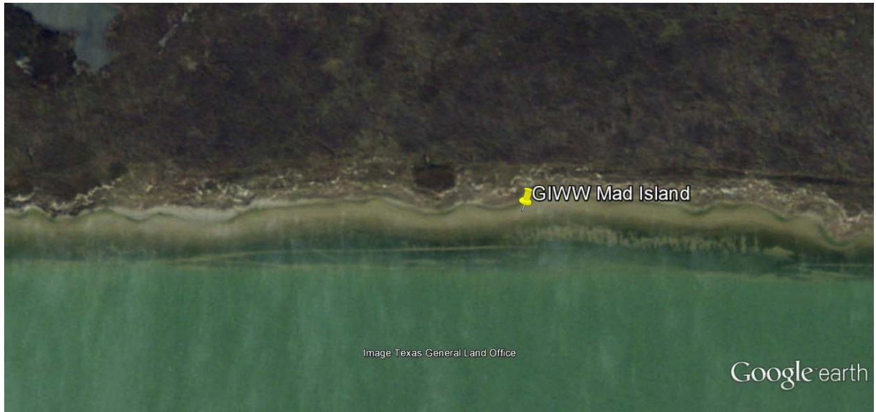
Figure 24. Retreating Shorelines and Eroding Marshes along GIWW (Stations 826+000 to 828+000) at Mad Island, January 2009.
