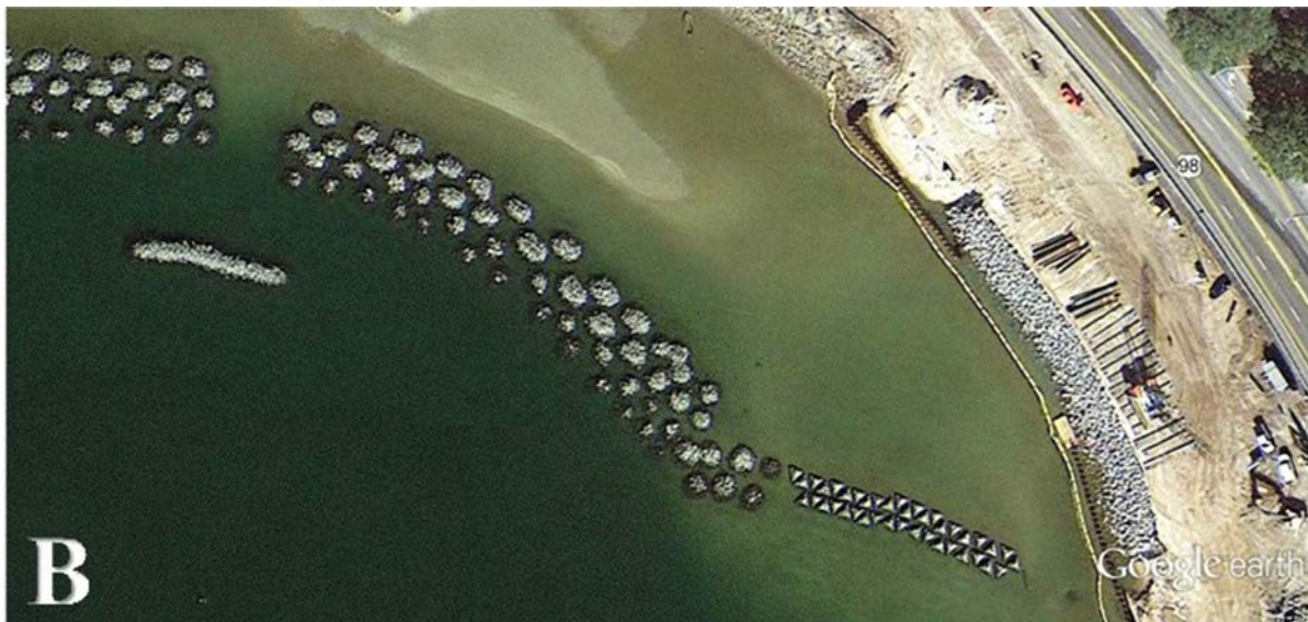
Figure 43. Segmented Breakwater Systems in Pensacola Bay, Florida. Source Google Earth
