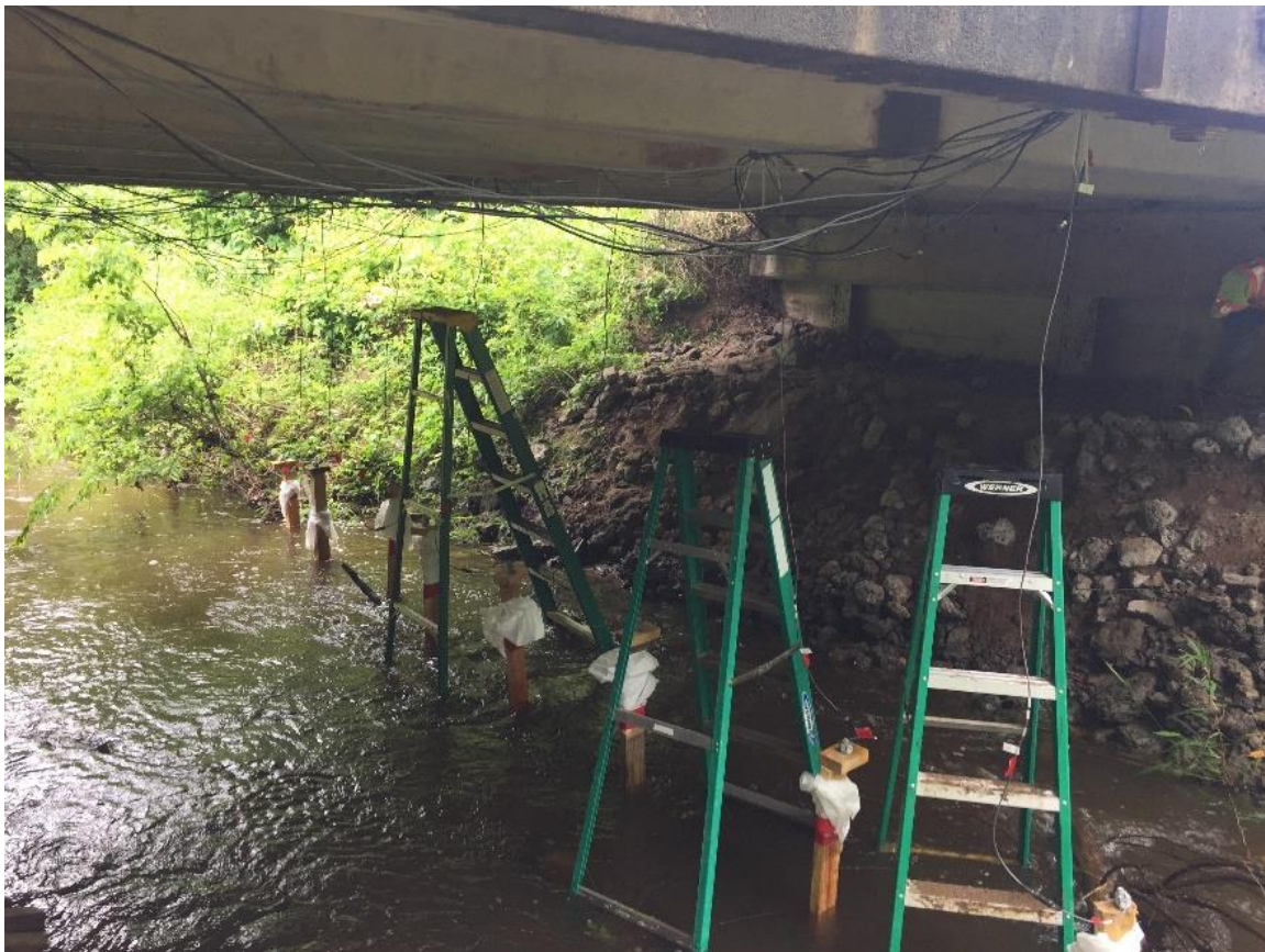
(c) Installed String Potentiometers
