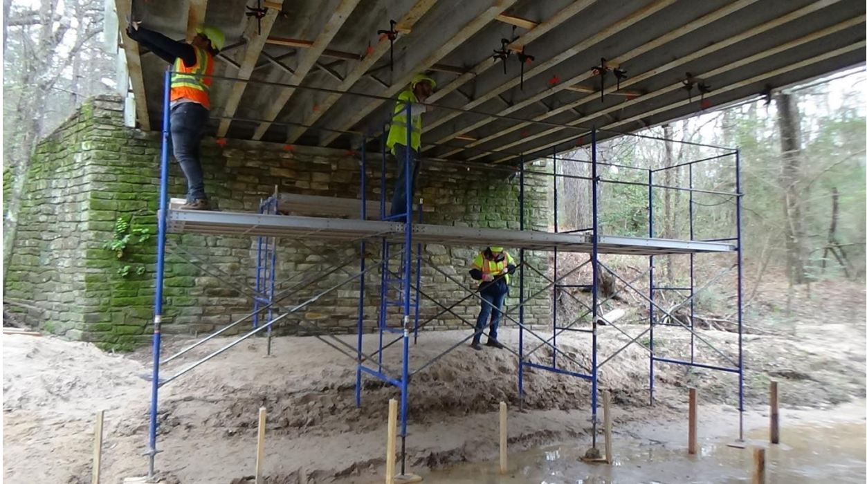
(a) Instrumentation of Bridge SM-5
