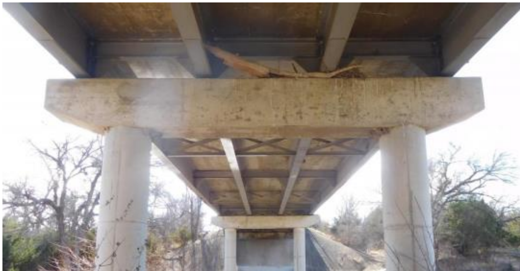
(b) Underside view
