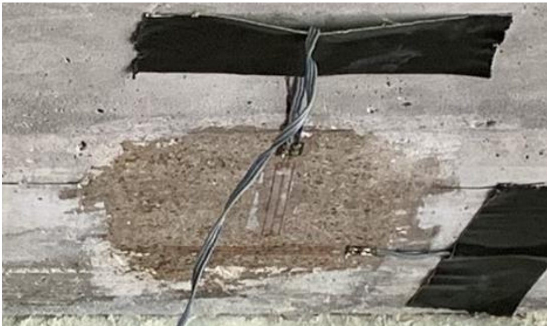
Figure 9.4. Close-Up of Strain Gauge Installation
