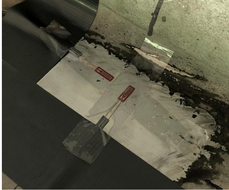
Figure 7.8. Close-Up of Strain Gauge Installation
