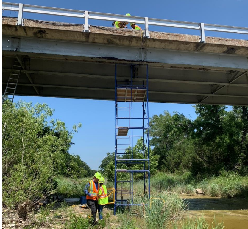
(a) Instrumentation of Bridge SC-12
