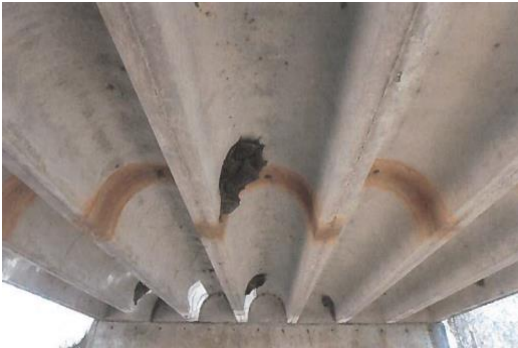
(b) Underside view
