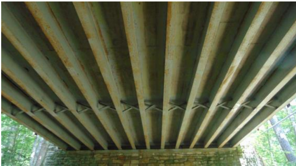
(b) Underside view
