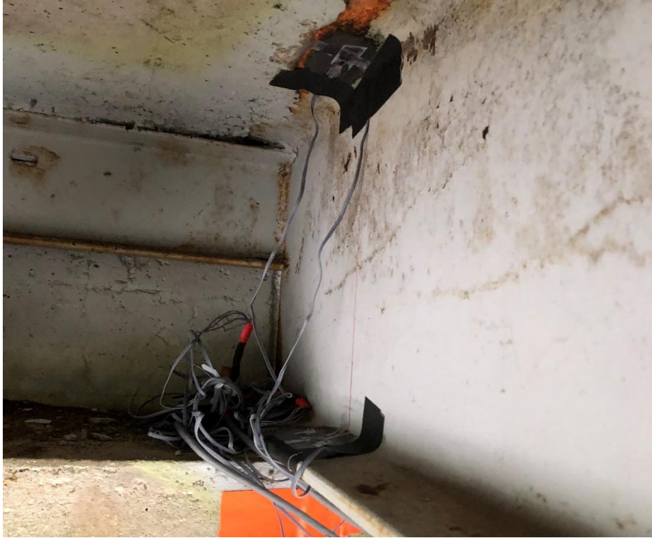
(a) Installed Strain Gauges at an End Location of a Girder
