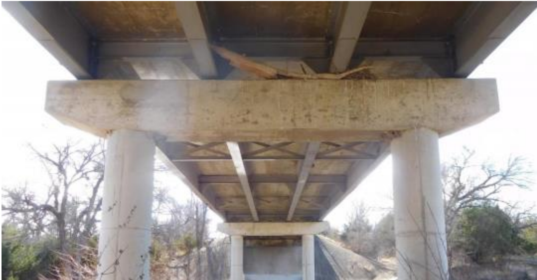
(b) Underside view
