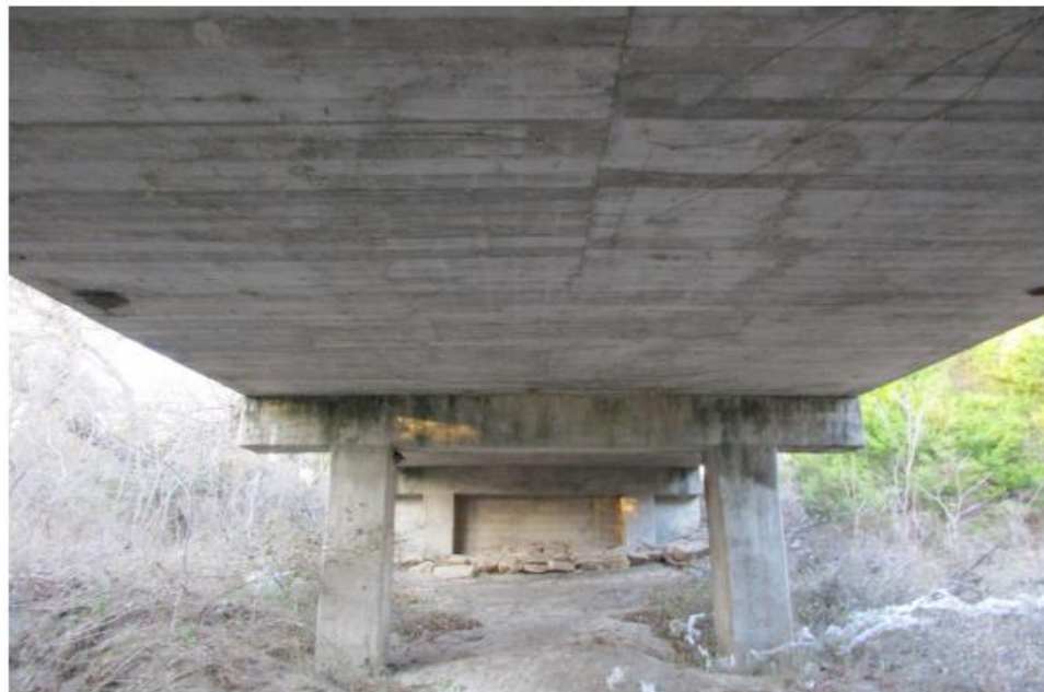
(b) Underside View
