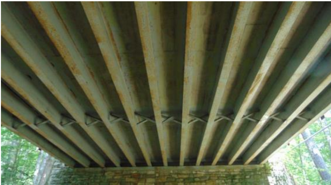
(b) Underside view
