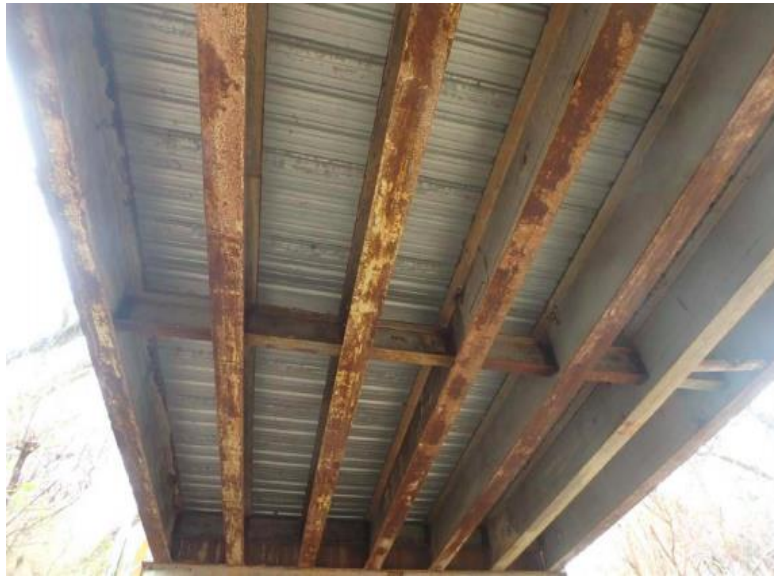
(b) Underside view
