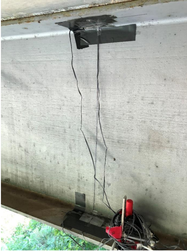
(a) Example of Installed Strain Gauges
