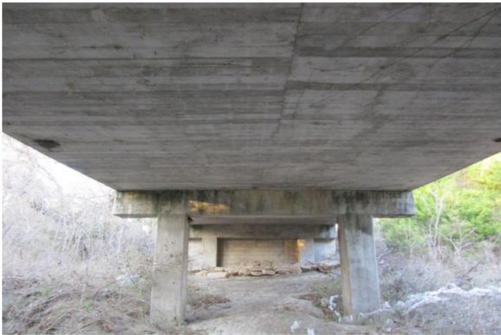
(b) Underside View
