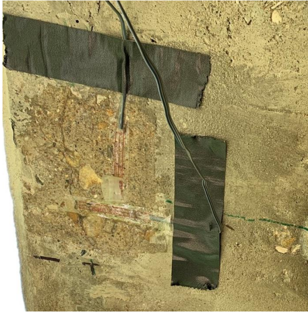
(a) Installed Strain Gauges
