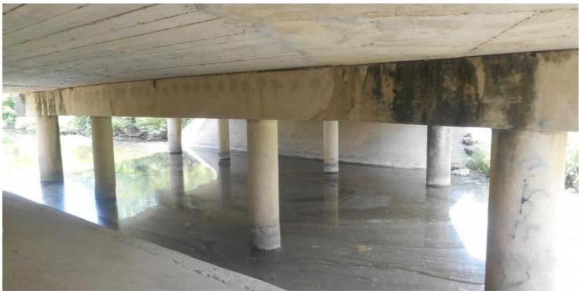
(c) Underside Superstructure View
