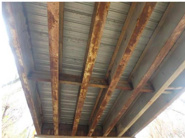
(c) Underside Superstructure View
