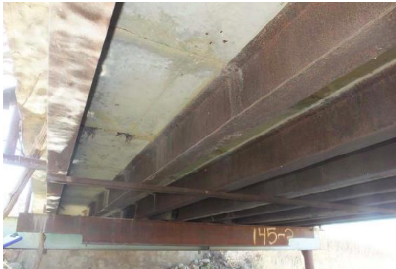
(c) Underside Superstructure View
