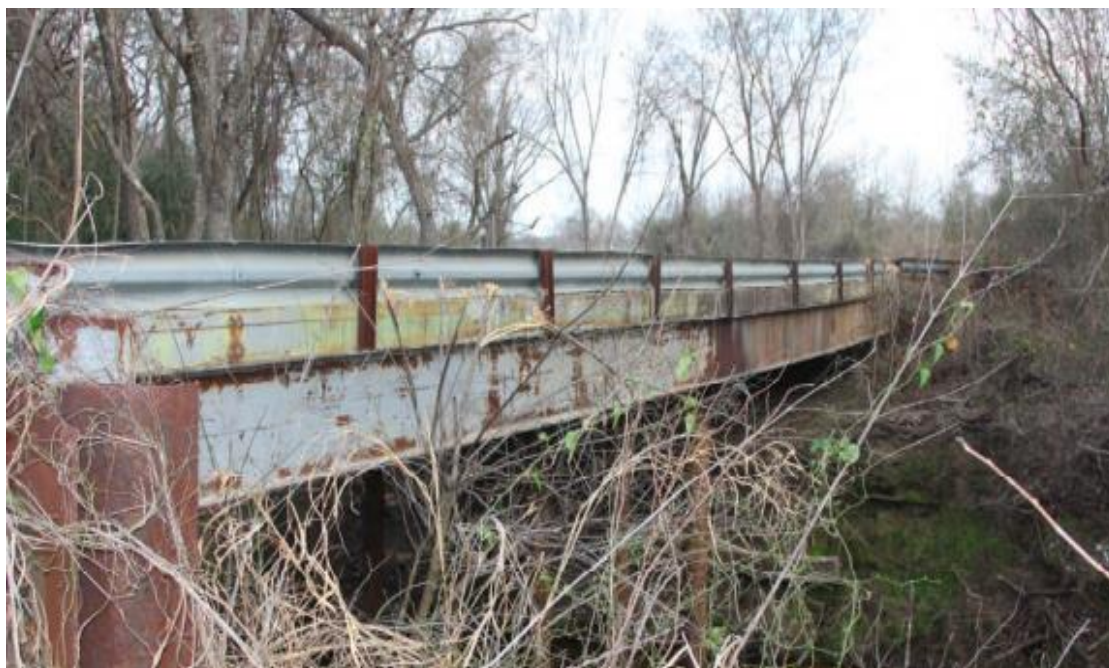
Figure B.81. Bridge SC-16 (TxDOT 2018c)
