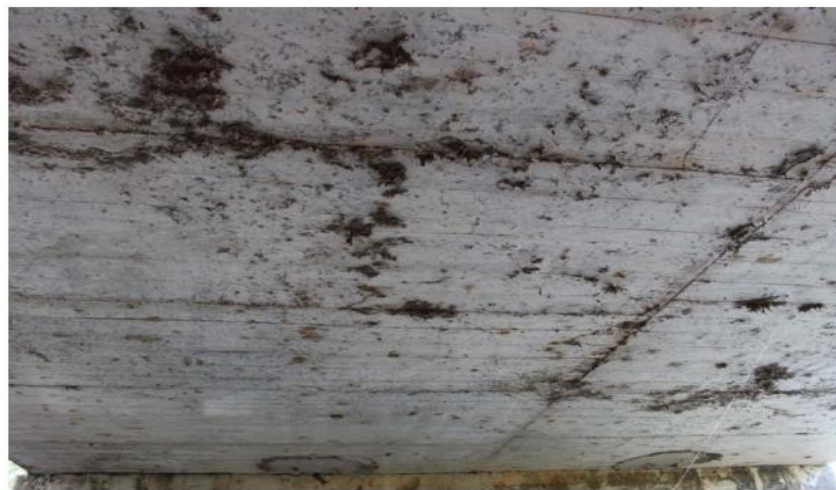
(c) Underside Superstructure View
