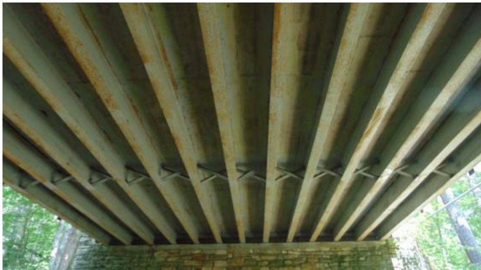
(c) Underside Superstructure View
