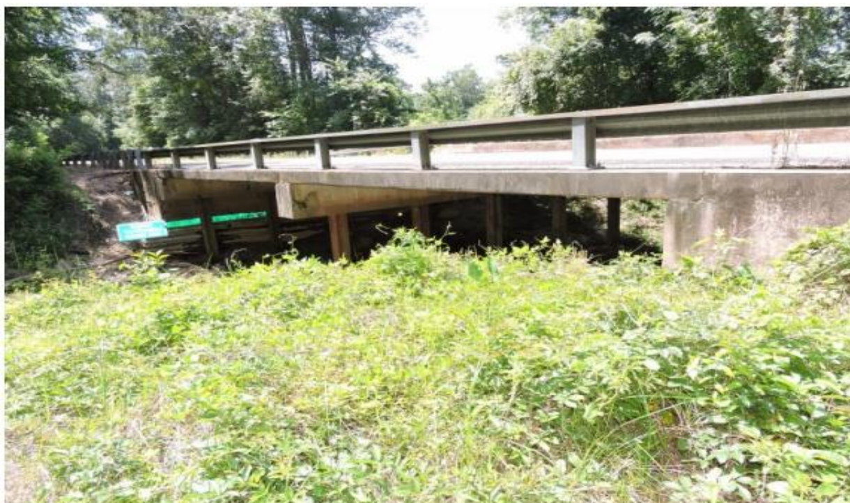
Figure C.37. Bridge CS-19 (TxDOT 2018c)
