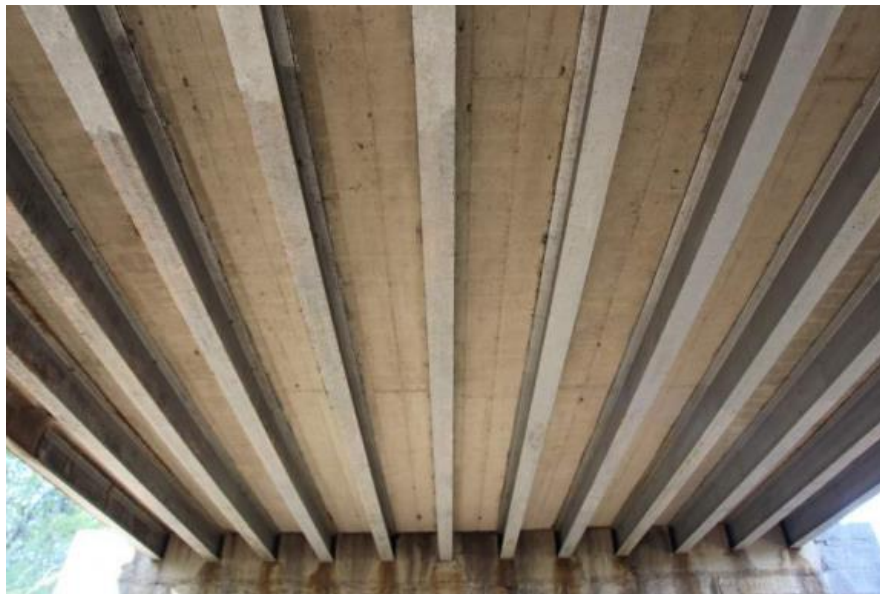
(c) Underside Superstructure View
