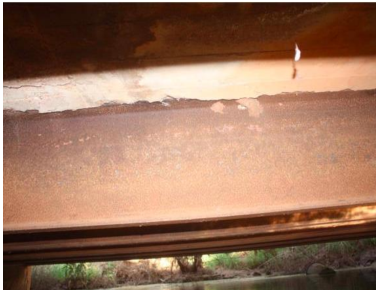
(c) Underside Superstructure View
