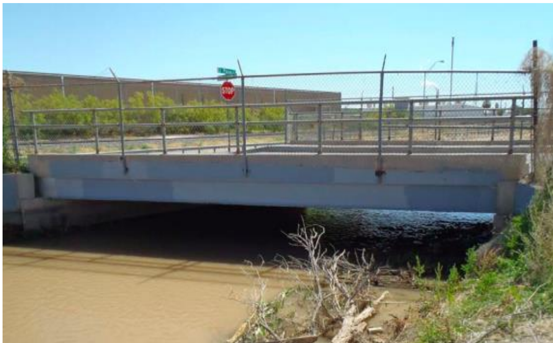
Figure B.31. Bridge SM-16 (TxDOT 2018c)
