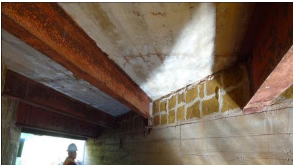
(c) Underside Superstructure View
