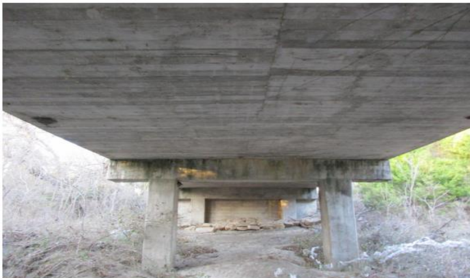
(c) Underside Superstructure View
