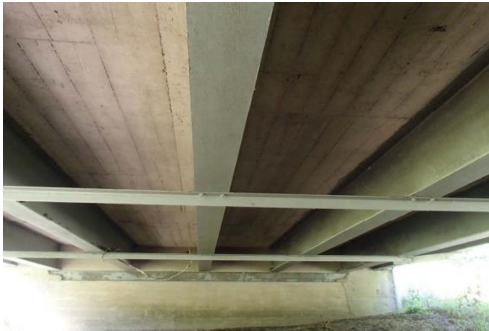
(c) Underside Superstructure View
