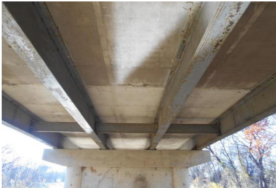
(c) Underside Superstructure View
