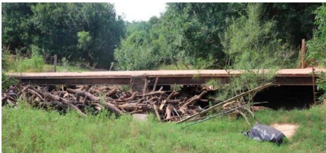
Figure B.53. Bridge SC-2 (TxDOT 2018c)
