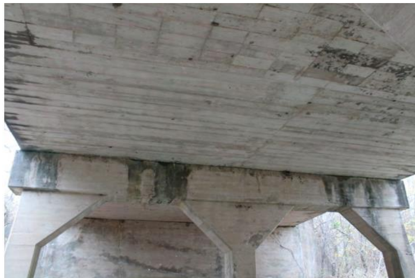
(c) Underside Superstructure View
