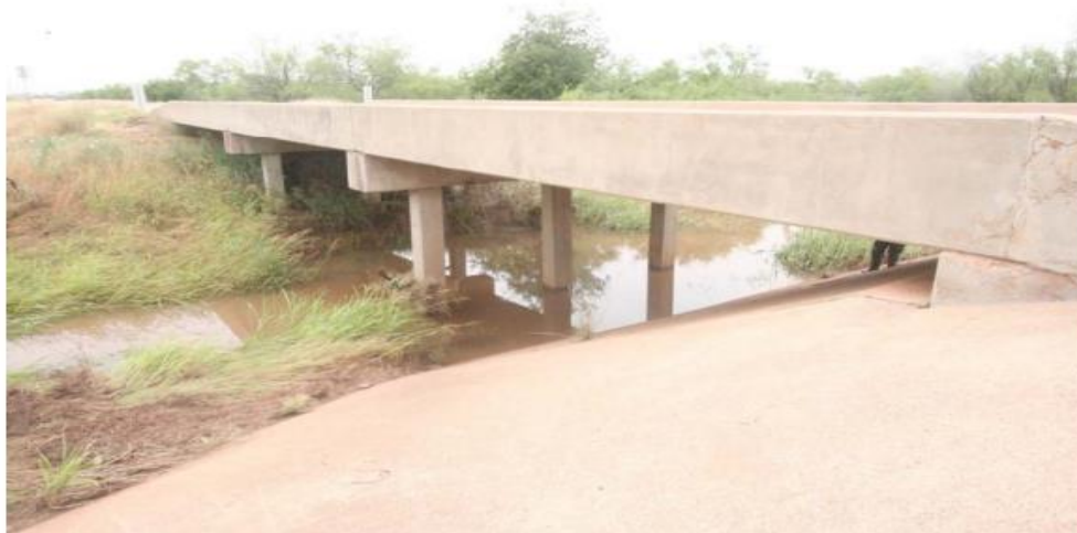
Figure C.33. Bridge CS-17 (TxDOT 2018c)
