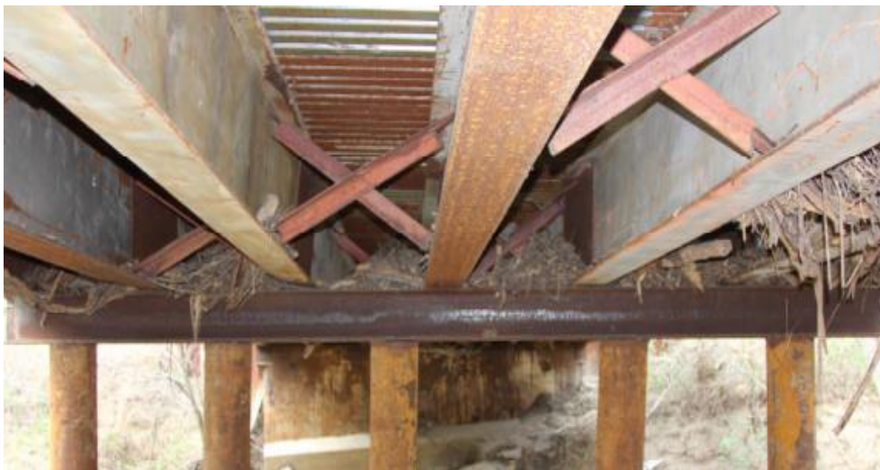
(c) Underside Superstructure View
