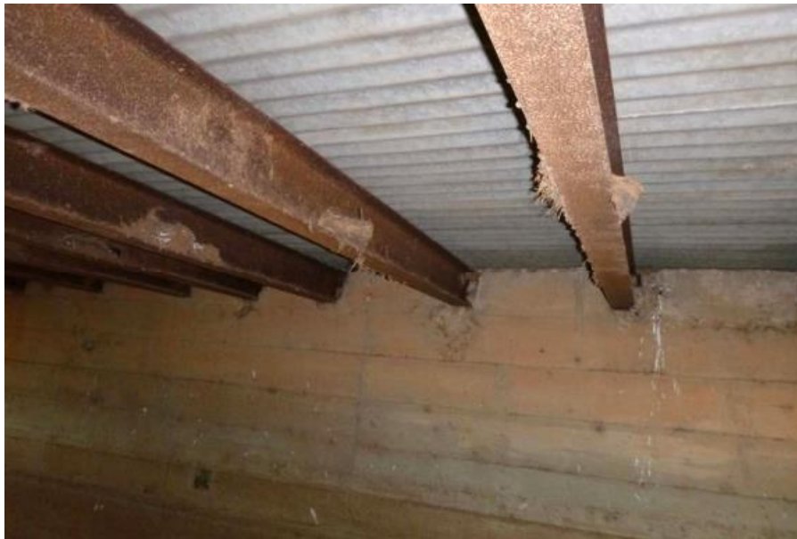
(c) Underside Superstructure View
