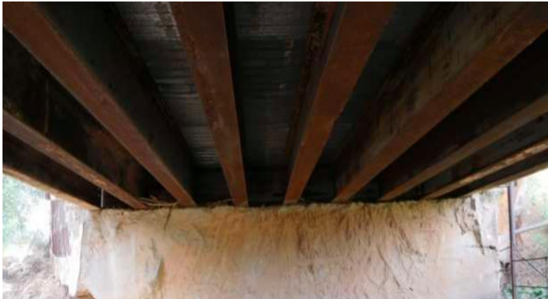
(c) Underside Superstructure View
