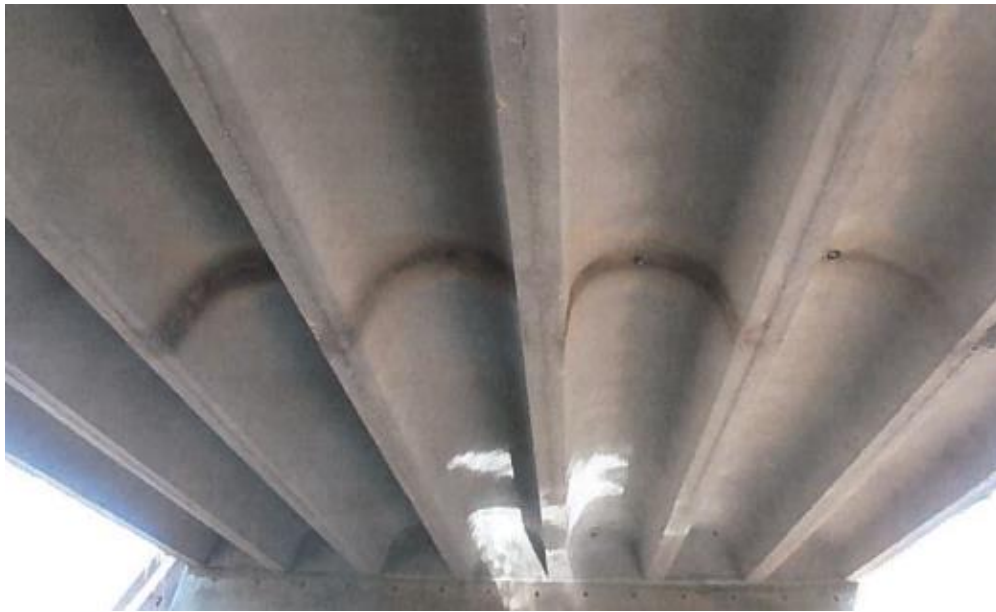
(c) Underside Superstructure View
