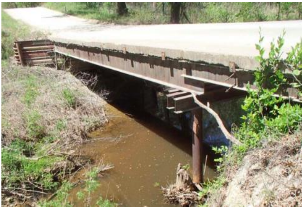
Figure B.77. Bridge SC-14 (TxDOT 2018c)
