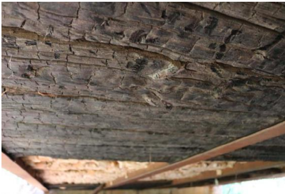
(c) Underside Superstructure View
