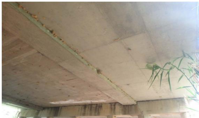
(c) Underside Superstructure View
