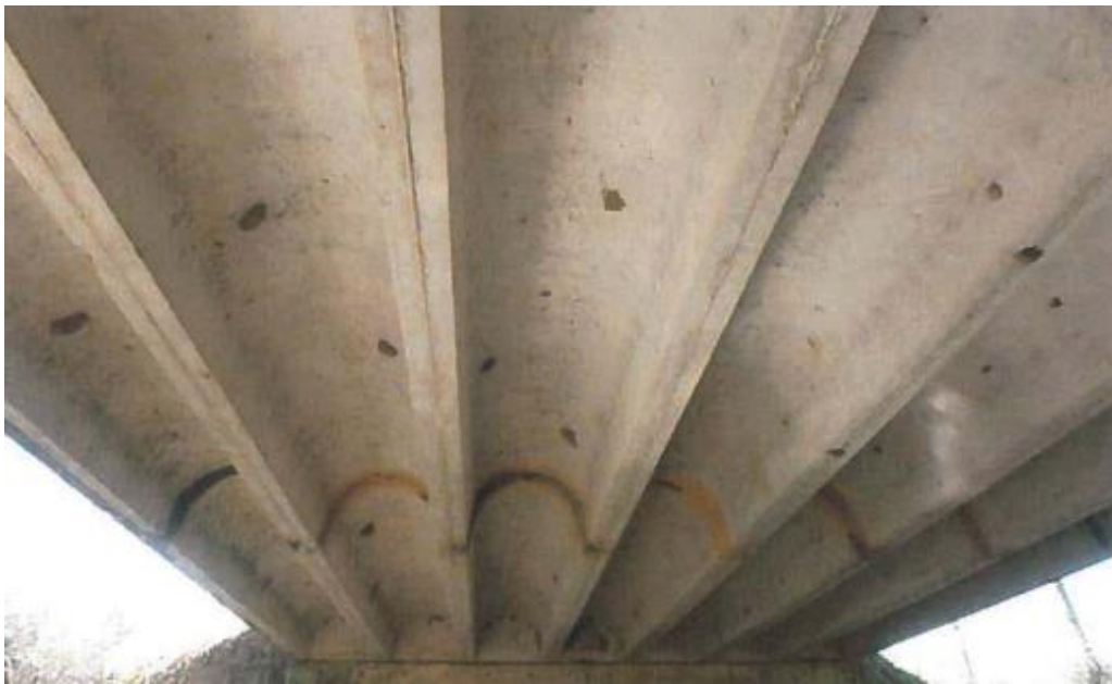
(c) Underside Superstructure View
