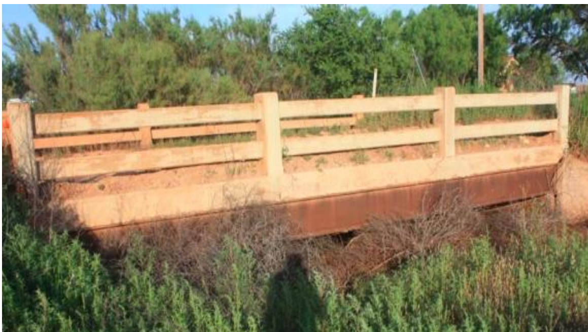
Figure B.19. Bridge SM-10 (TxDOT 2018c)
