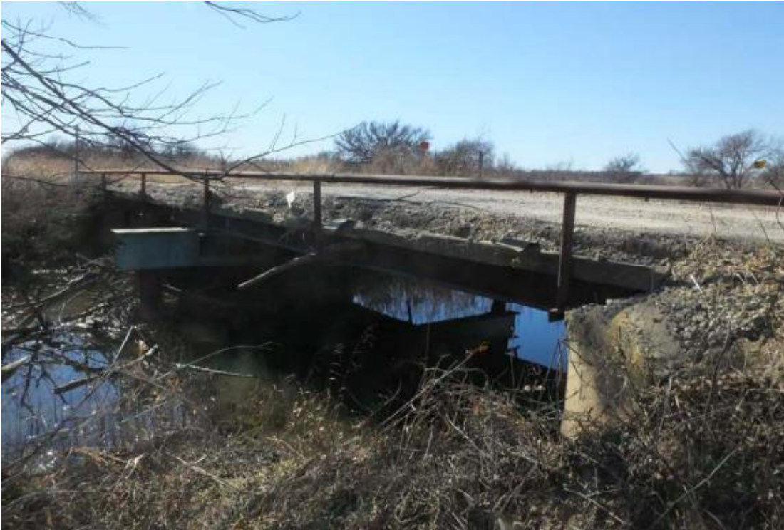
Figure B.57. Bridge SC-4 (TxDOT 2018c)
