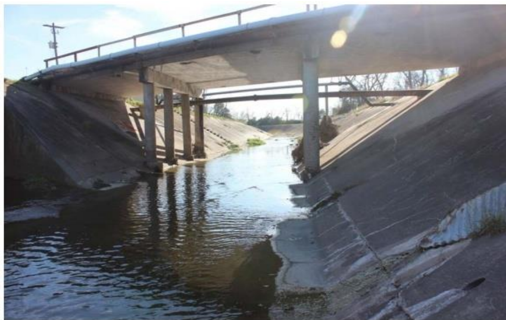
Figure C.45. Bridge CS-23 (TxDOT 2018c)
