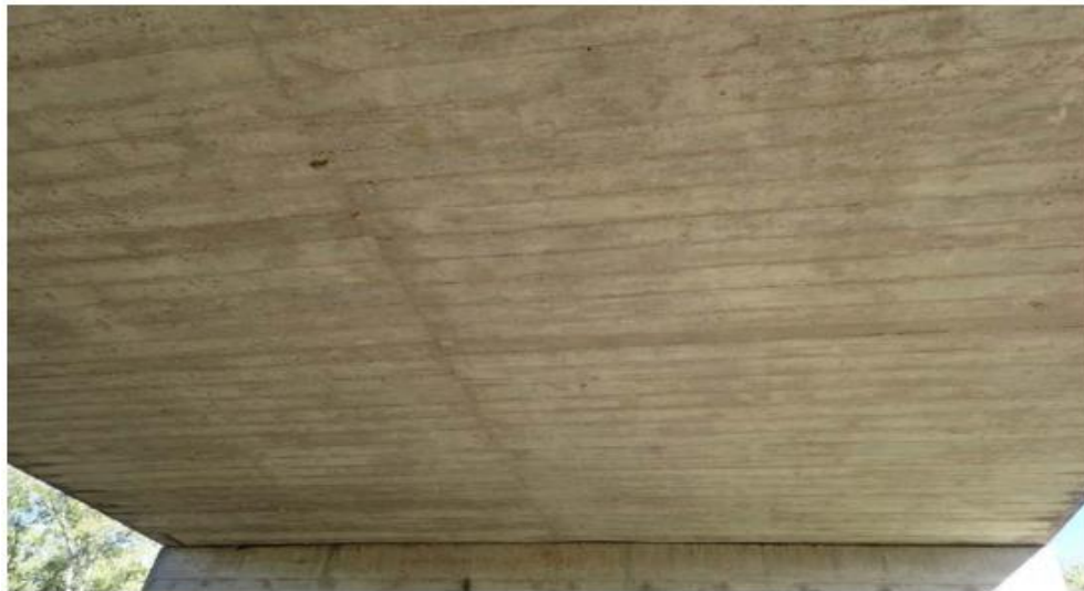
(c) Underside Superstructure View
