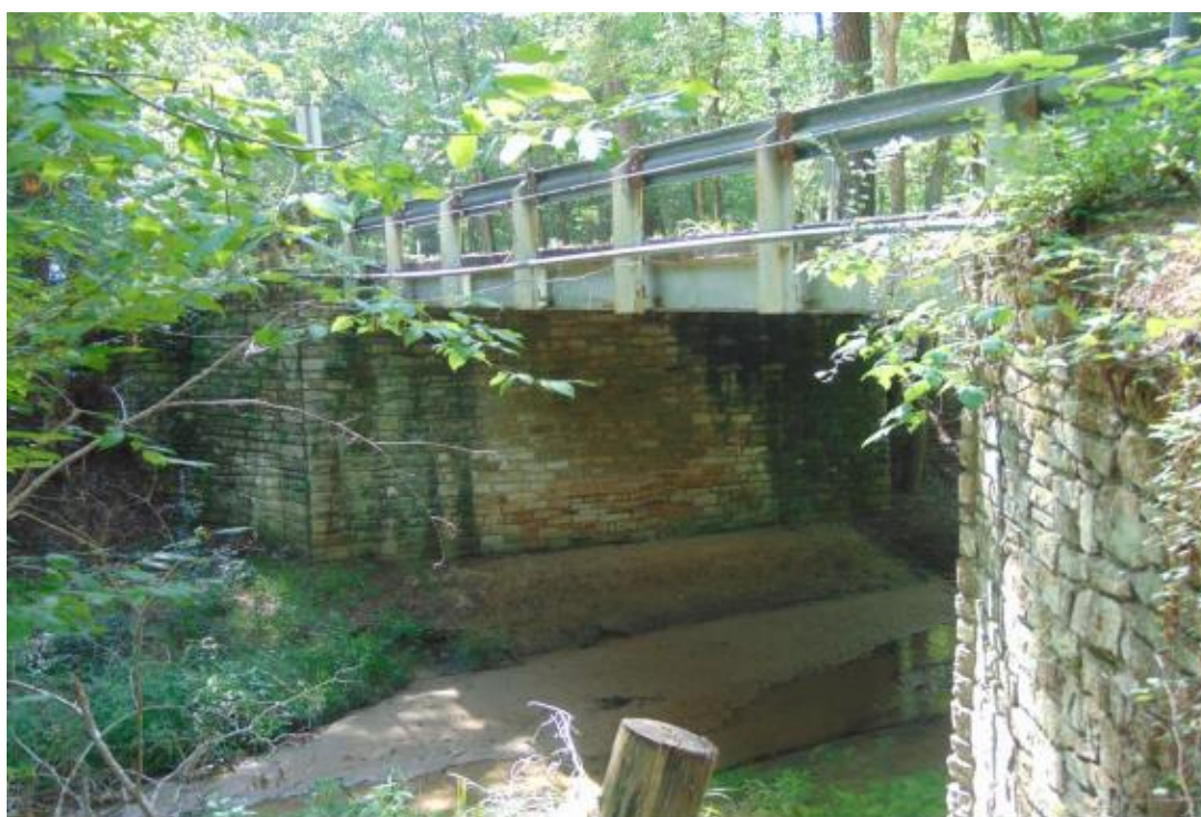
Figure B.9. Bridge SM-5 (TxDOT 2018c)
