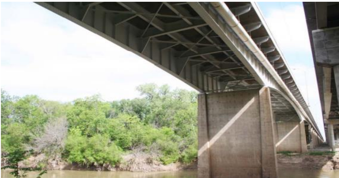
(c) Underside Superstructure View
