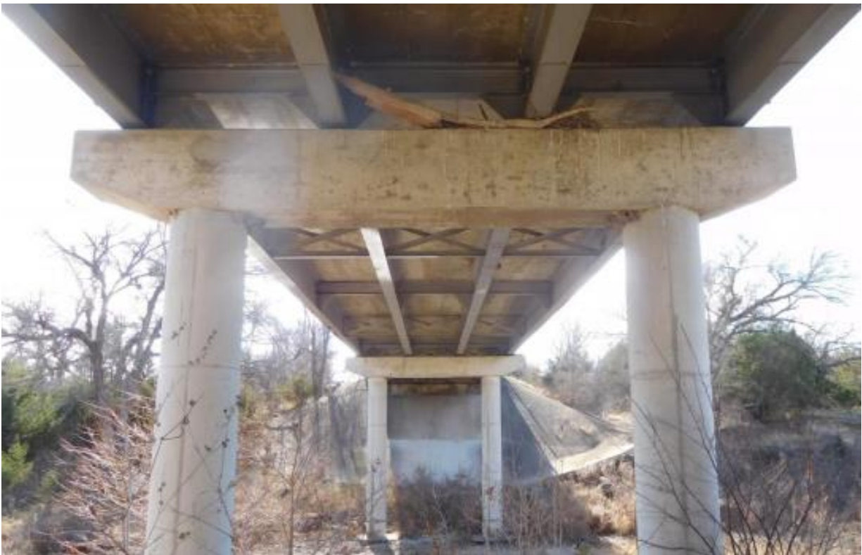
(c) Underside Superstructure View
