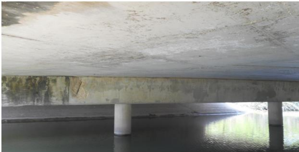
(c) Underside Superstructure View
