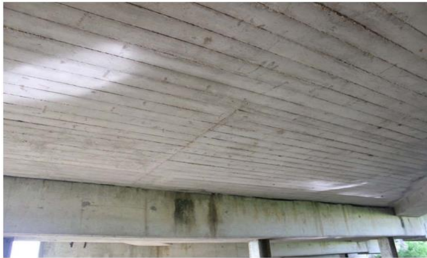
(c) Underside Superstructure View
