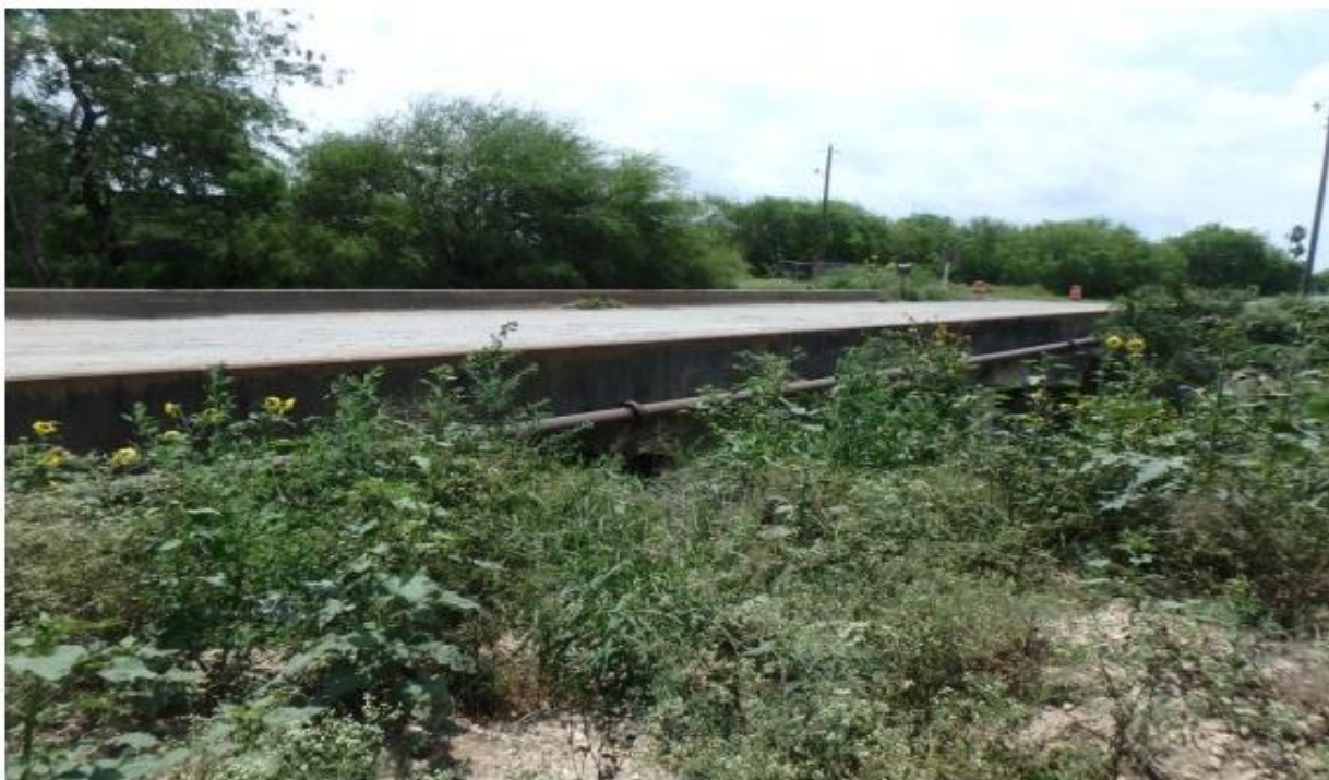
Figure C.41. Bridge CS-21 (TxDOT 2018c)
