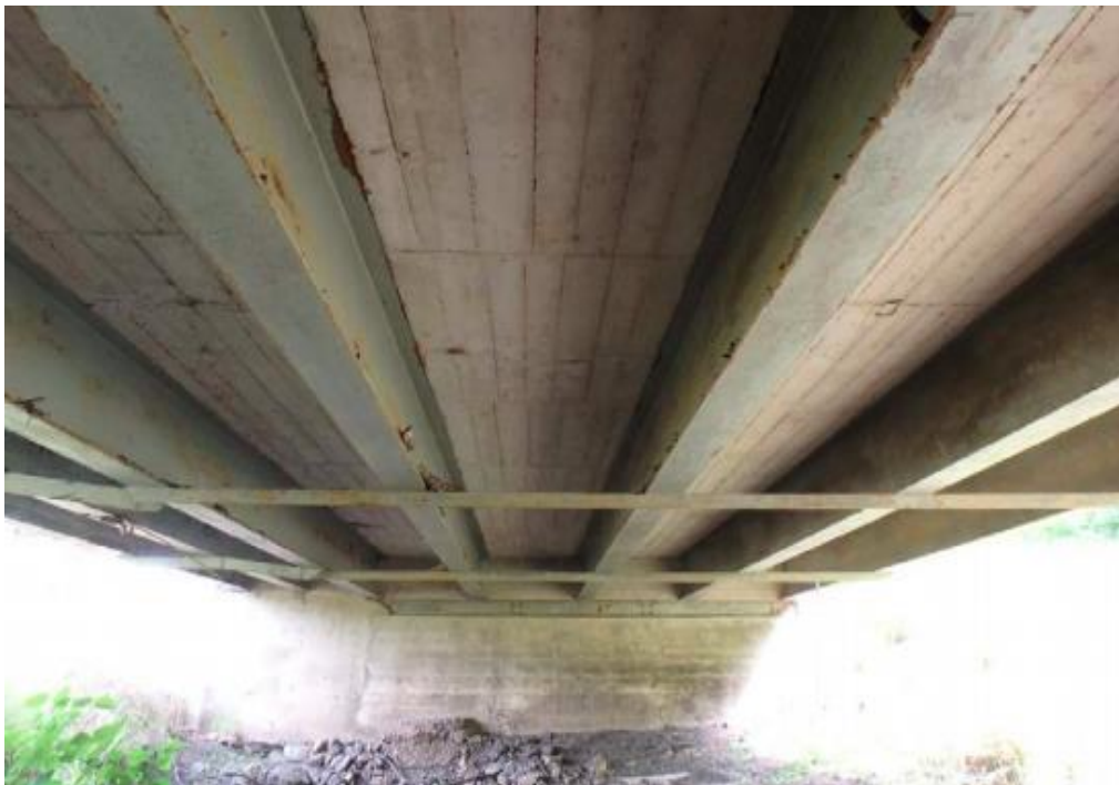
(c) Underside Superstructure View
