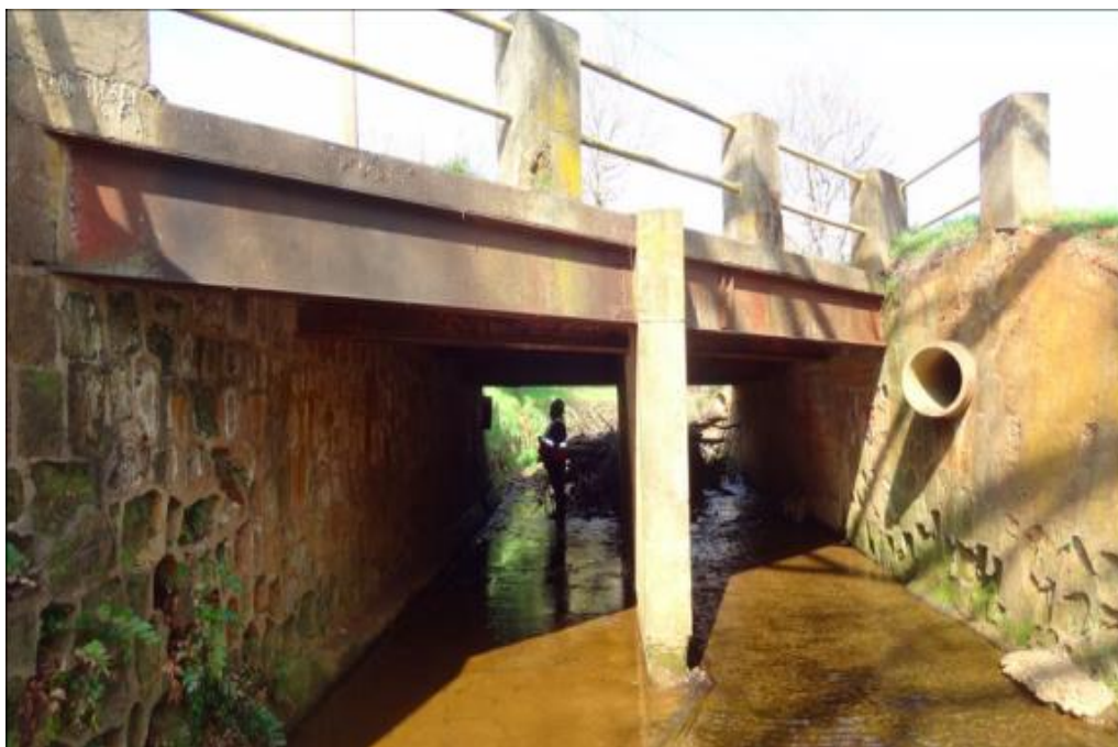
Figure B.25. Bridge SM-13 (TxDOT 2018c)
