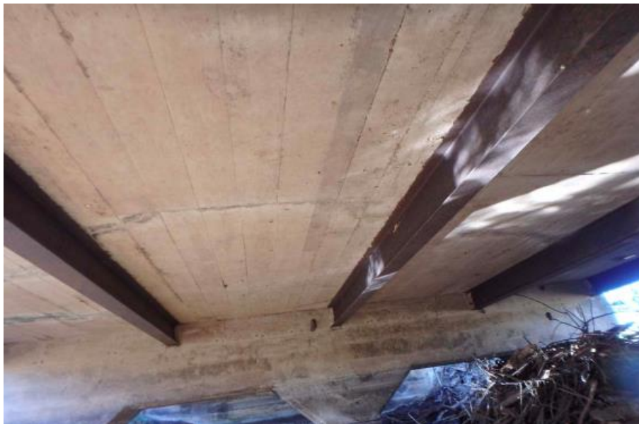
(c) Underside Superstructure View
