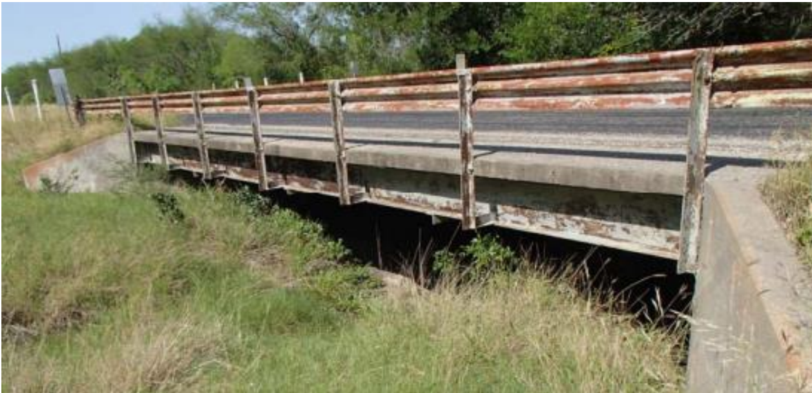
Figure B.1. Bridge SM-1 (TxDOT 2018c)
