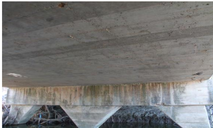
(c) Underside Superstructure View
