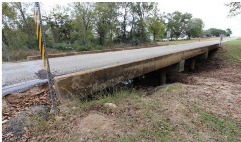
Figure C.39. Bridge CS-20 (TxDOT 2018c)
