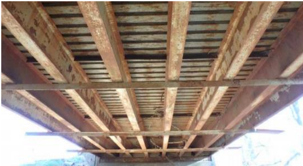
(c) Underside Superstructure View
