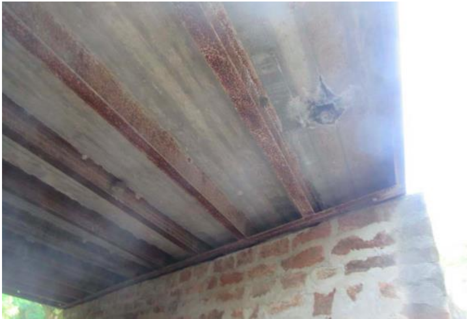
(c) Underside Superstructure View
