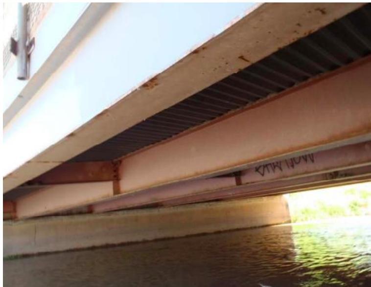
(c) Underside Superstructure View
