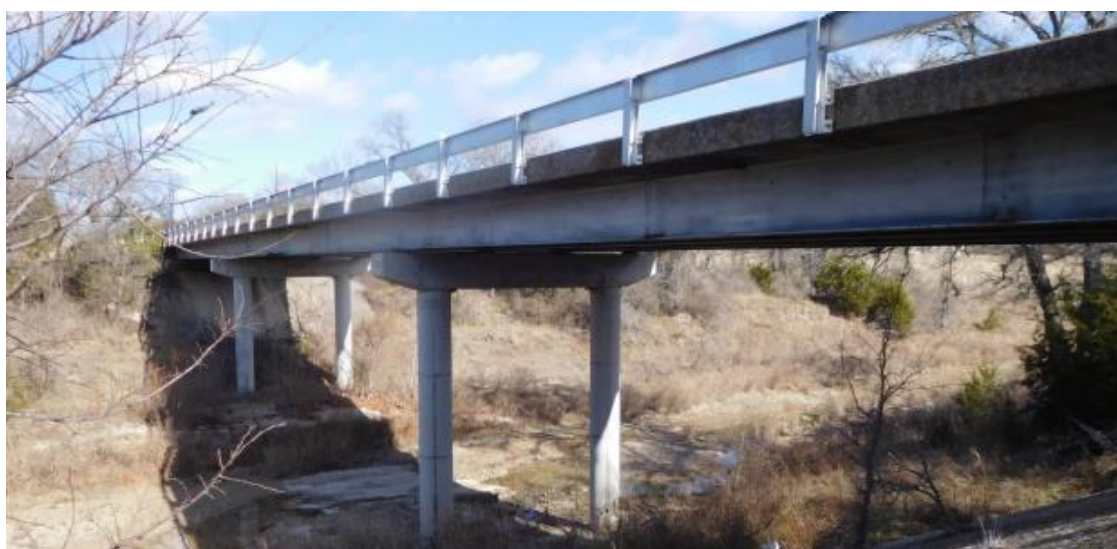
Figure B.73. Bridge SC-12 (TxDOT 2018c)
