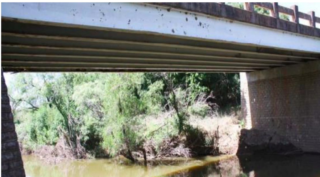
Figure B.15. Bridge SM-8 (TxDOT 2018c)
