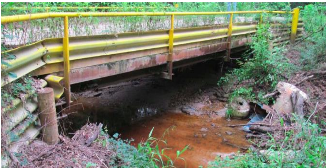
Figure B.47. Bridge SM-24 (TxDOT 2018c)
