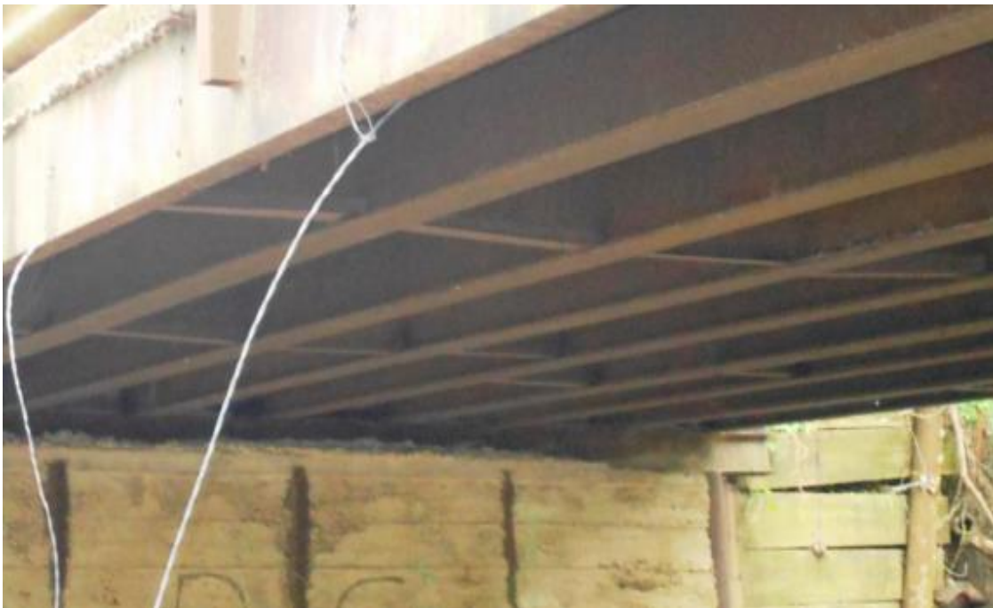
(c) Underside Superstructure View
