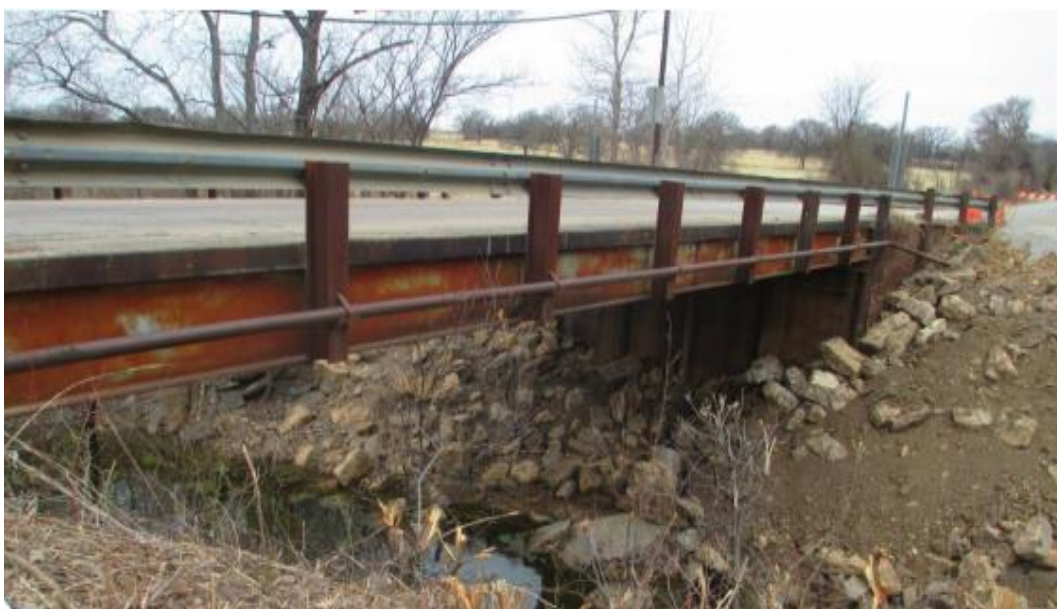
Figure B.39. Bridge SM-20 (TxDOT 2018c)
