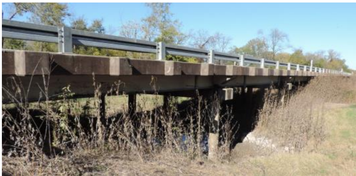
Figure B.5. Bridge SM-3 (TxDOT 2018c)
