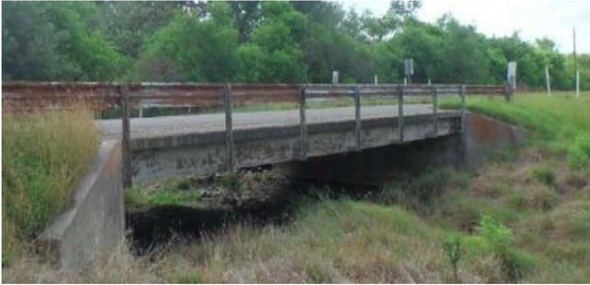
Figure B.3. Bridge SM-2 (TxDOT 2018c)
