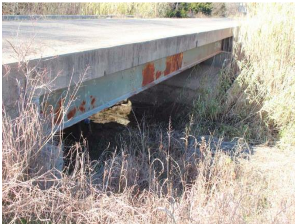
Figure B.43. Bridge SM-22 (TxDOT 2018c)
