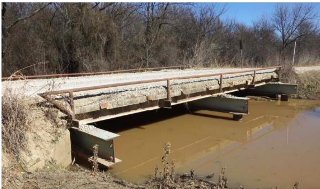
Figure B.55. Bridge SC-3 (TxDOT 2018c)
