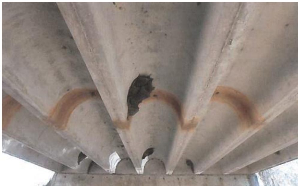
(c) Underside Superstructure View
