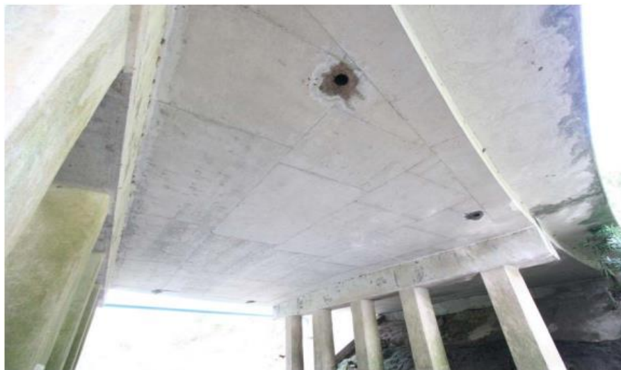
(c) Underside Superstructure View
