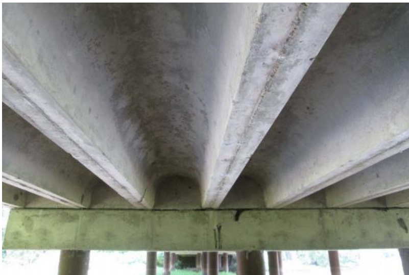
(c) Underside Superstructure View
