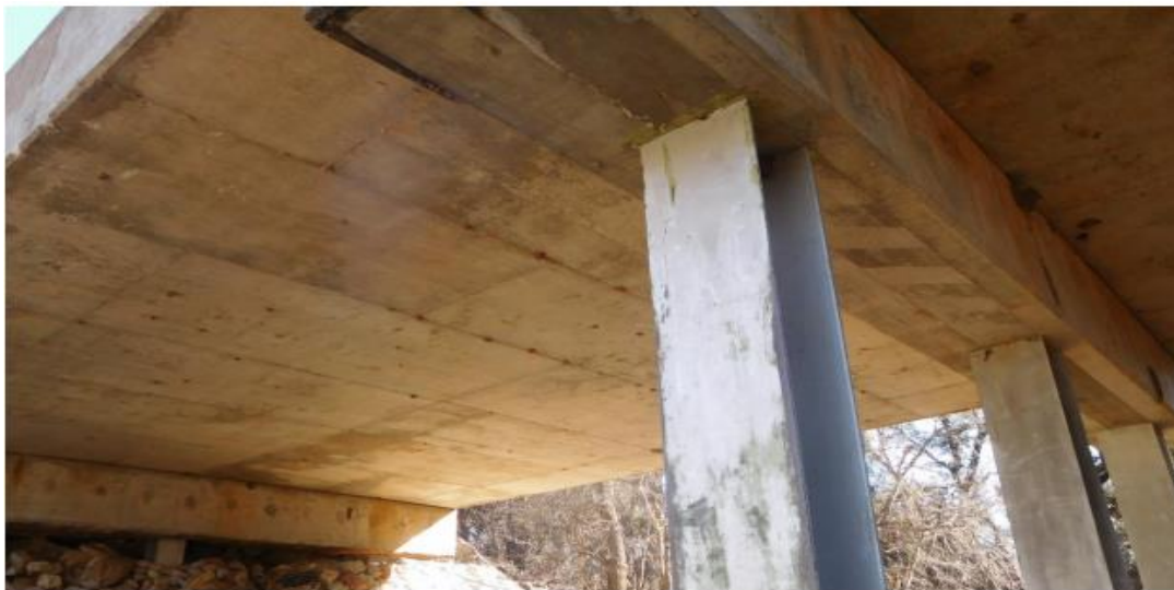
(c) Underside Superstructure View
