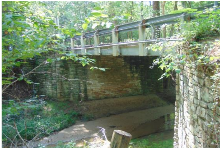
Figure 7.1. Bridge SM-5 (TxDOT 2018c)
