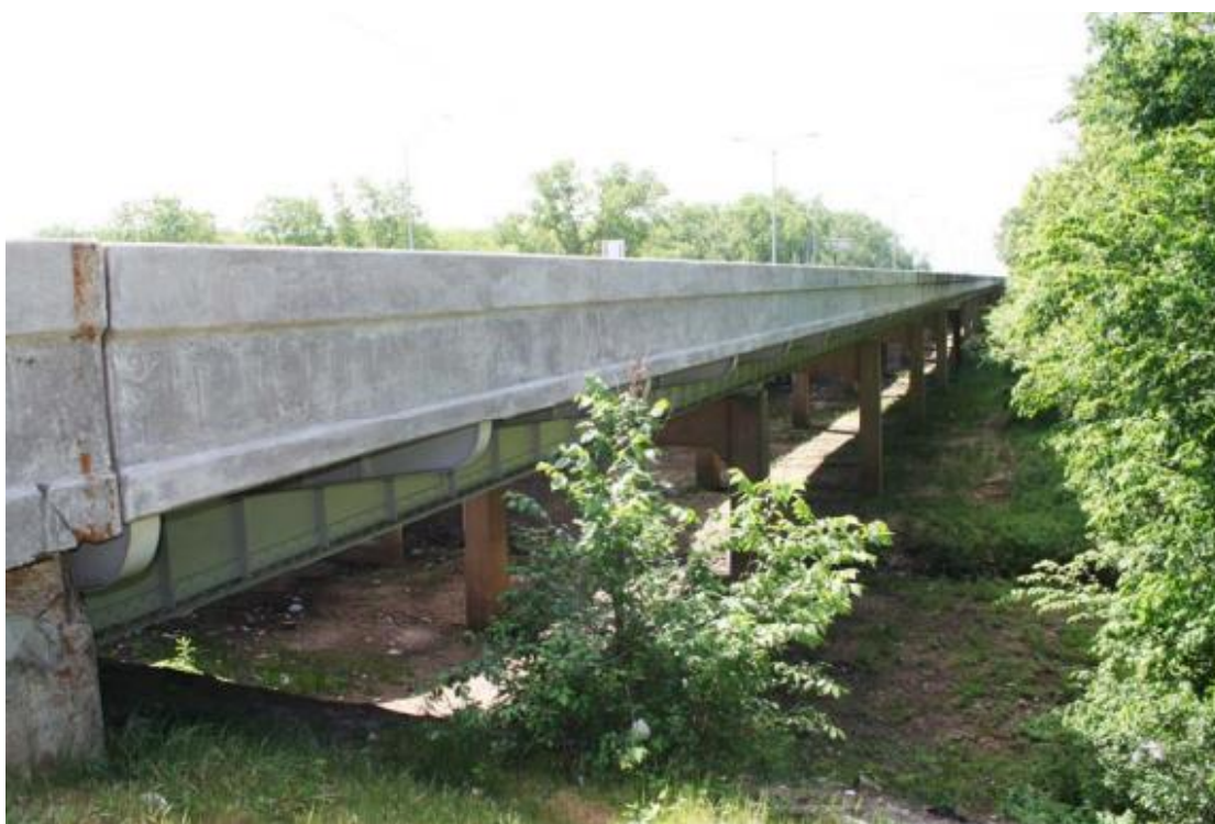
Figure B.69. Bridge SC-10 (TxDOT 2018c)
