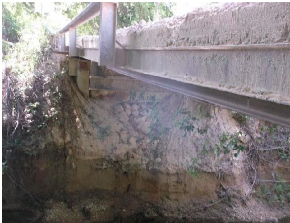
Figure B.35. Bridge SM-18 (TxDOT 2018c)
