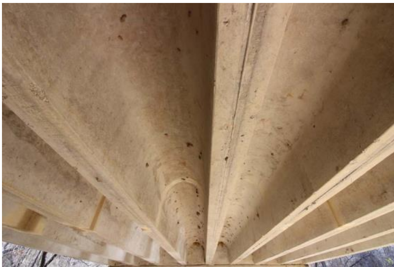
(c) Underside Superstructure View
