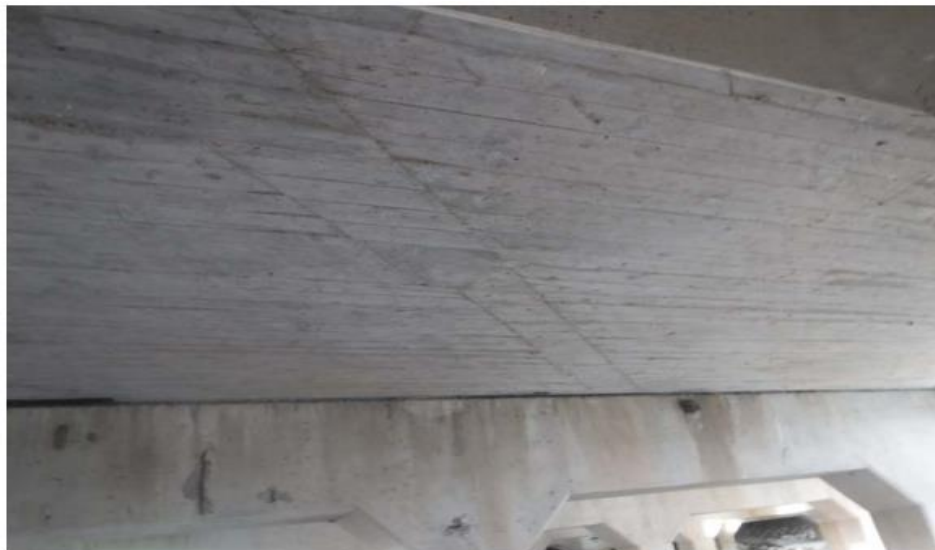
(c) Underside Superstructure View
