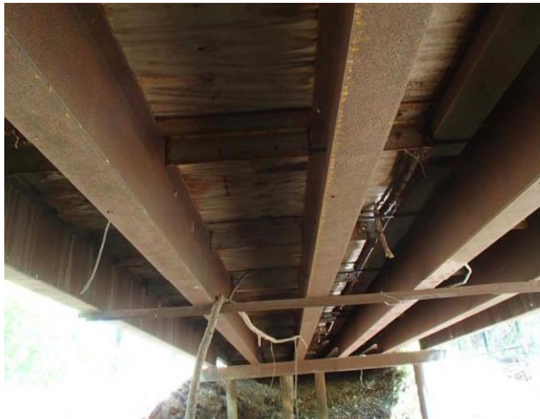
(c) Underside Superstructure View
