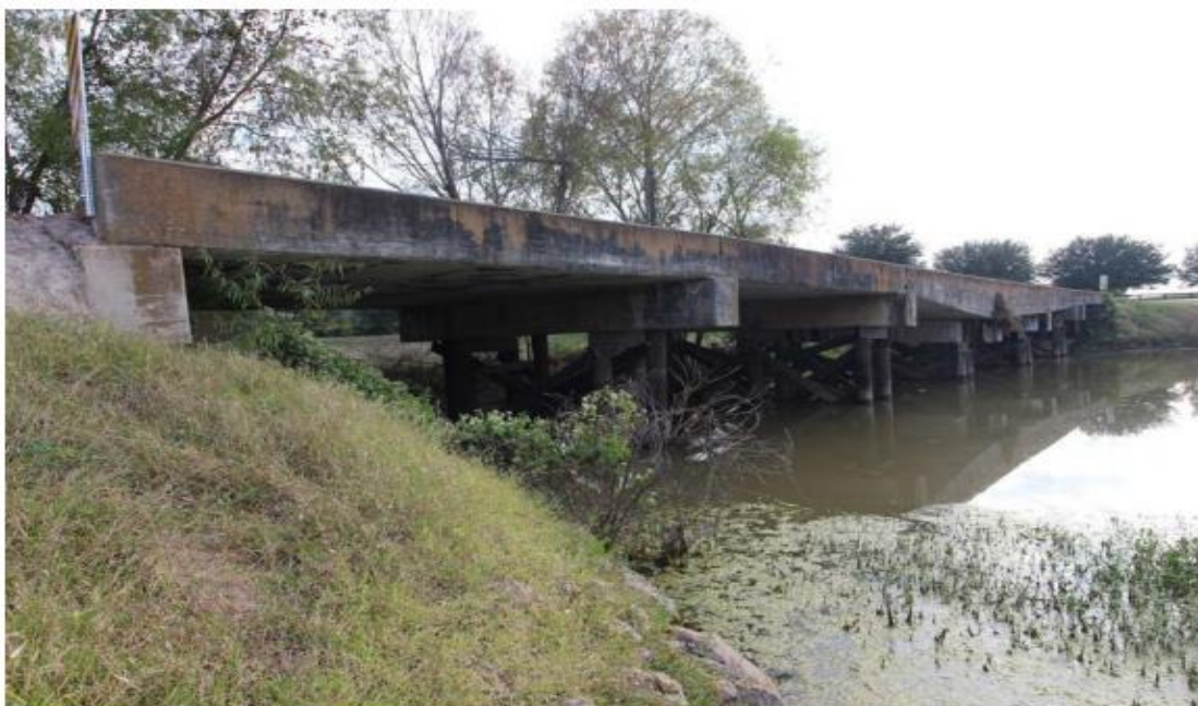
Figure C.13. Bridge CS-7 (TxDOT 2018c)
