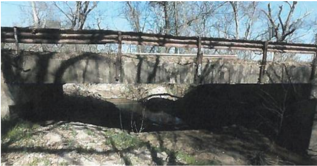
Figure 7.7. Bridge CM-5 (TxDOT 2018c)
