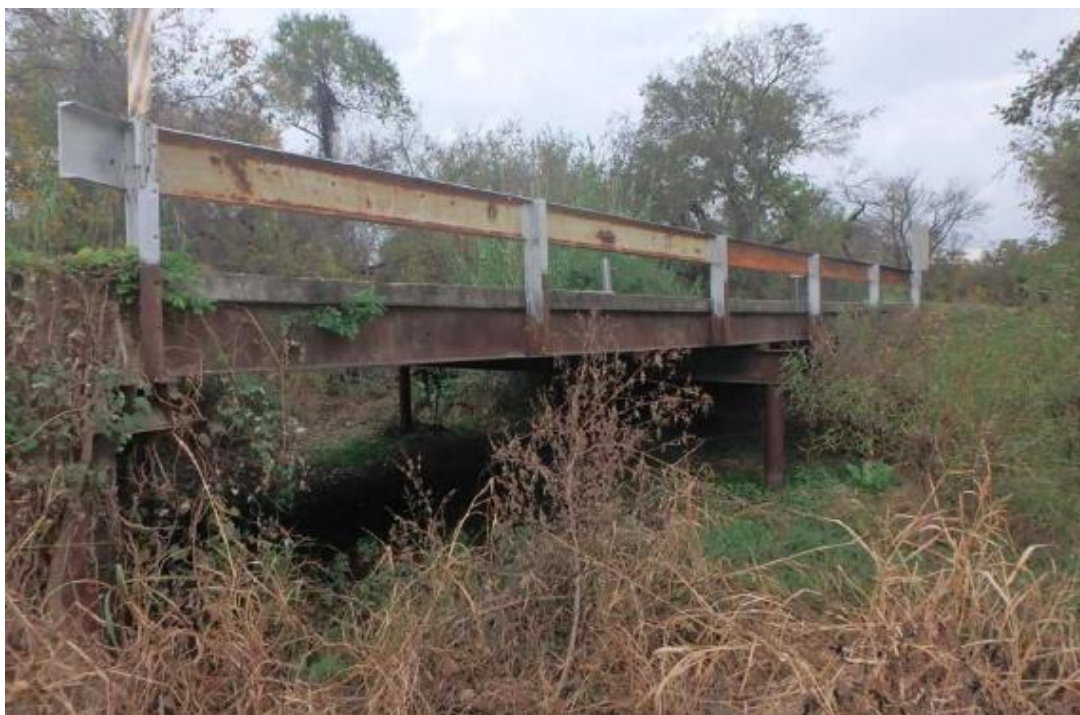
Figure B.61. Bridge SC-6 (TxDOT 2018c)
