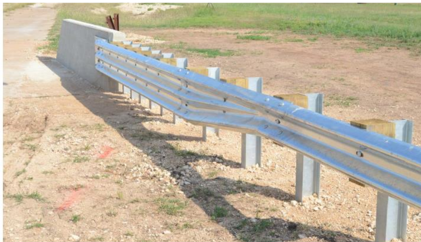
Figure 2.8. Thrie Beam Transition without Curb.
