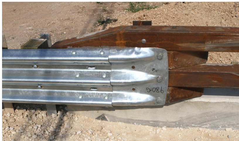
Figure 2.10. T131RC Bridge Rail Transition Connection.
