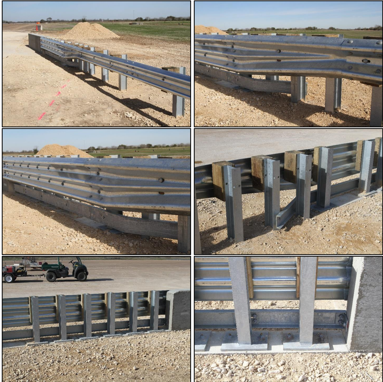
Figure 7.2. Upstream Transition prior to Testing.
