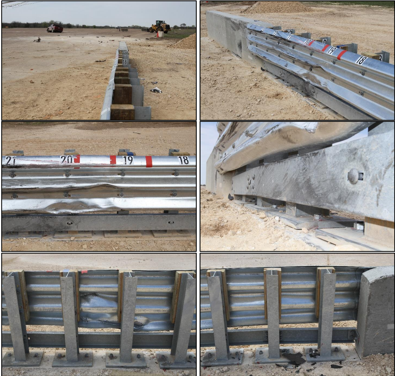
Figure 8.3. Downstream Transition after Test No. 469549-01-4.
