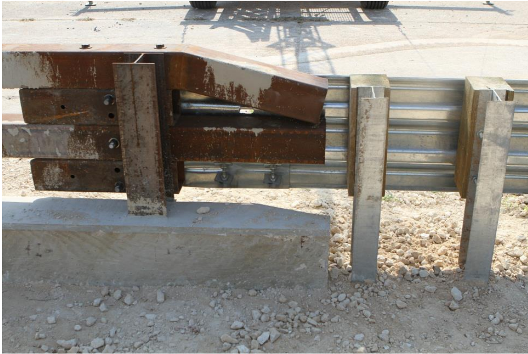
Figure 2.11. T131RC Bridge Rail Transition Connection Field View.
