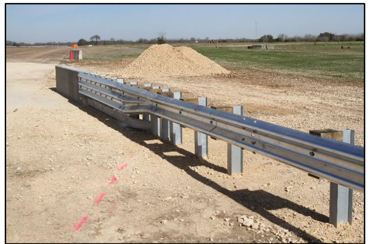
Figure 1. Guardrail to Rigid Barrier Transition.
