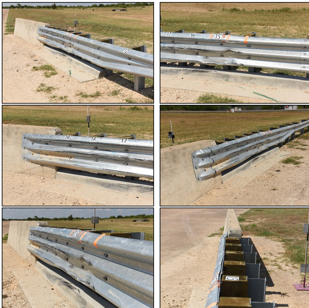
Figure 6.5. Thrie-Beam Transition without End Shoe Block after Test No. 469469-5.
