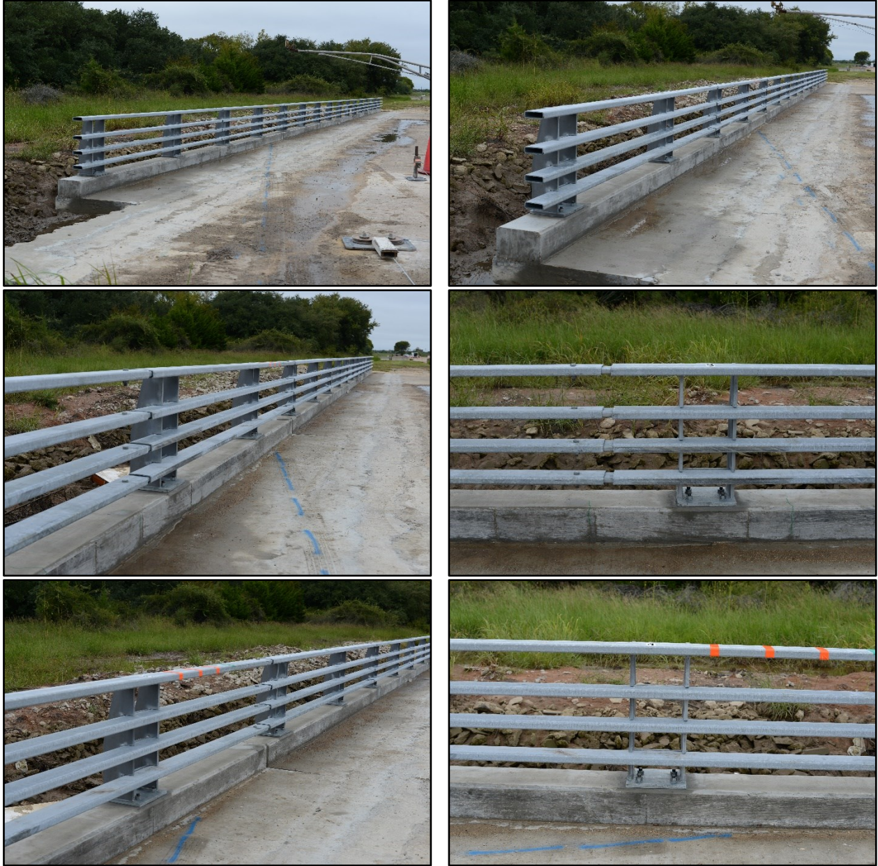
Figure 2.2. C1W Bridge Rail prior to Testing.
