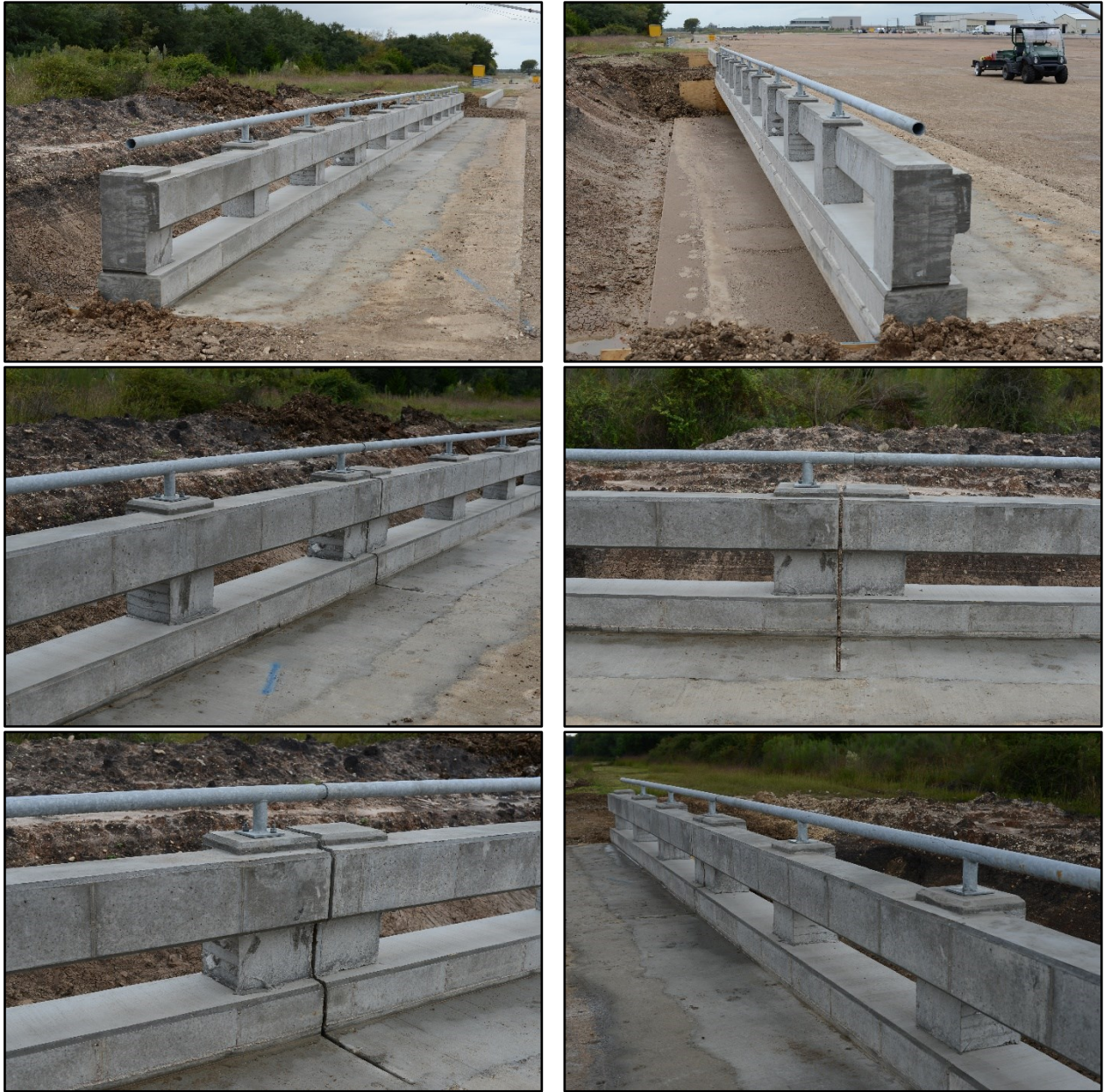
Figure 3.2. Modified C66 Bridge Rail prior to Testing.
