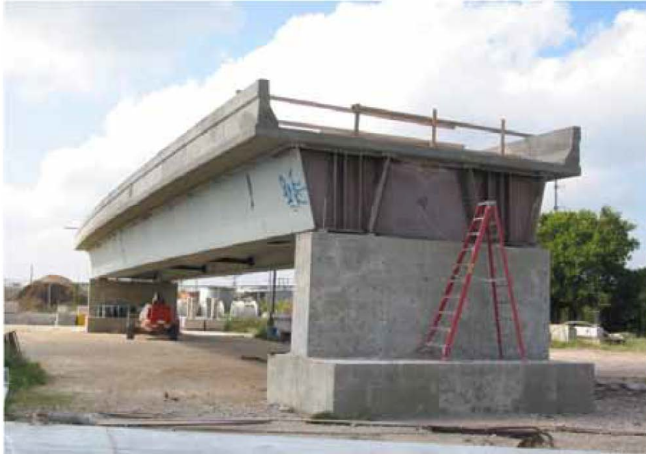
Figure 3.1. The FSEL Test Bridge (Barnard et al. 2010).
