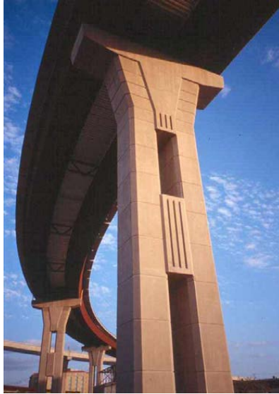
Figure 2.4. STTG Bridge, I-35/US 290 Interchange, Austin, Texas (Coletti et al. 2005).
