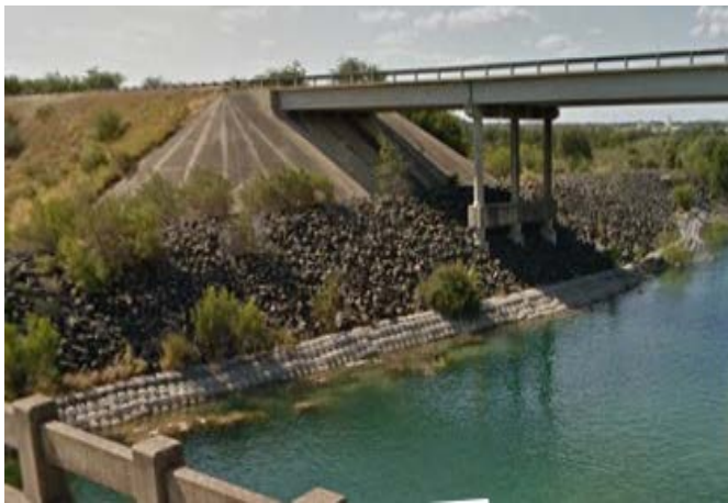
Figure 30. Right Abutment Repair at US 90 over Nueces River.
