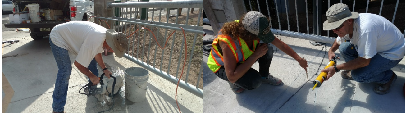
Figure 17. Example of Saw Cutting and Sealing Loops.
