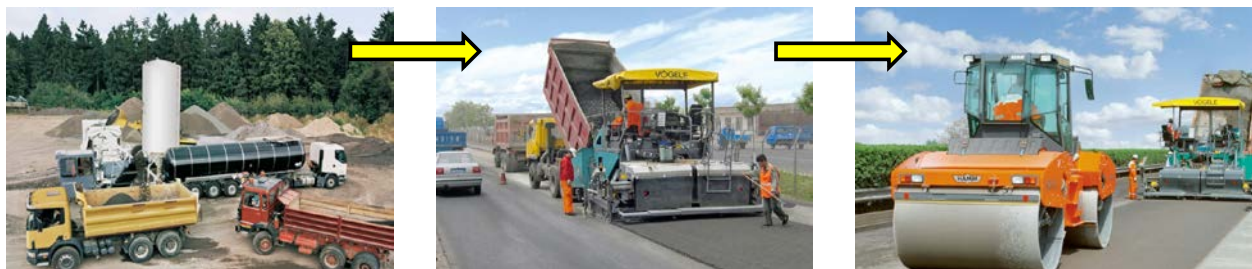
Figure 3. Typical CCPR Construction Steps.
