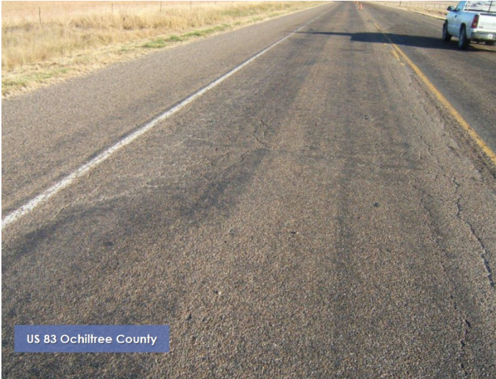
(a) Condition before CIR construction
