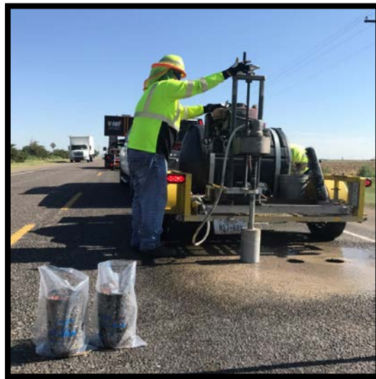
Figure 19. FWD and Coring of existing CIR Section.
