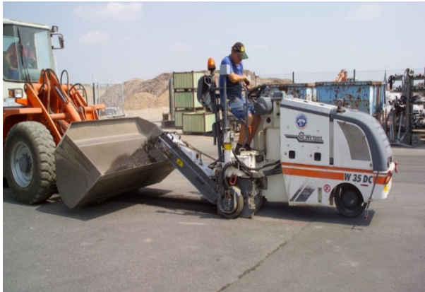
(a) Wirtgen small milling machine
